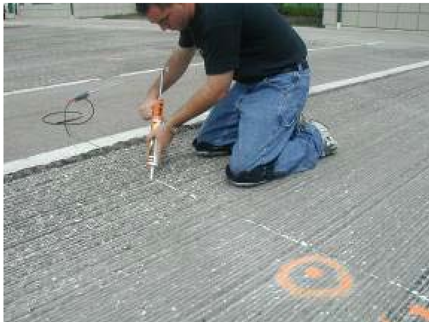
FIGURE 6 Sealing gauge wire path with silicone sealant.
