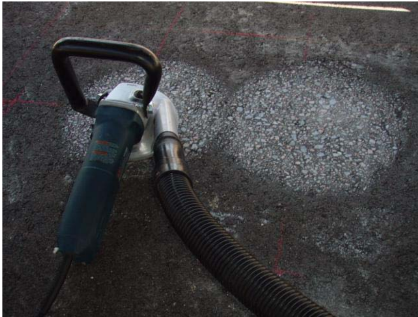
FIGURE 9 Grinding the HMA surface.
