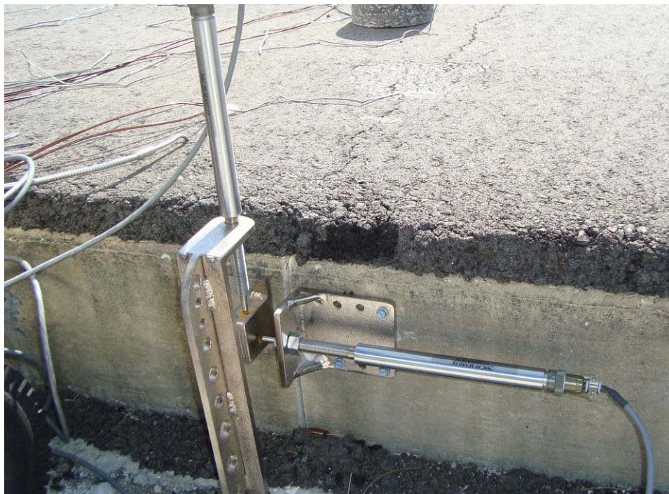
FIGURE 25 Measurement of concrete joint movement with LVDTs.
