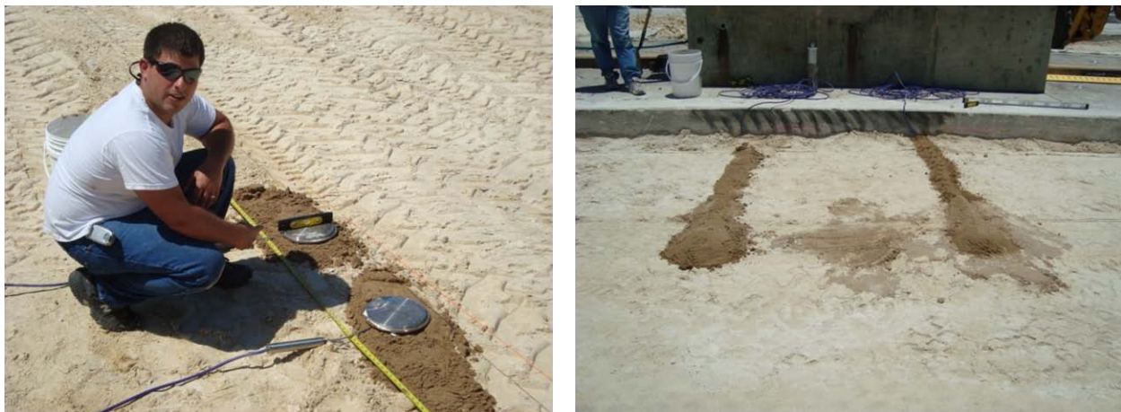
FIGURE 16 Placing and leveling pressure cells.
