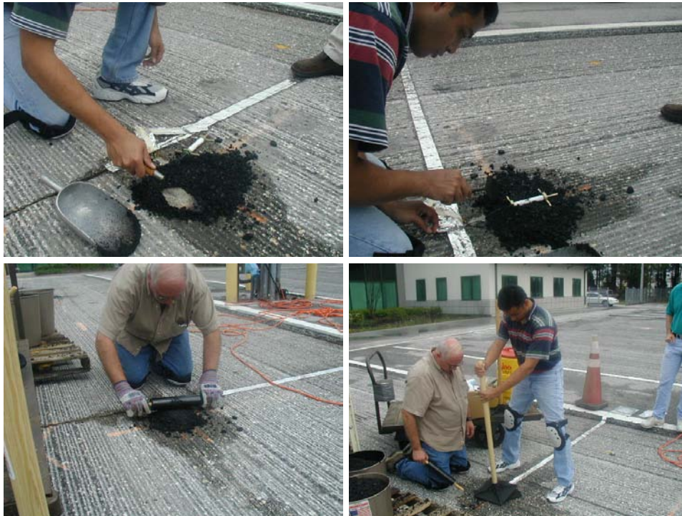
FIGURE 7 Placement of gauges prior to paving.
