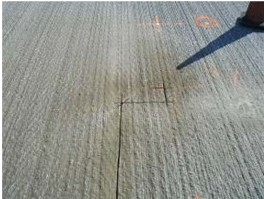
FIGURE 4 Saw-cut for strain-gauge wire.
