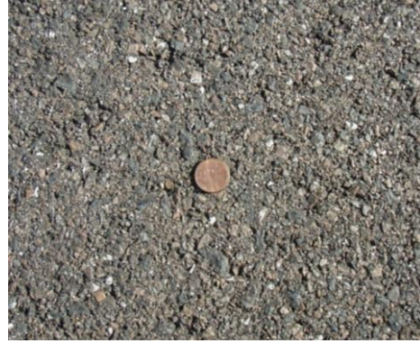
(b) Non-segregated area
