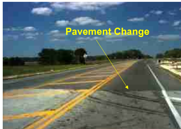
Figure 11. Example of Logged Pavement Change
