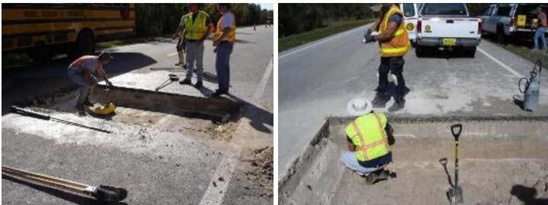
Figure 11. Nuclear density tests and layer thickness measurements in trench
