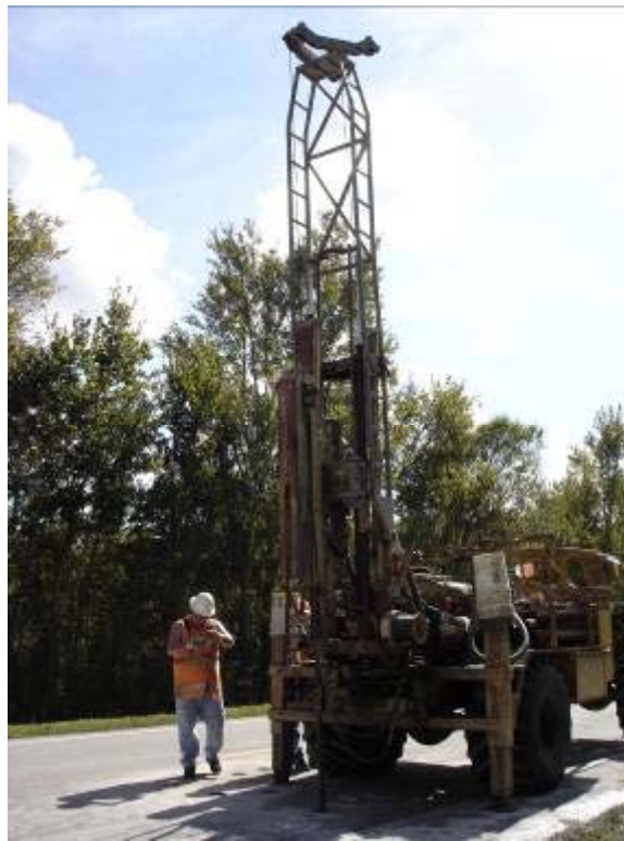
Figure 17. Standard penetration test using a split-spoon sample
