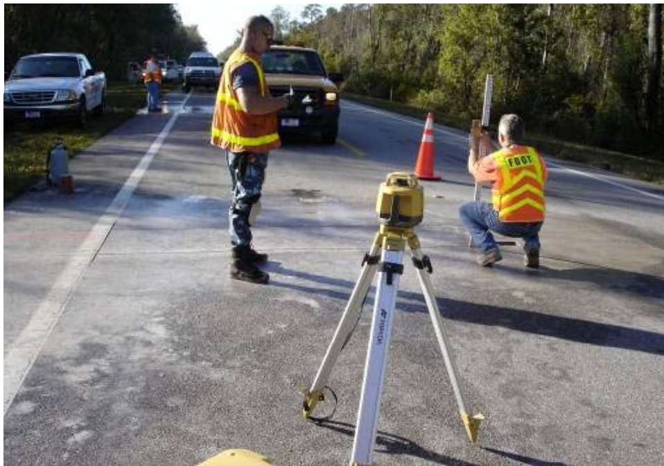
Figure 9. Measuring surface profile with laser level
