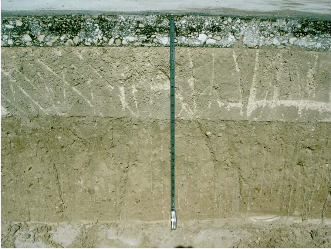
Figure 12. Photograph of a typical trench cross-section
