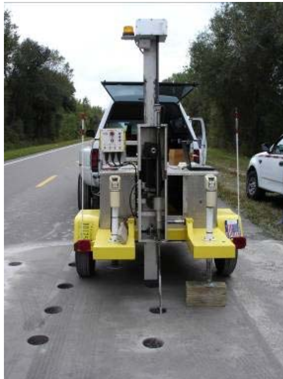
Figure 18. DCP test through core hole
