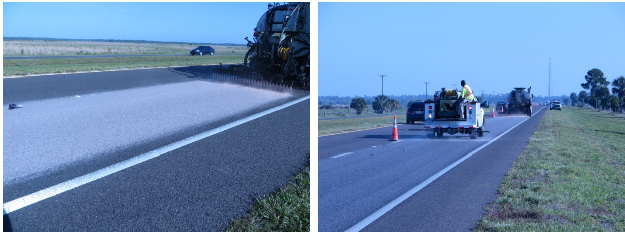
FIGURE 6. Application for Reclamite
