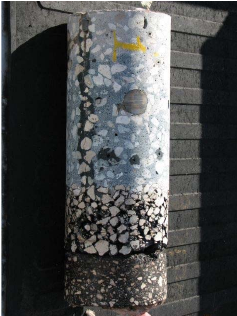
Figure 5 – Core Exhibiting No Distress; I-95 Rest Area - Martin County
