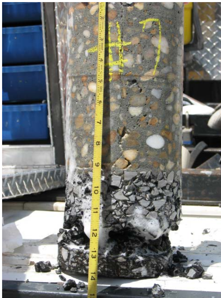
Figure 2 – Core Exhibiting Moisture Damage; I-10 Weigh Station - Jackson County
