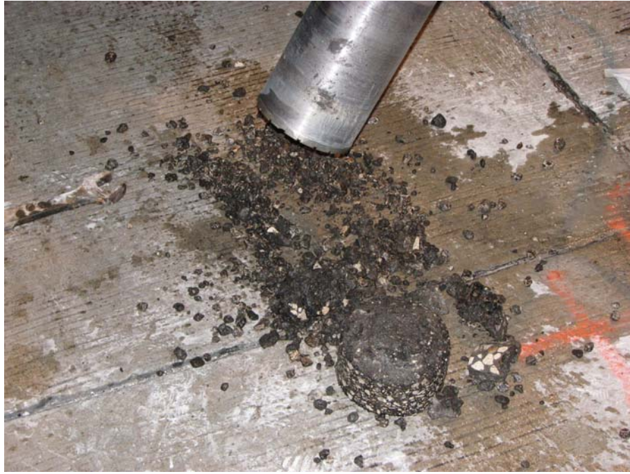
Figure 7 – Core Exhibiting Moisture Damage; SR-60 and North 22nd Street - Hillsborough County
