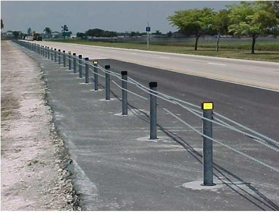
BRIFEN USA Post installed in a reinforced Ring set in concrete foundation. 4 cables are placed as follows: #1 in a slot on the top of post, #2 thru 4 are interwoven between all posts on pegs located on the sides of each post. The first 15 posts adjacent to the end terminal do not have top cable / rope slot. The top cable weaves on either side of posts until the first line post with a slot.
