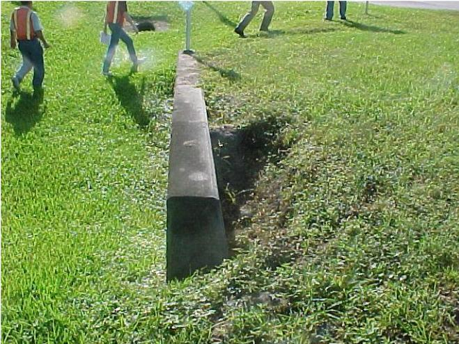
This is a washout in front of a headwall greater than 6 inches in depth. This would not meet MRP standards.
