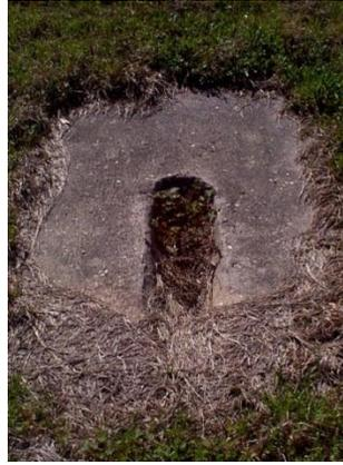
These pictures are of edge drains. The edge drain hardware cloth must be in place and functioning as intended to meet MRP standards. These edge drains do not meet MRP standards.
