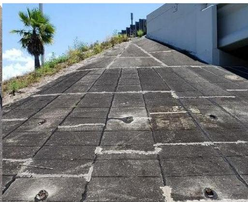
Some of these weep holes have vegetation growing out of them. If more than 10% are filled on one side of sample point, this would not meet maintenance conditions.
