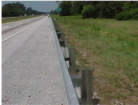
For MRP purpose, evaluate asphalt from edge of travel lane to face of guardrail as paved shoulder.
