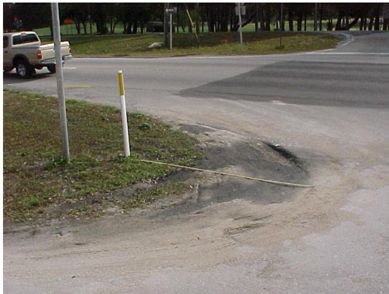
This is a rural crossover with a post mounted delineator installed. According to Standard Plans the delineator should be installed 6 ft. from the edge of pavement to the delineator. MRP has a tolerance of 1 ft. 6 inches. This delineator is installed 8 ft. 6 inches from the edge of pavement. This installation does not meet MRP standards.
