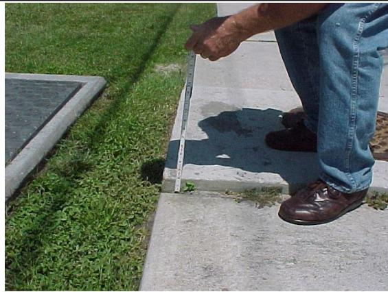
Sidewalk cracking. Measure each horizontal crack greater than  $\frac{1}{2}$  inch wide. For MRP purposes, each linear foot of horizontal crack greater than  $\frac{1}{2}$  inch equals 1 sq. ft. of crack area.
