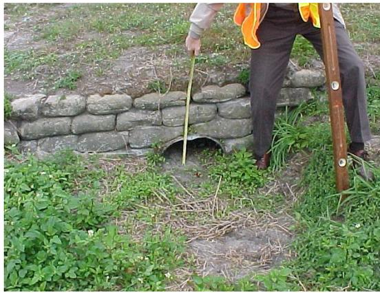
These two pictures show a typical side drain pipe in a roadside ditch. Determine the cross section of the pipe that is not obstructed and functions as intended. If more than 40% of the pipe cross section is obstructed or does not function as intended, then CROSS/SIDE DRAIN does not meet desired maintenance conditions.
