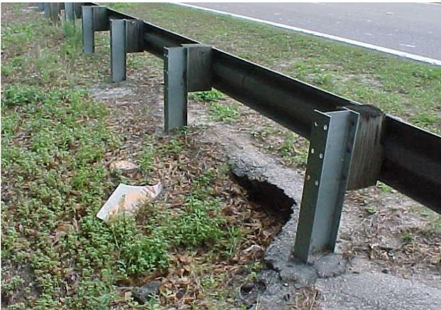
The asphalt under the guardrail has washed out. The guardrail meets desired maintenance conditions, however, unpaved shoulder or front slope would not meet MRP standards.
