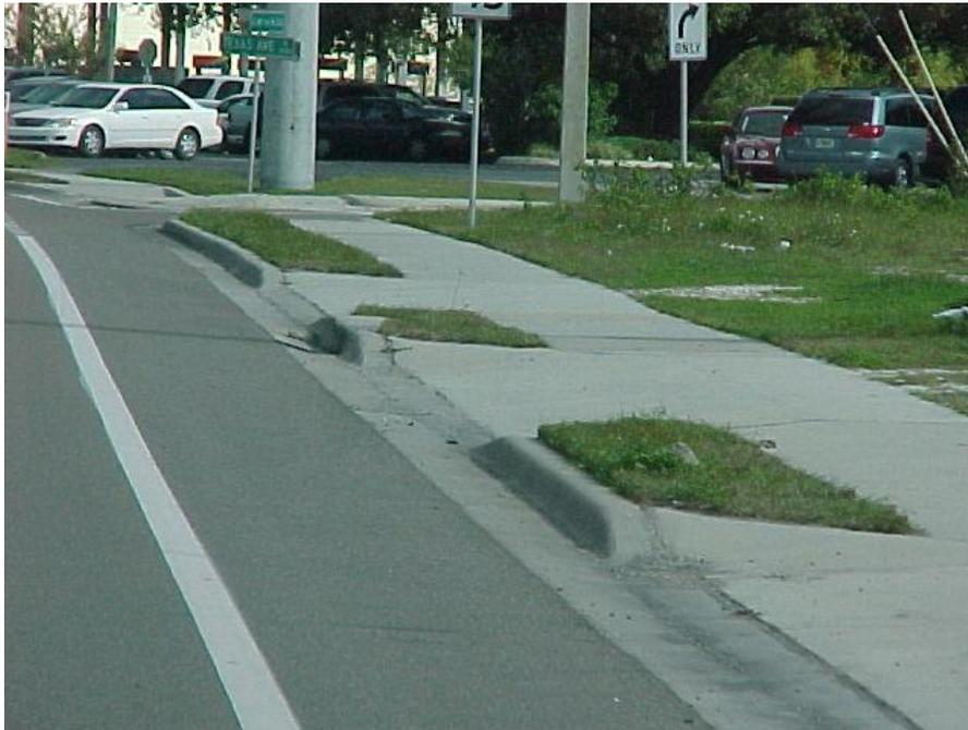
These are urban flared turnouts. The area from the back of curb to the front of the sidewalk is to be rated as turnout.
