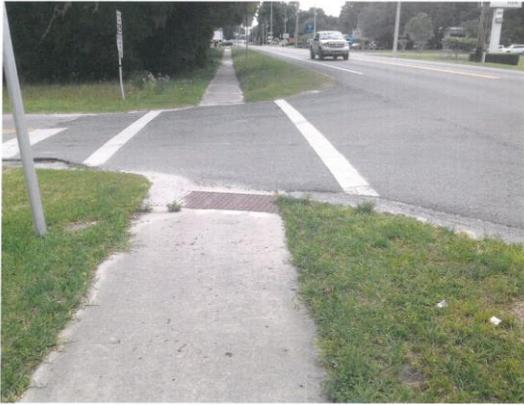
Material accumulation exceeds 3/4 inch deep at marked pedestrian crossings and would not meet MRP standards.
