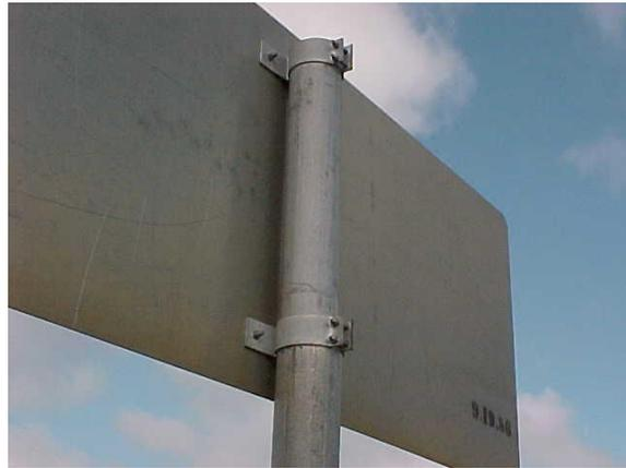
This sign was installed using "C clamps and does not meet MRP standards.
