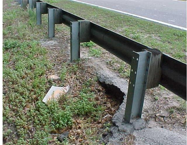
The asphalt under the guardrail has washed out. The guardrail meets desired MRP standards, however, unpaved shoulder or front slope would not meet desired MRP standards.
