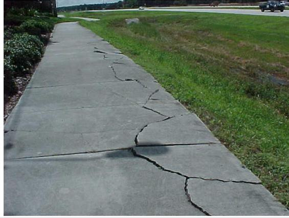
Sidewalk cracking. Measure each horizontal crack greater than  $\frac{1}{2}$  inch wide. For MRP purposes, each linear foot of horizontal crack greater than  $\frac{1}{2}$  inch equals 1 sq. ft. of crack area. Vertical misalignments greater than 1/4 inch equals 1 sq. ft. of crack area.
