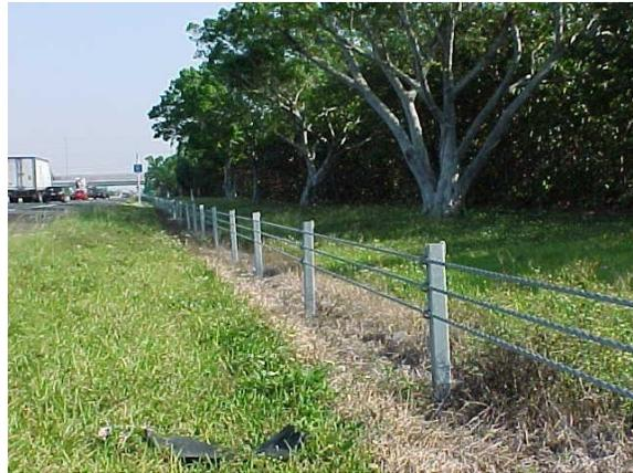
GIBRALTAR Post installation similar to the CASS and SAFENCE. 3 cables are placed in molded "hairpin" slots or J bolts installed along the sides of the posts.
