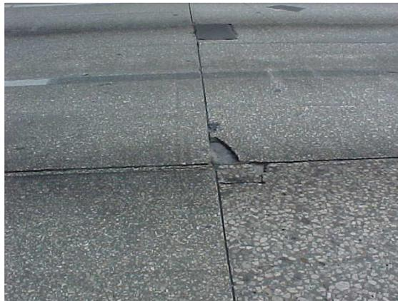
These are pictures of defects in rigid pavement. Calculate the area to determine if it is greater than 1/2 square foot and measure the depth of the defect. If BOTH depth and area are greater than the standard limits the areas do not meet MRP standards.
