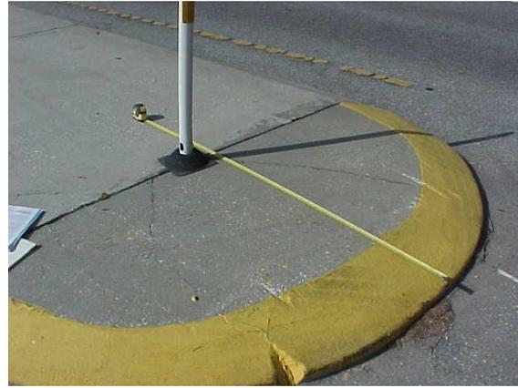
Post mounted delineators are installed according to the Standard Plans. The index shows the edge of pavement as the standard reference point. If curb and gutter is present measure from the top face of curb. At a curb without a gutter or traffic separator, the face is the edge of pavement (picture on right).
