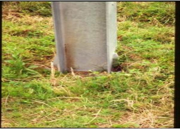
This breakaway device is covered and does not meet MRP standards.
