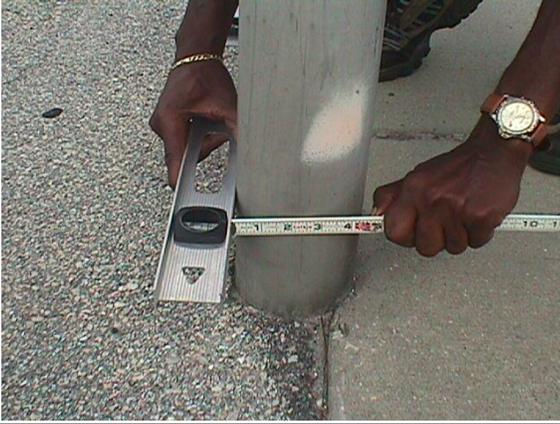
Measuring a sign post. This post is 4 inches and should be installed with a concrete foundation and breakaway assembly. This sign installation does not meet MRP standards.
