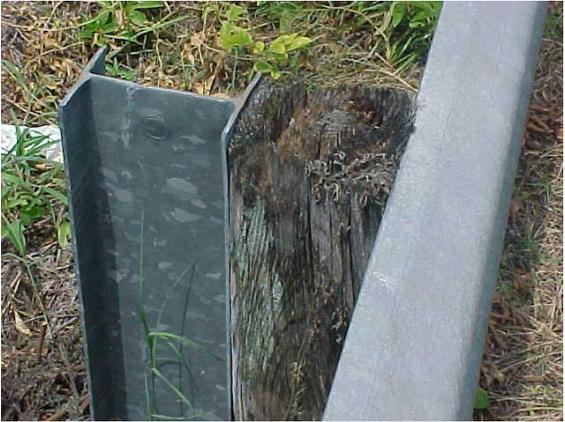
This is a rotten and deteriorated guardrail offset block. It does not meet MRP standards if more than 10% of the blocks are rotten and deteriorated.
