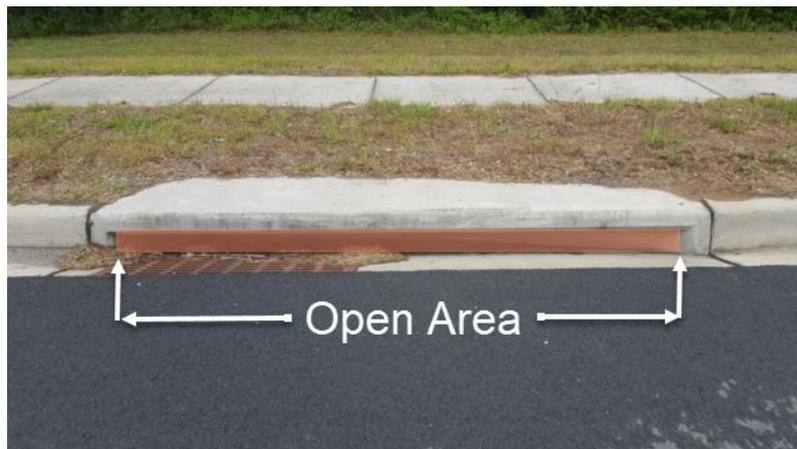
Measure the opening to determine the area. 85% of the opening area must be unobstructed to meet the inlet characteristic.
