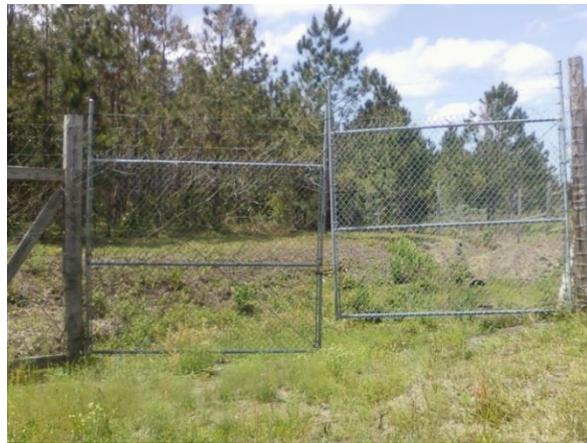
Misaligned gates, measure opening to ensure it is not greater than 6 inches.
