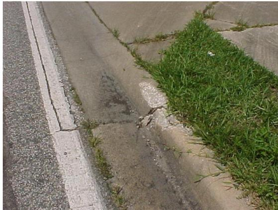
This type 'F' curb has been damaged. Type 'F' curb is not rated in MRP.
