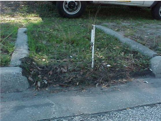
Soil buildup in a miscellaneous drainage structure. This does not meet MRP standards for miscellaneous drainage.
