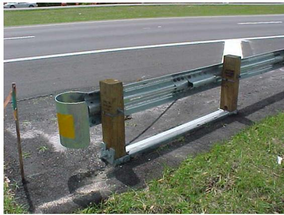
This is an approach end guardrail end section. Check to make sure all connecting hardware is in place.
