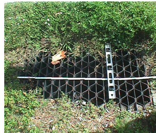
This is an obstructed inlet grate. If the Opening is obstructed more than 85%, then it would not meet MRP standard for inlets.
