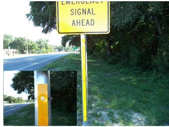
This Retroreflective panel is the correct color and has been mounted to the post correctly. This would meet maintenance conditions.
