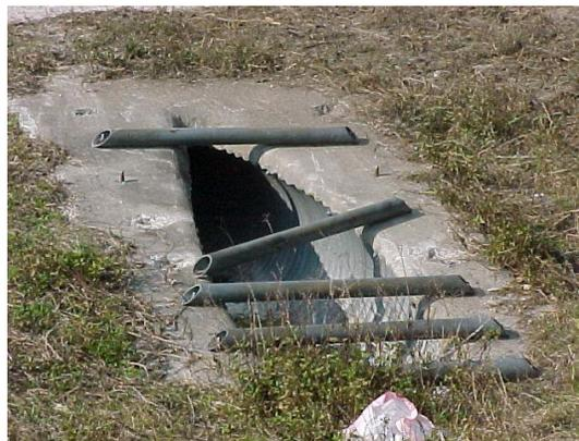
This is a side drain pipe with missing and damaged grates. This does not meet MRP standards.
