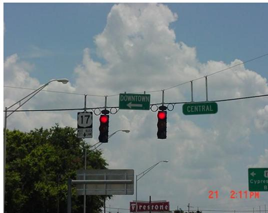
Do not rate county/city signs on signal cables. The US 17 route marker would be rated as a sign >30 sq.ft. because it is an over-lane sign.
