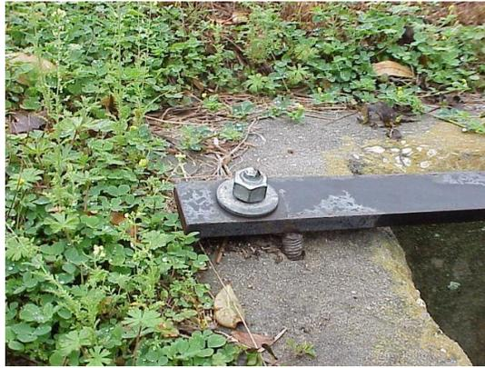
Repaired grate. Epoxy bolt. Meets conditions.
