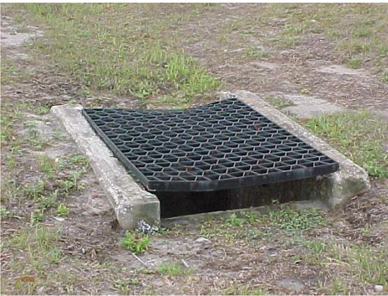
This inlet grate is not seated correctly in the design cradle. This does not meet MRP
