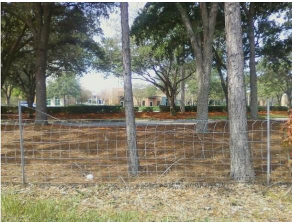
Both strands of barb wire are missing along top of fence, this would not meet desired maintenance conditions.
