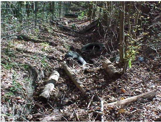
If the ditch bottom elevation of an outfall ditch is more than  $\frac{1}{3}$  of the difference between natural ground and the design flow line the outfall ditch does not meet MRP standards.
