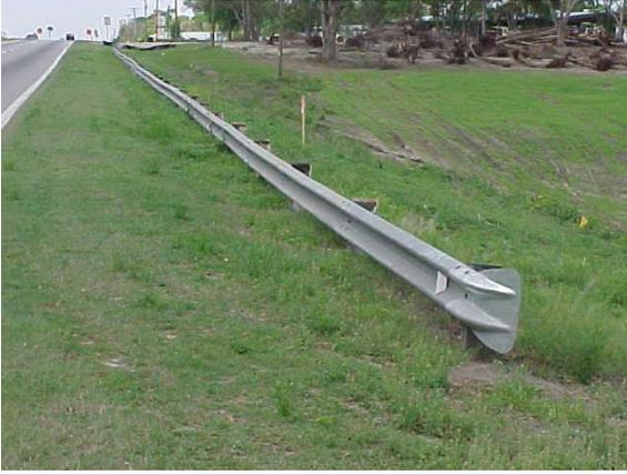
This guardrail section is low and should be measured to determine if it meets MRP standards.
