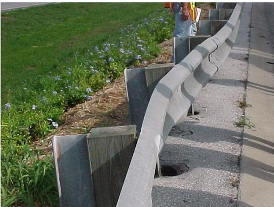
This guardrail has been hit by a vehicle. The posts have been knocked out of alignment and may not function as designed. This guardrail does not meet MRP standards.
