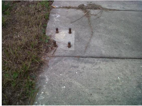
Rigid objects protruding from concrete greater than  $\frac{1}{4}$  inch in height.
