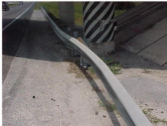
This guardrail has been hit and several posts are missing. This guardrail does not meet MRP standards.
