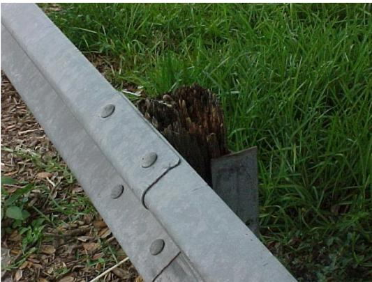
This guardrail section has several problems. The offset block is deteriorated and the rail is lapped incorrectly. This does not meet MRP standards.
