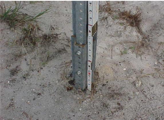
This steel flanged channel post is installed greater than 4 inches above the ground and is a non-standard installation does not meet MRP standards.
