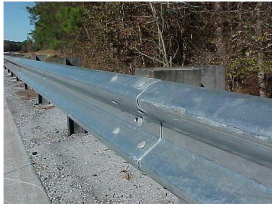
This guardrail section is lapped incorrectly. If hit by a vehicle, the rail would not function as designed. This does not meet MRP standards.
