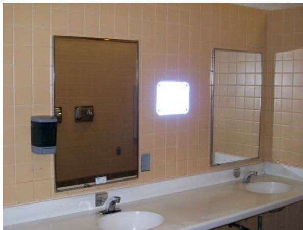
This countertop appears to meet conditions.
