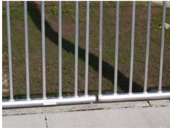
Picket railing missing steel sleeve at expansion joint. This does not meet desired maintenance conditions.
