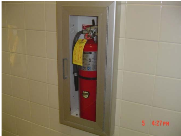
Extinguisher in proper cabinet with inspection sticker available.
