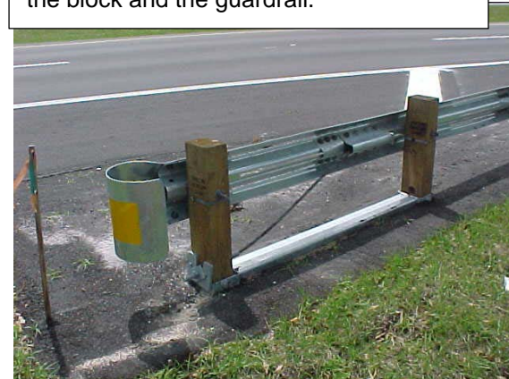
End anchorage cable is not drawn taut; check for more than 1 inch deflection
