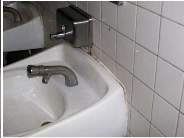
This faucet has some staining or discoloring but would meet conditions. The caulking would not meet desired maintenance conditions.
