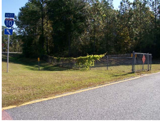
Example of Vegetation on fence and would not meet desired maintenance conditions.
