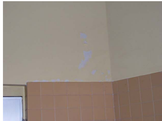
Example of peeling paint on wall.
