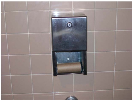
This dispenser is out of paper and would not meet desired maintenance conditions.
