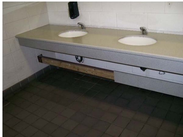
This countertop is missing a trim rail and would not desired meet conditions.
