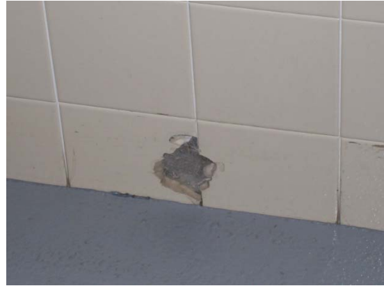
Example of broken tile on wall.
