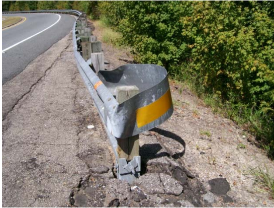
Damaged end section, this would not meet desired maintenance conditions.
