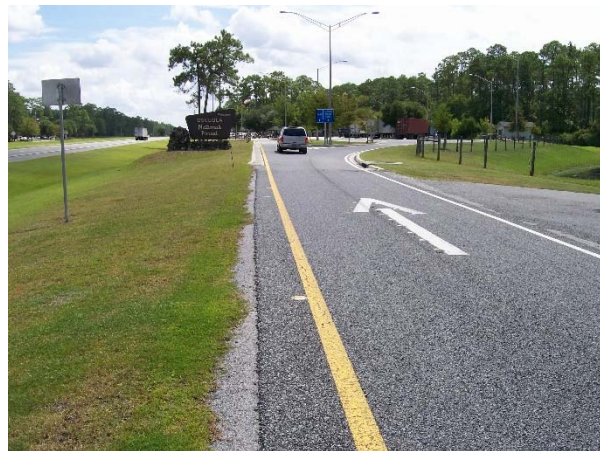
Example of symbol on roadway / ramp areas with raised pavement markers as part of the symbol measure total area of symbol also count total number of markers. Calculate if more than 30% do not meet desired maintenance conditions.
