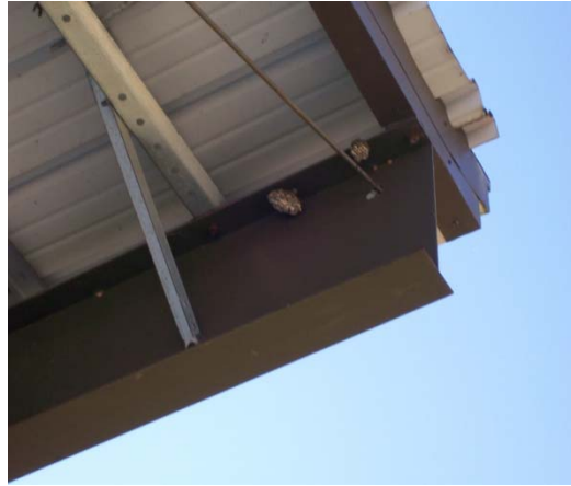
Example of wasp nests. If wasps are present this would be considered active, and would not meet desired maintenance conditions.
