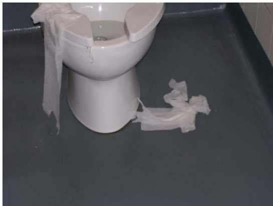
Scattered paper on the floor in stalls may not meet desired maintenance conditions.
