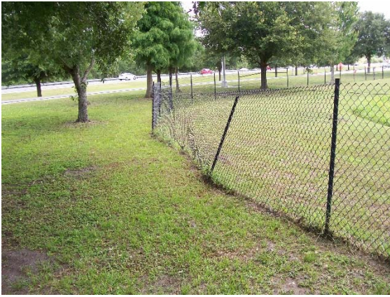
This fence will not meet desired maintenance conditions, because one post is missing and the fence fabric is not attached to the adjacent post.
