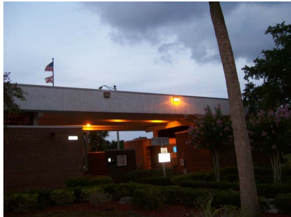
Example of building light not working.
