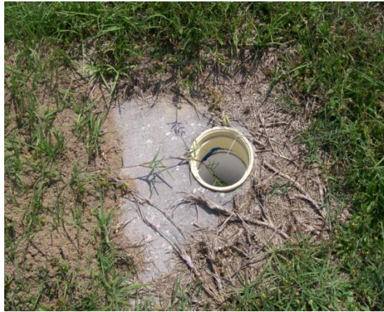
Missing valve cover in the common area this would not meet the desired maintenance conditions.
