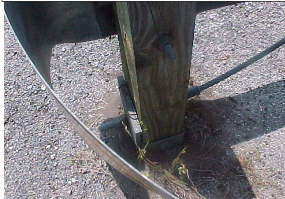
Secured bearing plate, nails in place, no rotation.
