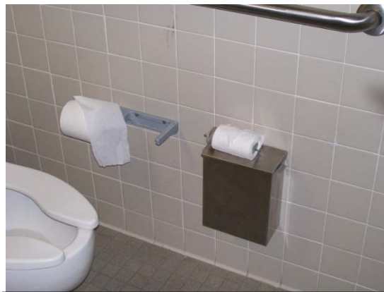
This dispenser is not in working order and would not meet desired maintenance conditions.
