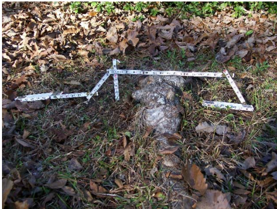
Tree root in picnic area measures 5 inches above the ground, this would not meet desired maintenance conditions.
