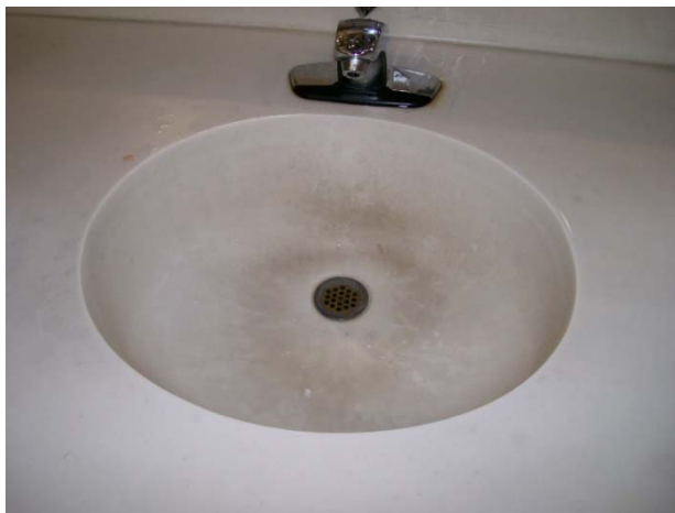
This basin is stained and would not meet desired maintenance conditions.
