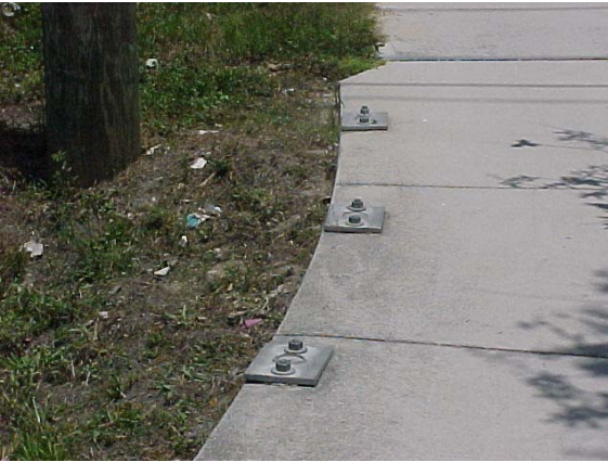
Missing handrail, this does not meet desired maintenance conditions.
