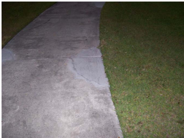
Sidewalk repaired, should be a smooth transition with no more than 1/4 inch misalignments.
