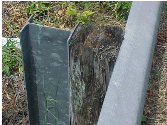
If more than 10% of the guardrail offset blocks are rotten and deteriorated. It will not meet desired maintenance conditions.
