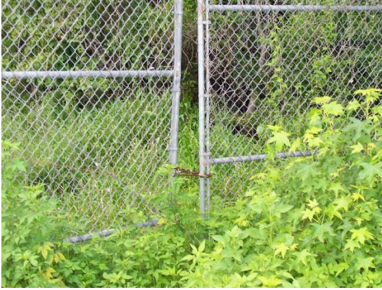
Opening between gates is greater than 6 inches and would not meet desired maintenance conditions.
