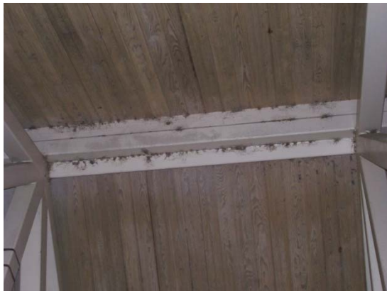
Example of cobwebs on ceiling.
