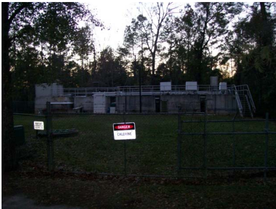
Photo of waste water treatment, appears to meet desired maintenance conditions.
