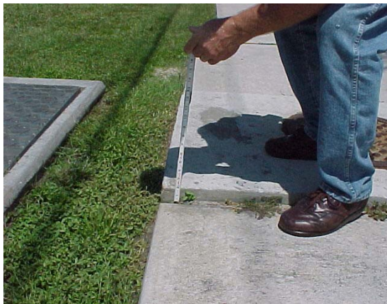
Misalignment greater than 1 1/2 inch, this would not meet desired maintenance conditions.
