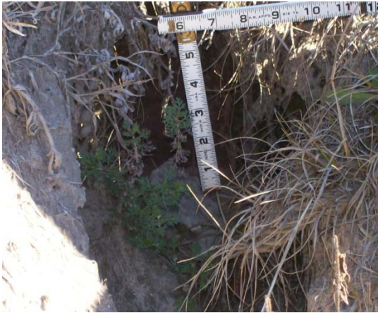
Large hole, 6 inches deep in the common and picnic area grounds this would not meet the desired maintenance conditions.
