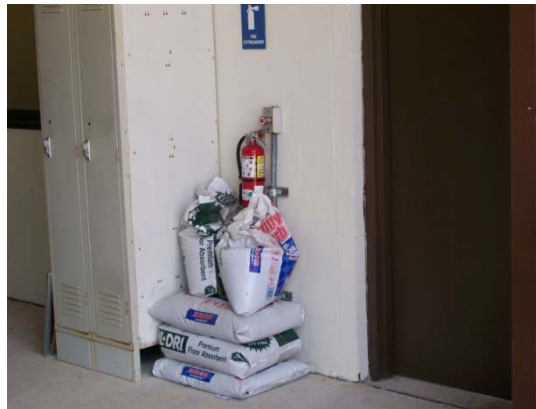
Extinguisher is obstructed; this would not meet desired maintenance conditions.
