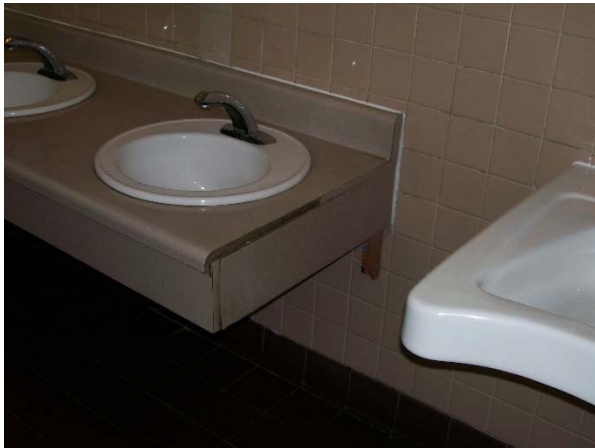
This countertop is missing its end cap trim and would not meet desired conditions.
