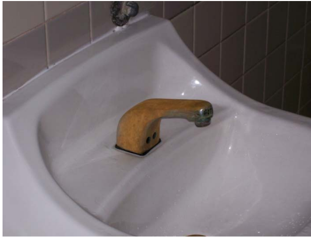
This faucet is corroded, or discolored, and would not meet desired maintenance conditions.
