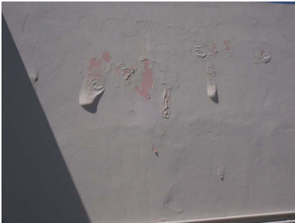
Wall with blistered and peeling paint, this possibly would not meet desired maintenance.
