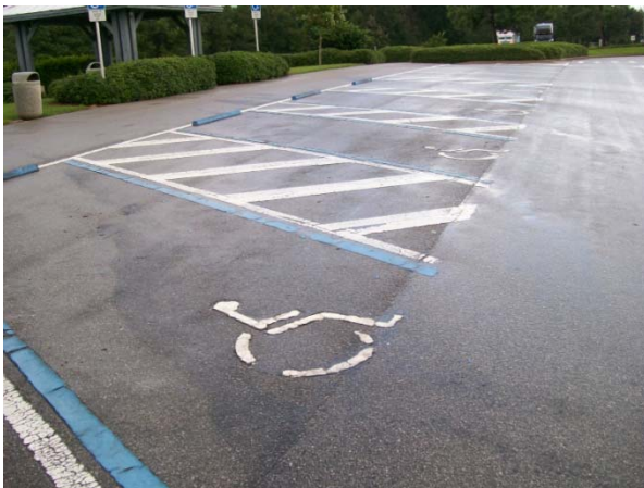
Symbol is faded and breaking up, measure total area to determine if it will meet desired maintenance conditions.
