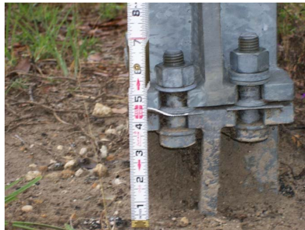
The slip base on this sign is more than 4 inches and would not meet desired maintenance conditions.
