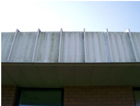
Roof/Fascia has dirt and mildew build-up.
