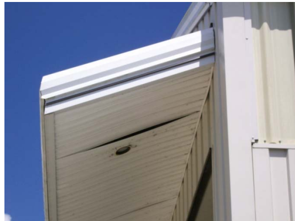
Soffit need to be repaired and cleaned.
