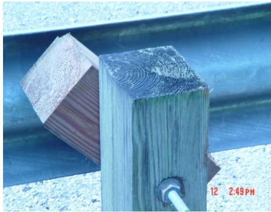
A guardrail block is considered twisted if there is a gap between the top edge of the block and the guardrail.
