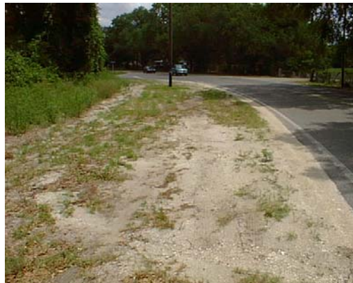
Example of more than 5 square feet of bare ground, this would not meet desired maintenance conditions.
