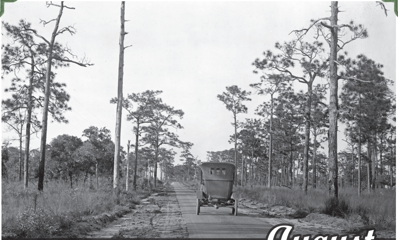
Polk County, 1917 Asphalt macadamized road from Haines City to Lake Hamilton
