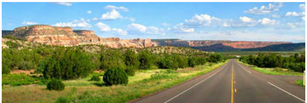
Figure 4-16. Dine’Bii’Tah “Among the People” Scenic Road runs through Canyon de Chelly National Monument, Window Rock Tribal Park, Navajo Nation Tribal Headquarters, Navajo Nation Museum, and the Ned A. Hatathli Museum, among many other points of interest.
