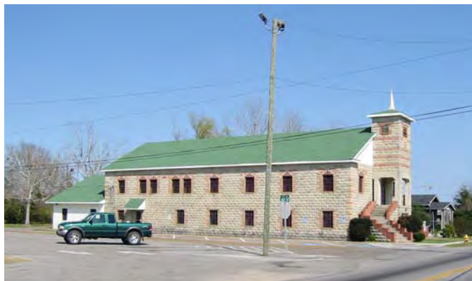
Figure 4-37. St. John Baptist Church at its 28th Street location.
