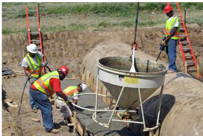
Figure 4-42. Red hats were worn by new job trainees for safety reasons to help all workers recognize them.
