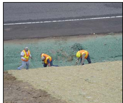
Straw matting and hydroseeding are effective erosion control measures.
