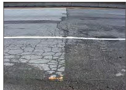
Cracked and deteriorated pavement on I-90.
