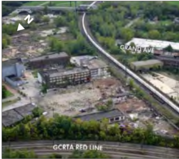
▲ Figure 4-32: The study area includes industrial properties that are vacant or no longer in use but that could contain polluted soil or groundwater.
