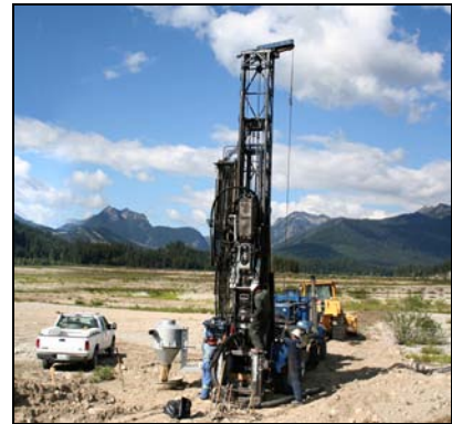
WSDOT would conduct work around Keechelus Lake during low pool elevations when the shoreline is exposed.
