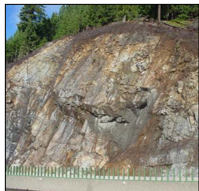
WSDOT may use rock netting at high risk locations throughout the project area.
