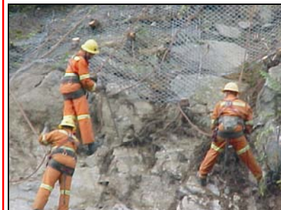
WSDOT installs rock bolts and netting to improve safety from rock fall within the project area.
