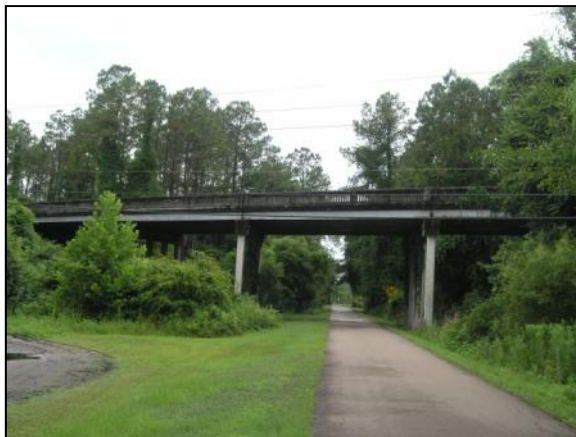
Photo 6-25. 1940 Baldwin Overpass, Duval County (No. 720026)
