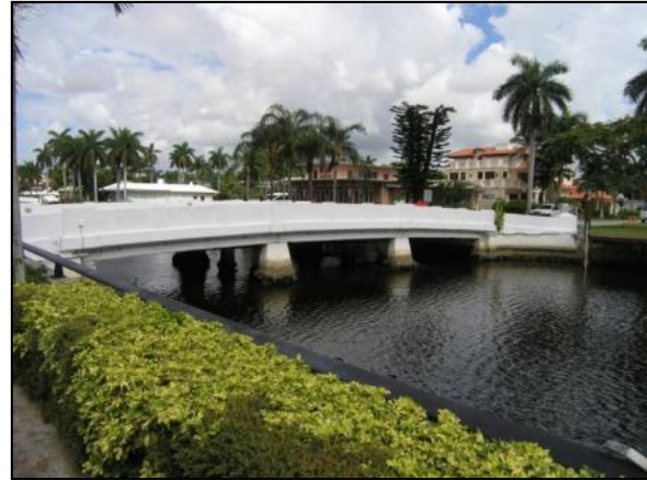
Photo 6-2. Royal Palm Drive Bridge (No. 865737)
