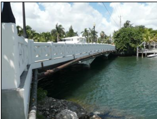
Photo 6-10. Venetian Causeway Bridge 5 (No. 874465)
