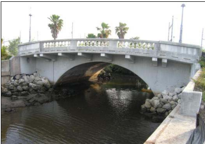
Photo 5-11. Moore's Creek Bridge, St. Lucie County (No. 945000)
