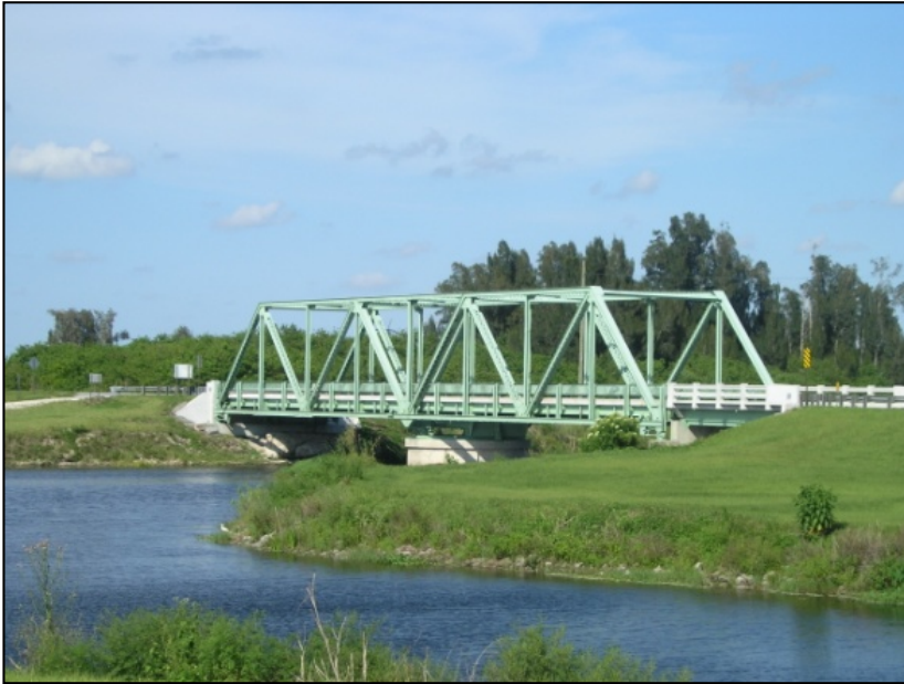
Photo 5-60. Loxahatchee Bridge/Twenty Mile Bend Bridge, Palm Beach County (No. 930940)
