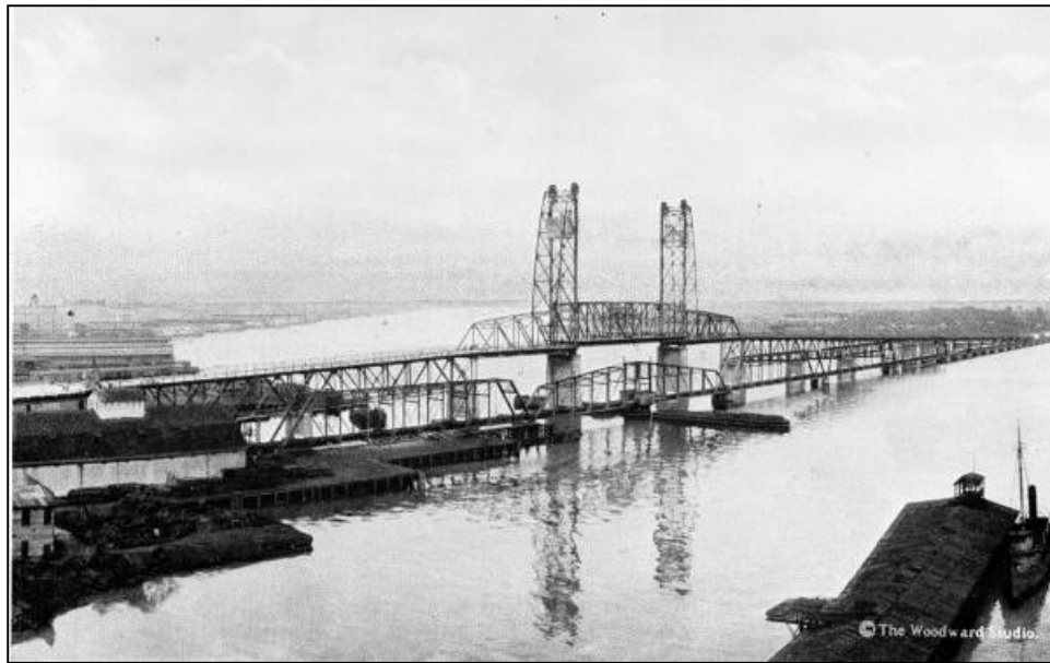
Photo 2-3. Acosta River Bridge over the St. Johns River. (Florida Photographic Collection)
