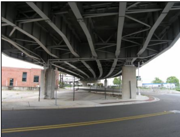
Photo 6-31. SR-228 (Leg G) Bridge (No. 720490)
