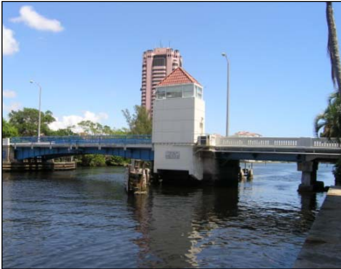
Photo 5-74. Clarence Geist Memorial Bridge/Camino Real Bridge/Boca Raton Club Bridge, Palm Beach County (No. 934408)
