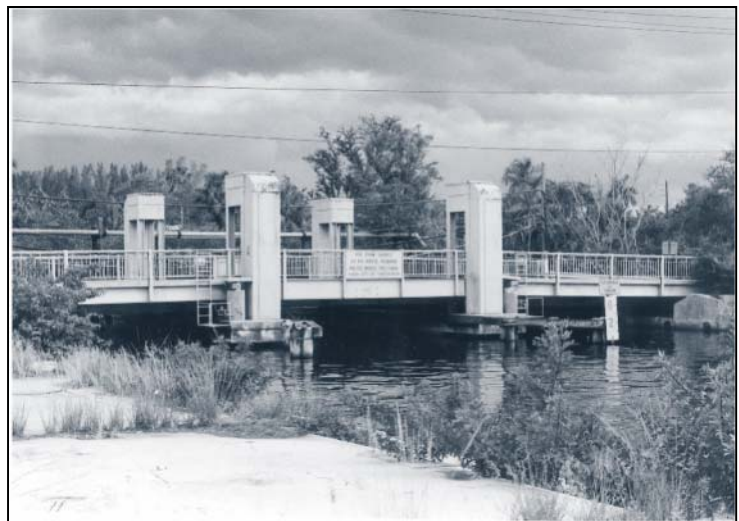
Photo 5-52. The Billy Creek Lift Bridge in Lee County is the Smallest Lift Bridge in Florida.
