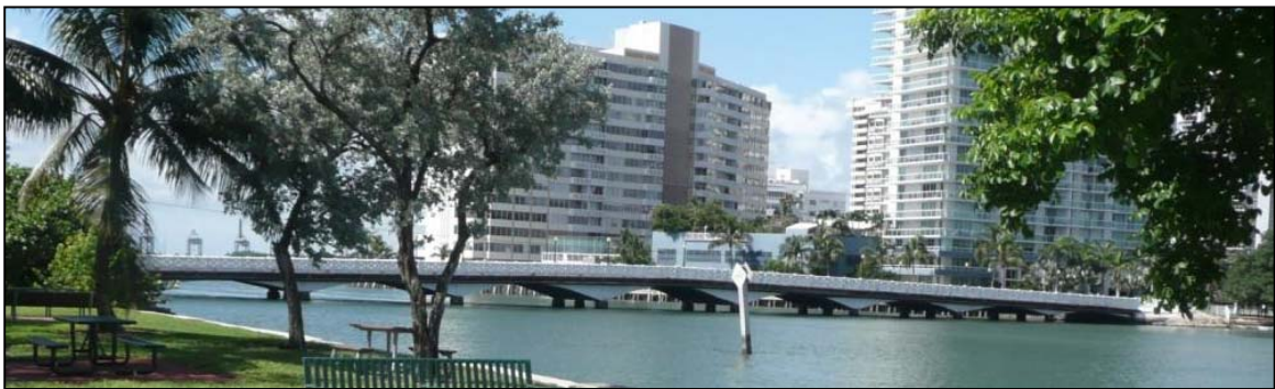
Photo 6-9. Venetian Causeway Bridge (No. 874481)
