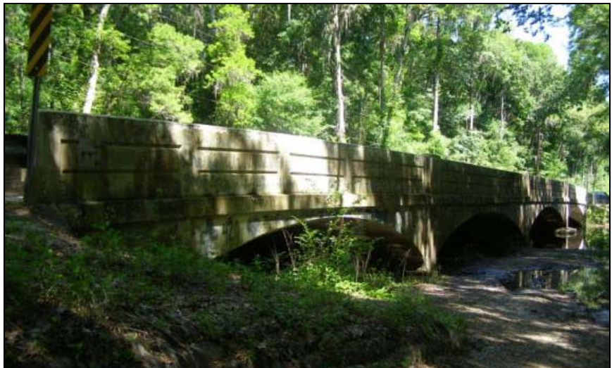
Photo 5-17. North Crystal Springs Bridge, Pasco County (No. 144002)
