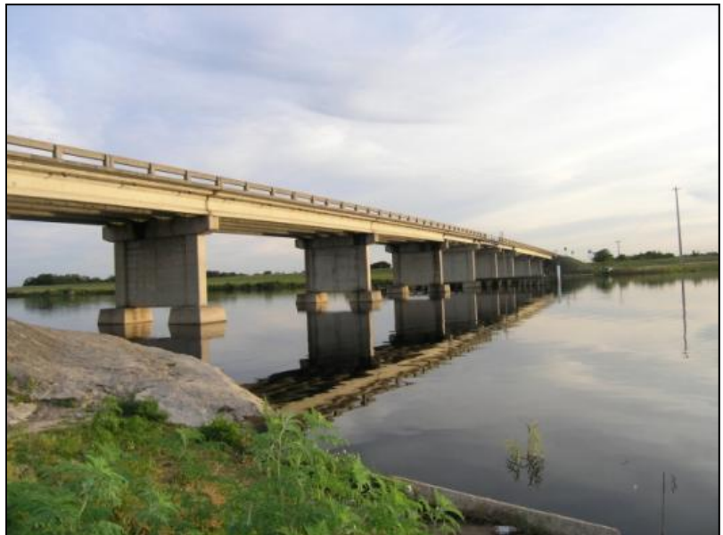
Photo 5-38. SR-78 Bridge, Okeechobee County (No. 910009)
