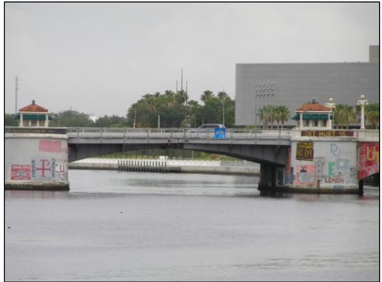
Photo 5-77. Kennedy Boulevard Bridge, Hillsborough County (No. 100100)
