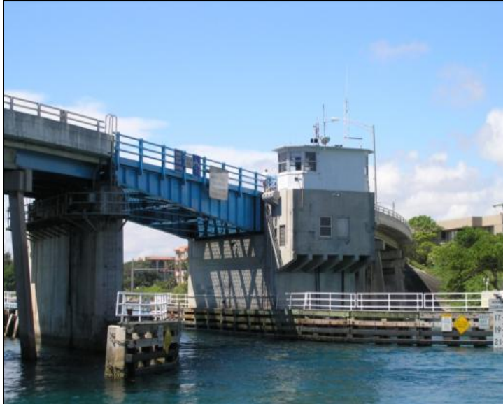
Photo 5-72. Boca Inlet Bridge, Palm Beach County (No. 930060)
