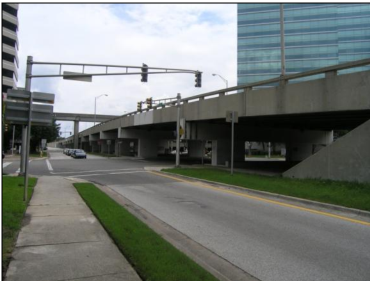
Photo 5-40. US-1/SR-5 Bridge over Miami Road, Looking Southwest, Duval County (No. 720087)
