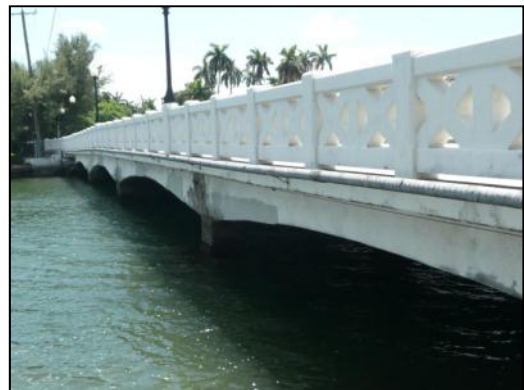
Photo 6-11. Venetian Causeway Bridge 7 (No. 874471)
