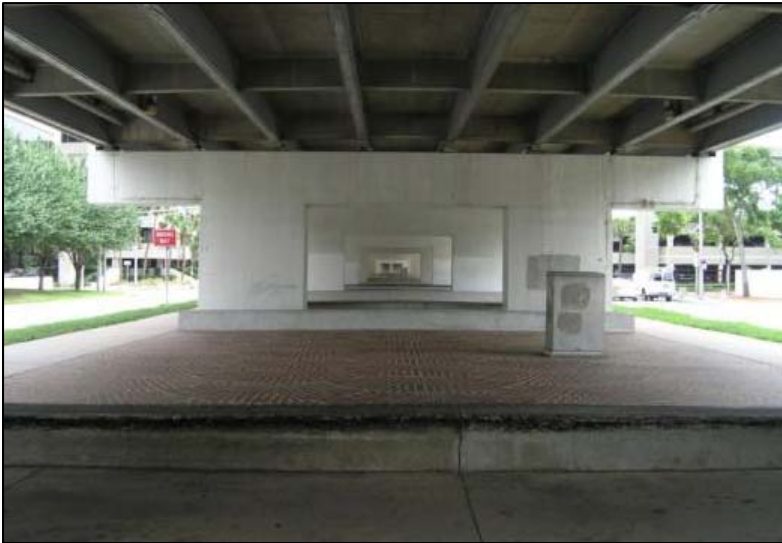
Photo 5-41. Plaza beneath Bridge No. 720087, Duval County
