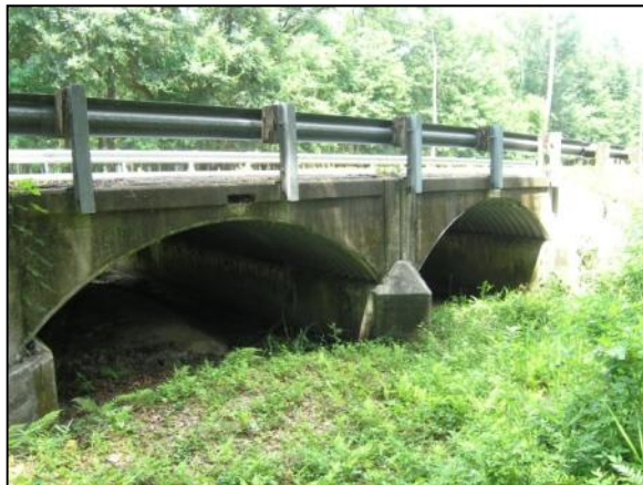
Photo 6-21. CR-18/Sampson River Branch Culvert, Bradford County (No. 280038)
