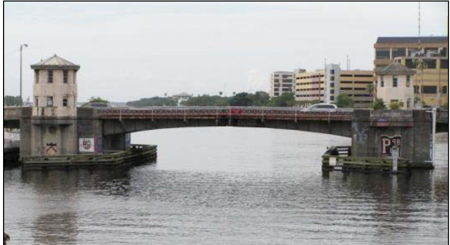
Photo 5-78. Platt Street Bridge, Hillsborough County (No. 105500)
