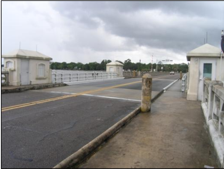
Photo 5-65. Ortega River Bridge, Duval County (No. 720005)
