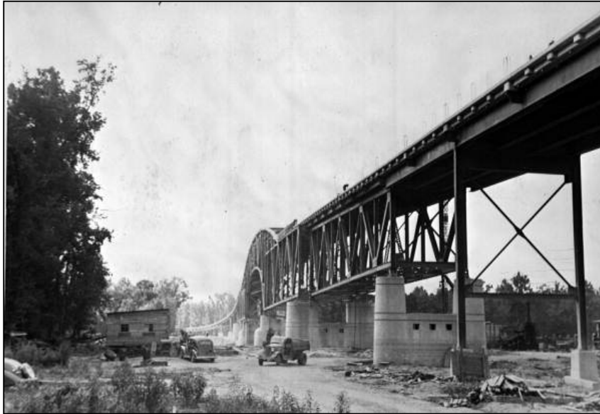
Photo 2-7. Construction of Blountstown Bridge Nearing Completion, 1937. ( Florida Photographic Collection )
