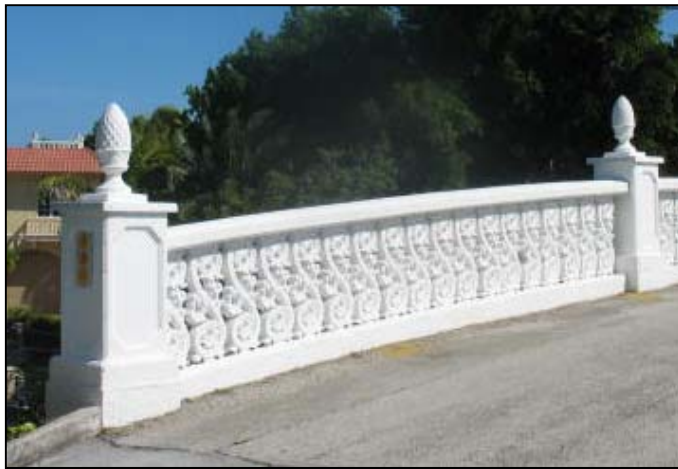
Photo 6-5. Harbour Bridge (No. 904604)
