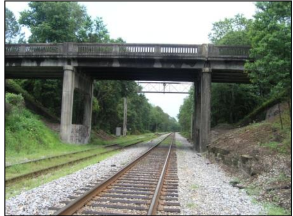
Photo 6-24. US-301/SR-200 over SCL RR, Nassau County (No. 740022)
