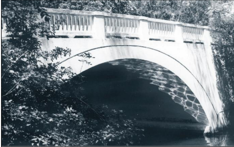
Photo 7-14. Original Appearance of the Granada Boulevard Bridge.
