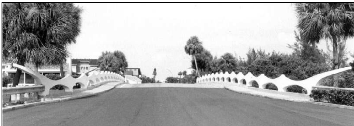
Photo 7-12. The 13 th Street Bridge from its Western Approach.
