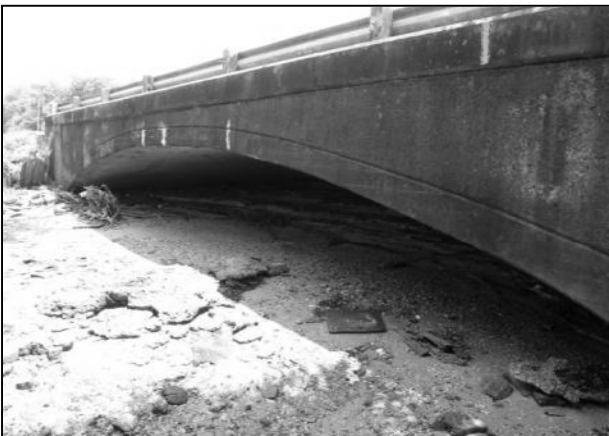
Photo 2-6. Remnant 1940 Memorial Causeway Overflow Bridge, FDOT #764038, Putnam County.
