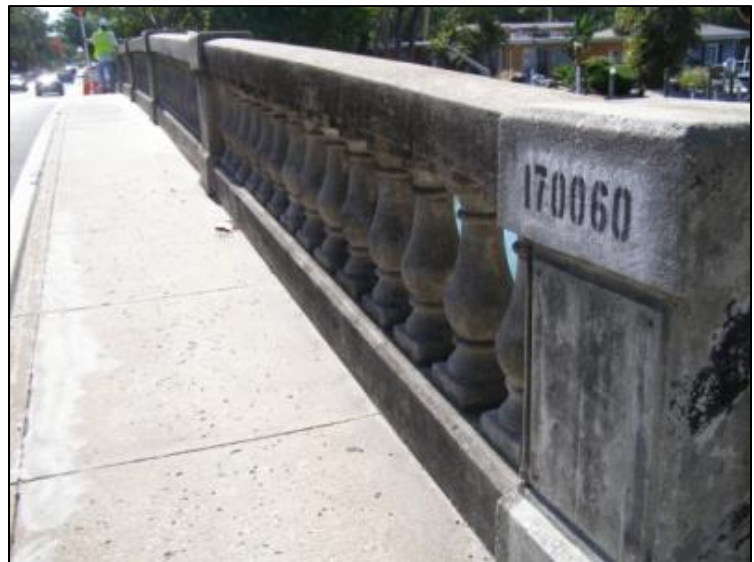
Photo 5-26. Hanson Bayou Bridge, Sarasota County (No. 170060)
