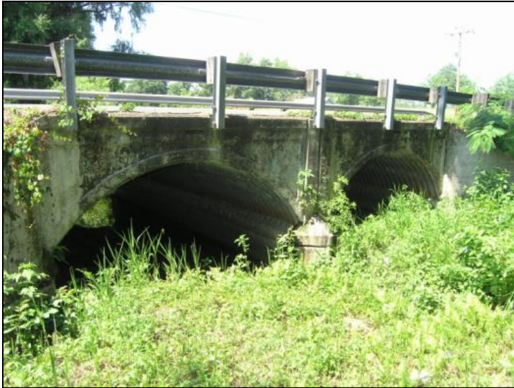
Photo 5-48. CR-18 over Braggs Branch, Bradford County (No. 280036)
