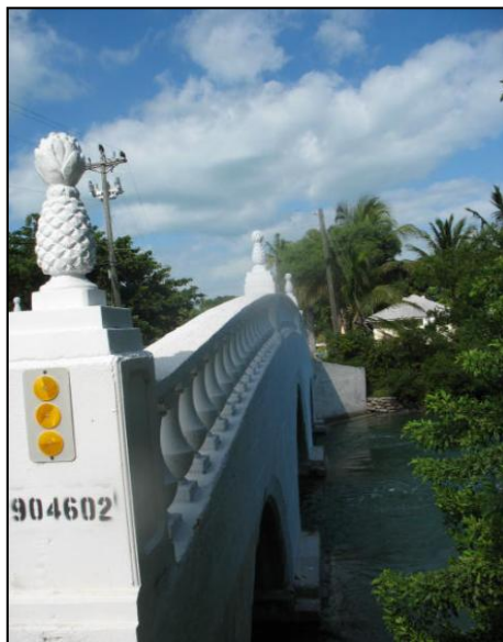
Photo 6-3. Truman Bridge (No. 904602)
