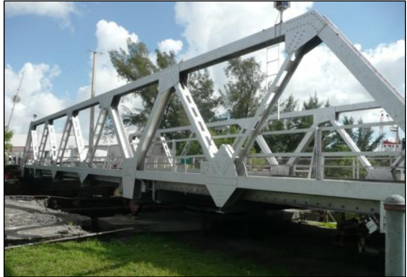
Photo 5-63. Tamiami Canal/NW South River Dr. Swing Bridge, Miami-Dade County (No. 874135)
