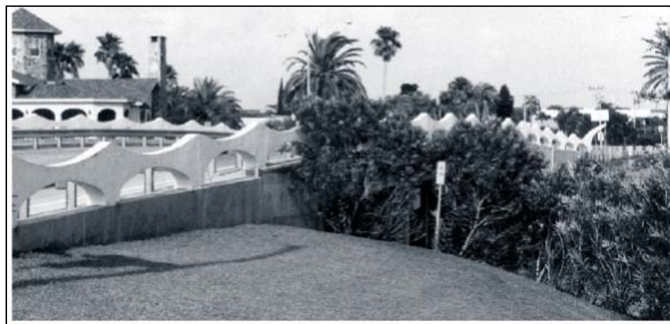
Photo 7-11. The Unique Railings of the Madonna Boulevard Bridge Reflect a Neo-Expressionist Styling.
