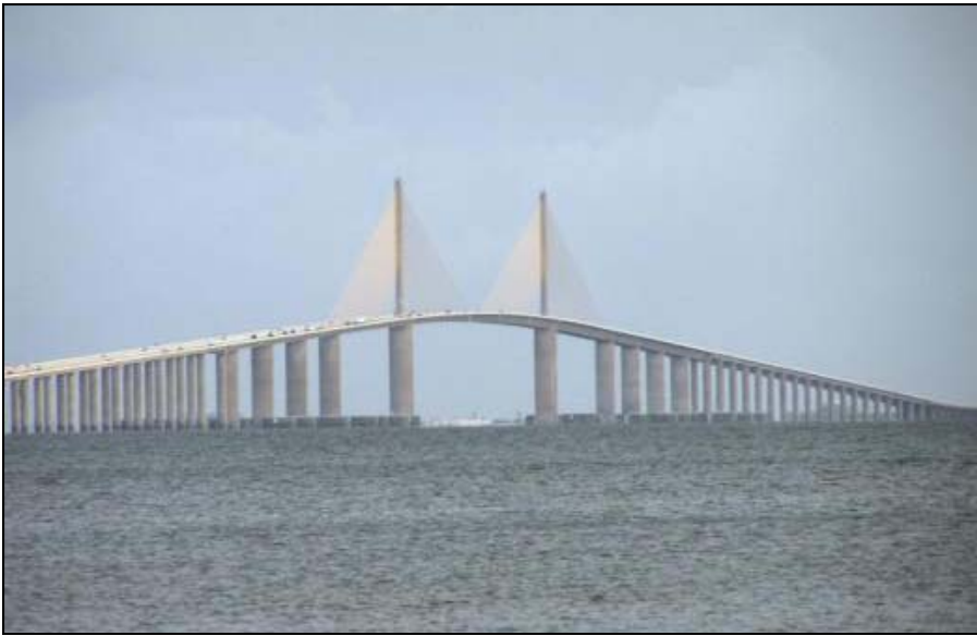
Photo 5-47. Bob Graham Sunshine Skyway Bridge (No. 150189)
