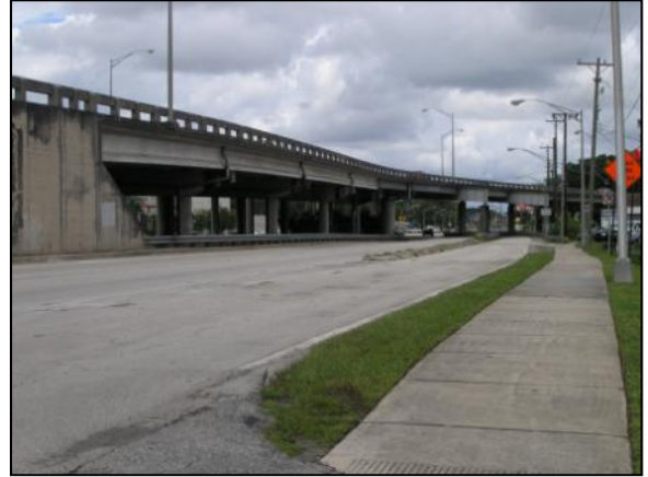
Photo 6-30. SR-228 at US-90 Steel Girder Bridge (No. 720113)
