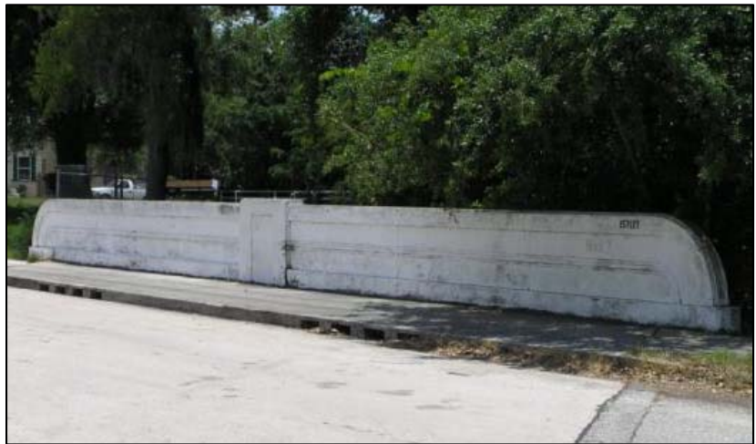
Photo 5-35. Burlington Avenue Bridge, Pinellas County (No. 157127)
