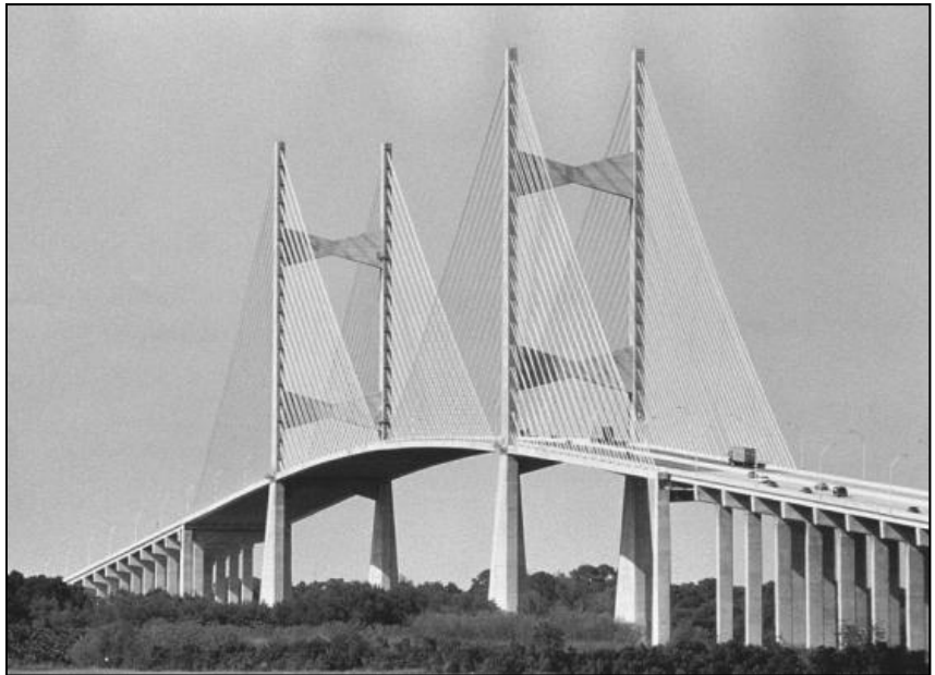
Photo 5-46. Dames Point Bridge, Duval County (No. 720518)
