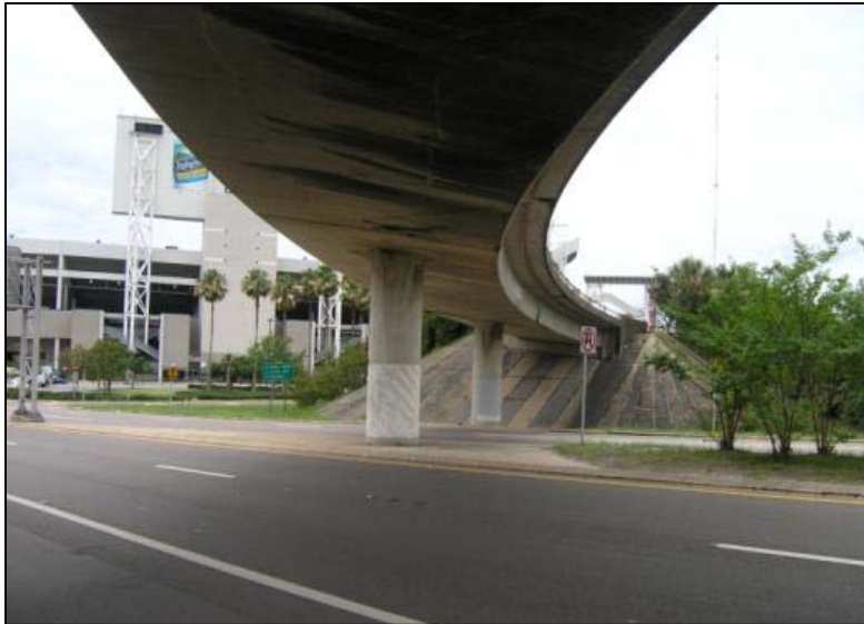
Photo 5-36. SR-115A Flyover to SR-10A, Duval County (No. 720100)
