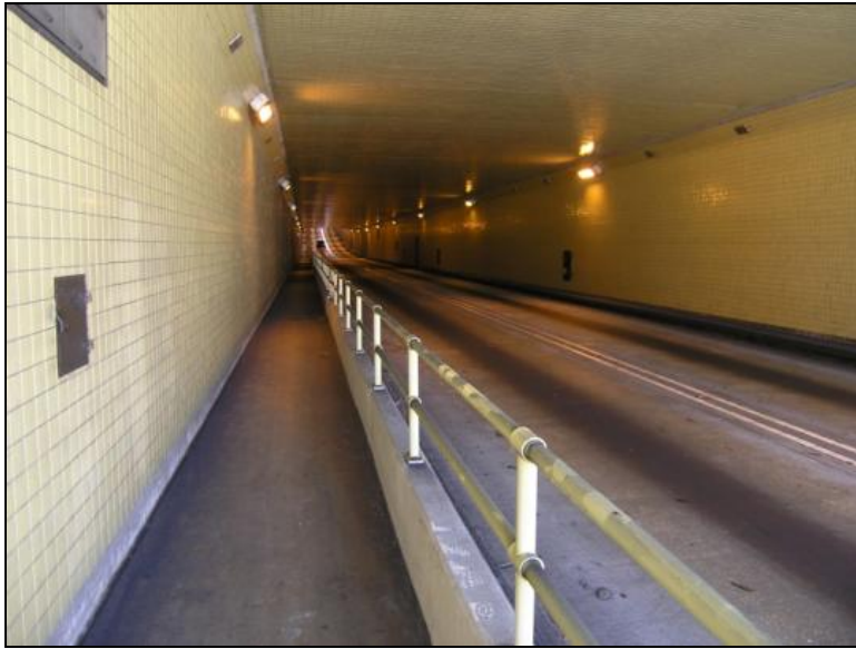
Photo 5-84. Henry Kinney Tunnel - Interior, Broward County (No. 764039)
