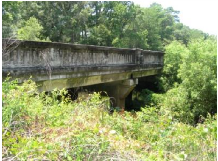
Photo 5-29. Ten Mile Creek Bridge, Levy County (No. 340045)
