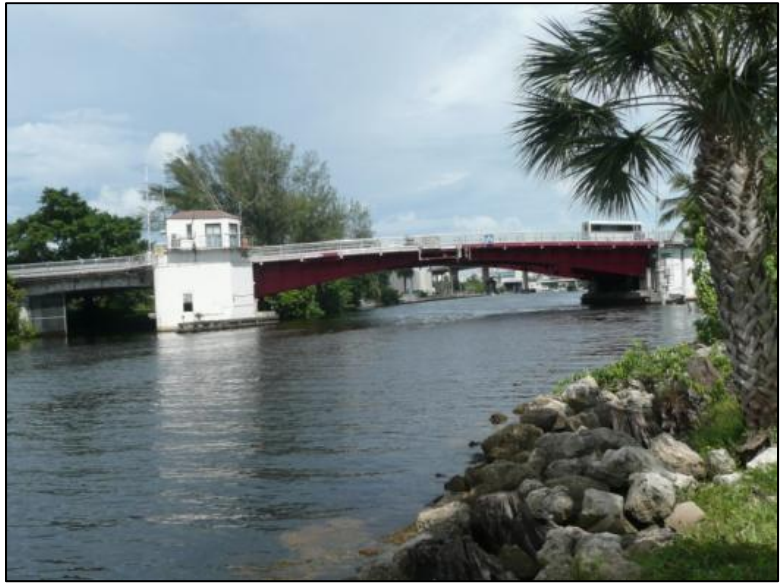
Photo 5-76. NW 17 th Avenue Bridge, Miami-Dade County (No. 874161)
