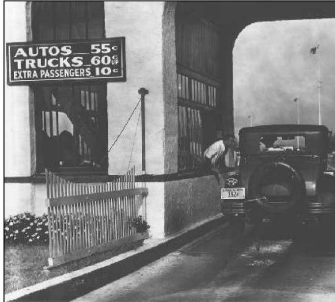
Photo 2-4. Gandy Bridge Toll Gate, 1930.
