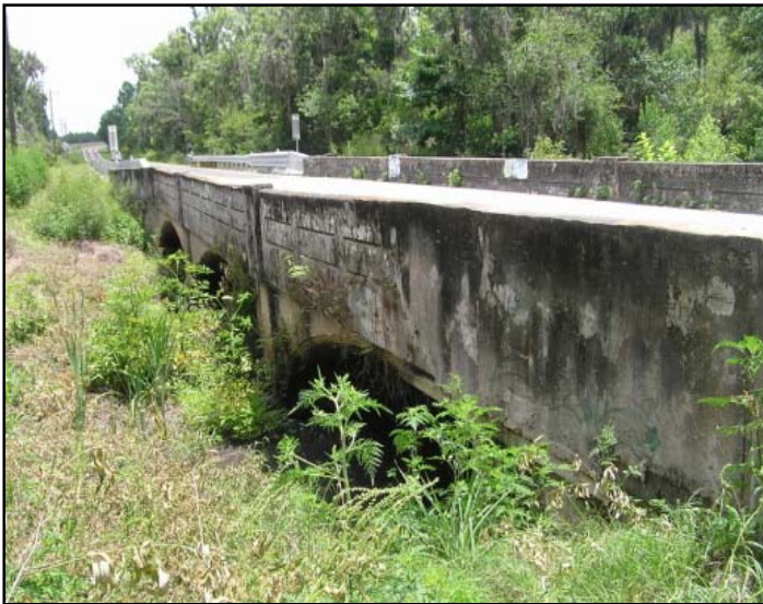
Photo 5-7. Little Payne Creek Bridge, Hardee County (No. 060034)
