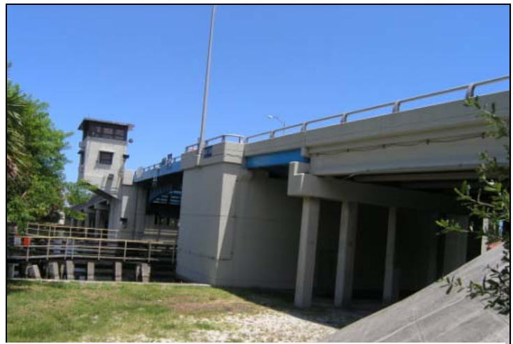
Photo 5-69. Davie Boulevard Bridge, Broward County (No. 860038)
