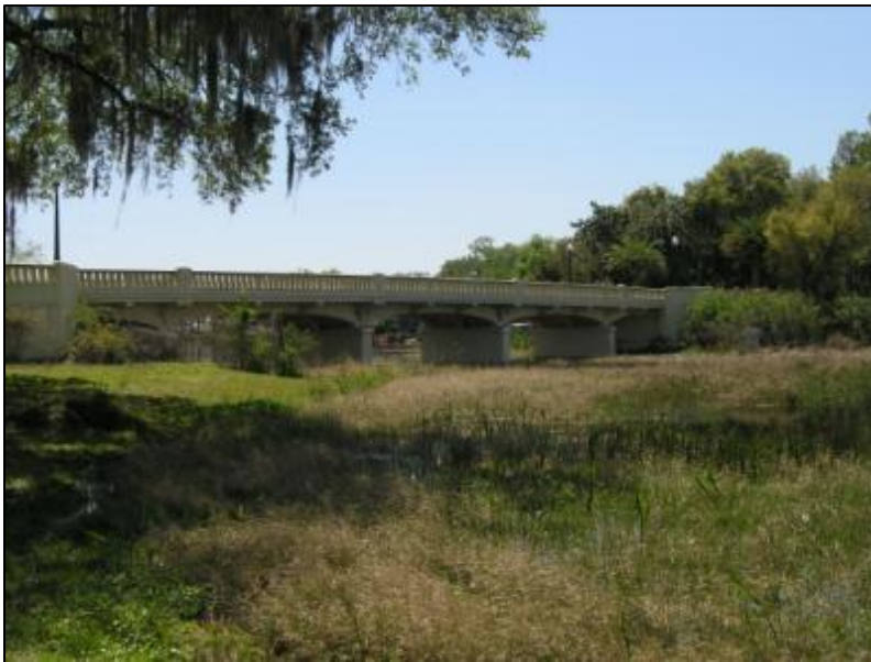
Photo 5-32. Lake Conway Bridge, Orange County (No. 755100)
