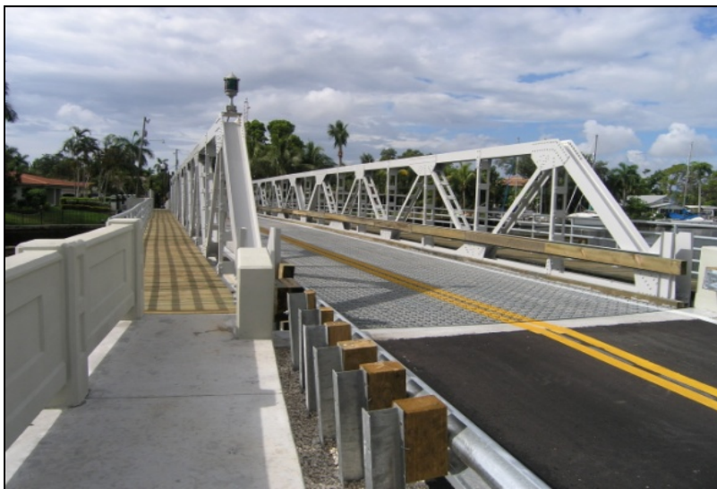
Photo 5-59. Snow-Reed Swing Bridge/Southwest 11 th Street Swing Bridge, Broward County (No. 865748)
