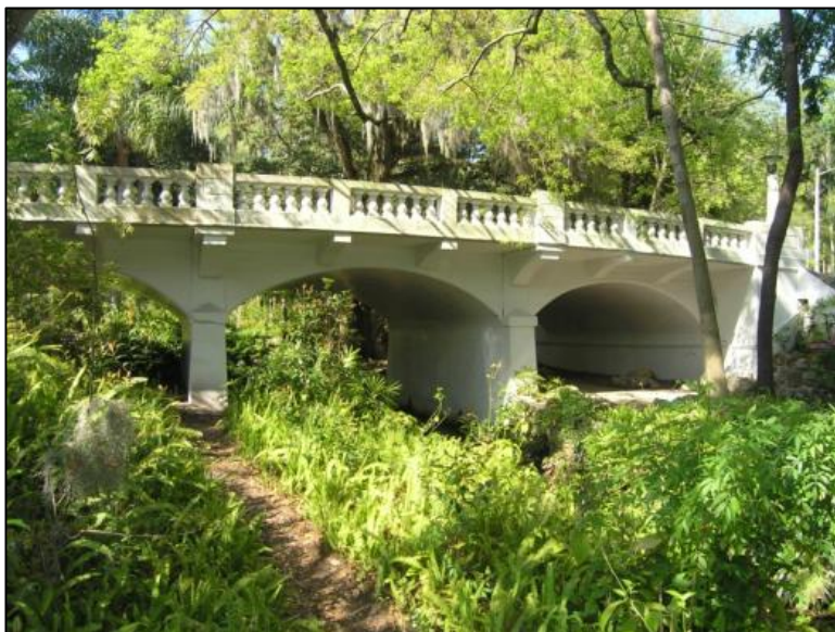
Photo 5-14. Washington Street Bridge, Orange County (No. 755806)
