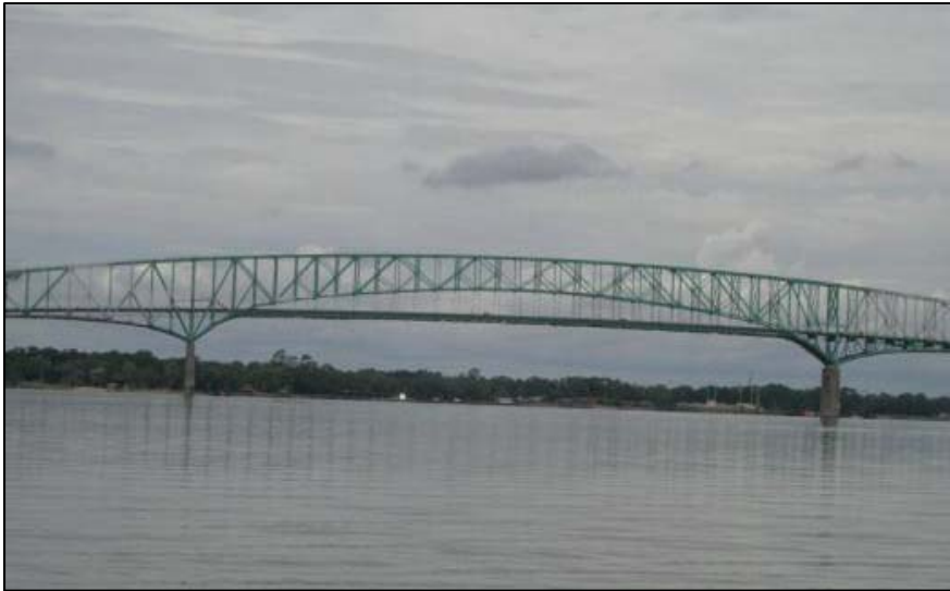
Photo 5-4. Hart Bridge, Duval County (No. 720107)
