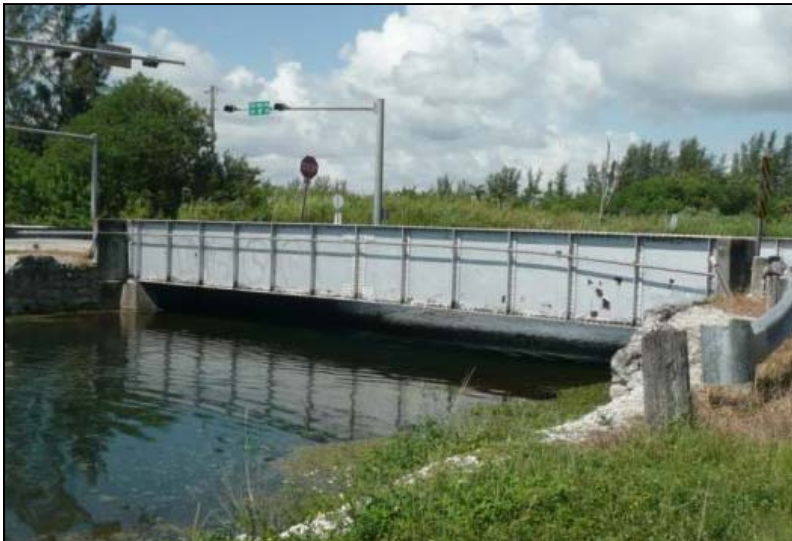
Photo 5-44. SW 117 th Avenue Bridge, Miami-Dade County (No. 874307)
