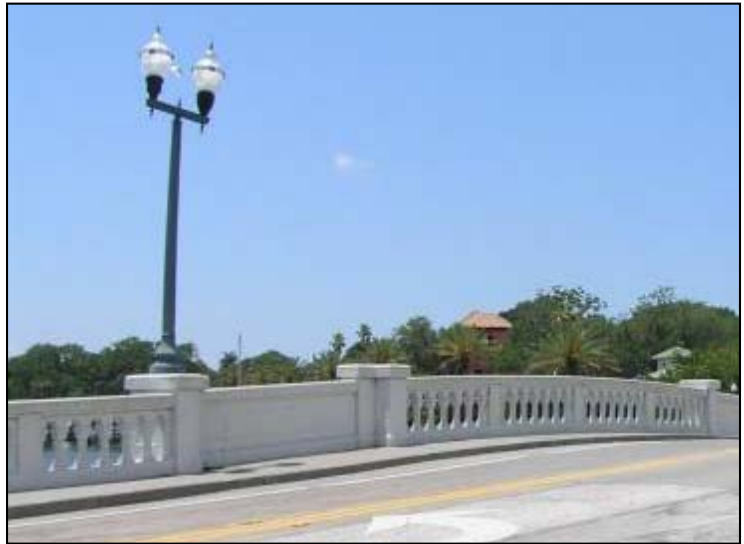
Photo 5-34. Snell Isle Bridge, Pinellas County (No. 157191)
