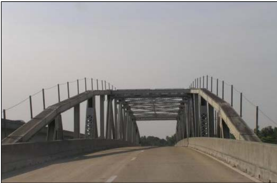
Photo 5-2. Blountstown Truss Bridge, Calhoun County (No. 470029)
