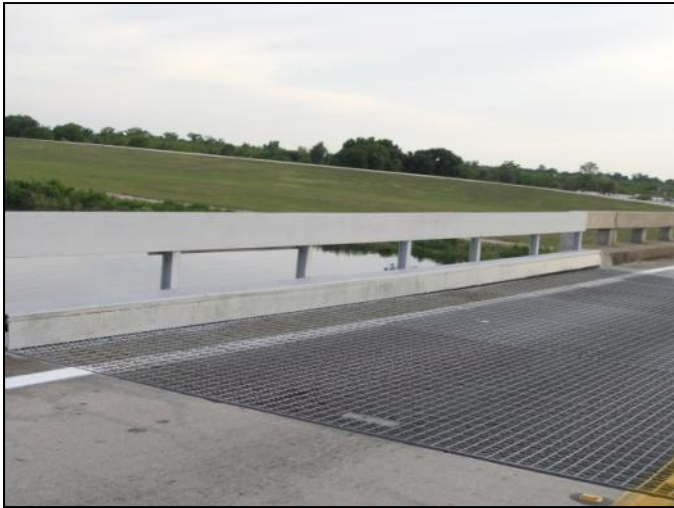
Photo 5-39. SR-78 Bridge (No. 910009) - Removable Span
