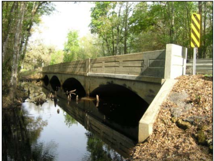
Photo 5-13. Deep Creek Arch Deck, Volusia County (No. 794081)
