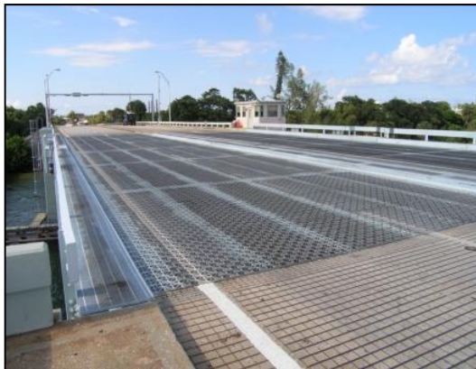
Photo 7-6. Main Four-Leaf Bascule Span of Jupiter US-1/SR-5 Bascule Bridge, Palm Beach County (No. 930005).
