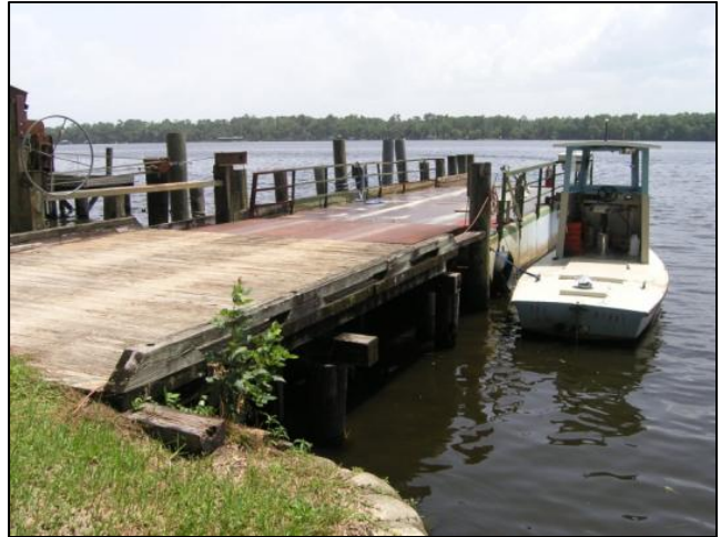
Photo 5-86. Barge Operation: Fort Gates Ferry, Putnam County (No. 764039)
