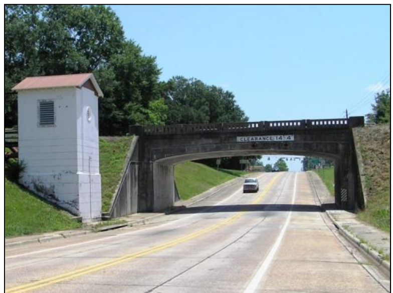
Photo 5-21. Atlanta and St. Andrews Bay Railway Frame Bridge, Jackson County (No. 530003)
