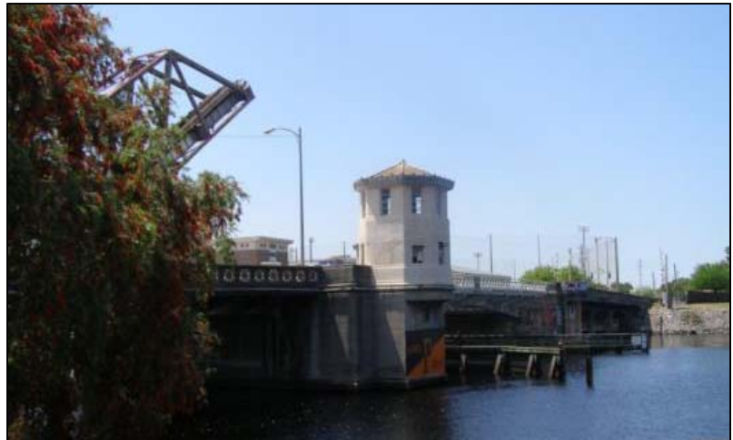
Photo 5-80. Cass Street Bridge, Hillsborough County (No. 105502)
