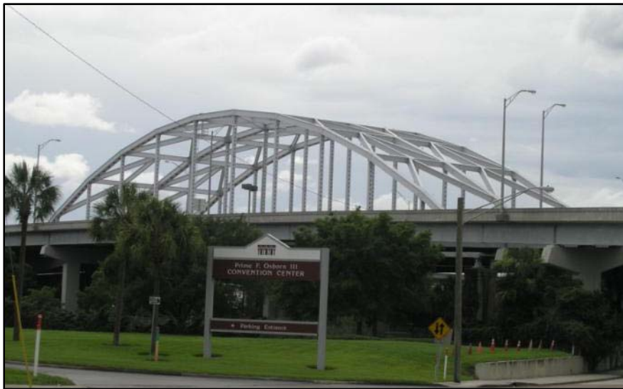
Photo 5-9. Myrtle Avenue Overpass, Duval County (No. 720163)
