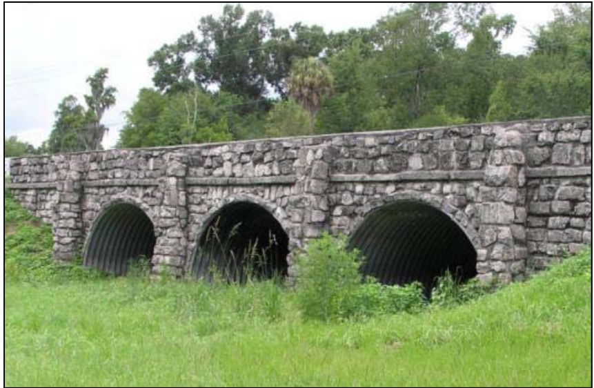
Photo 5-50. Blackwater Creek Relief Structure, Hillsborough County (No. 100647)
