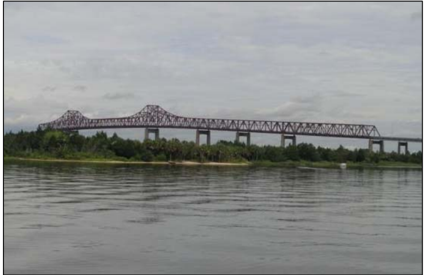
Photo 5-3. Mathews Bridge, Duval County (No. 720076)
