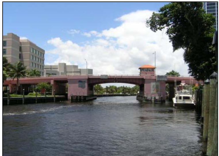
Photo 5-71. SE 3 rd Avenue Bridge, Broward County (No. 864071)
