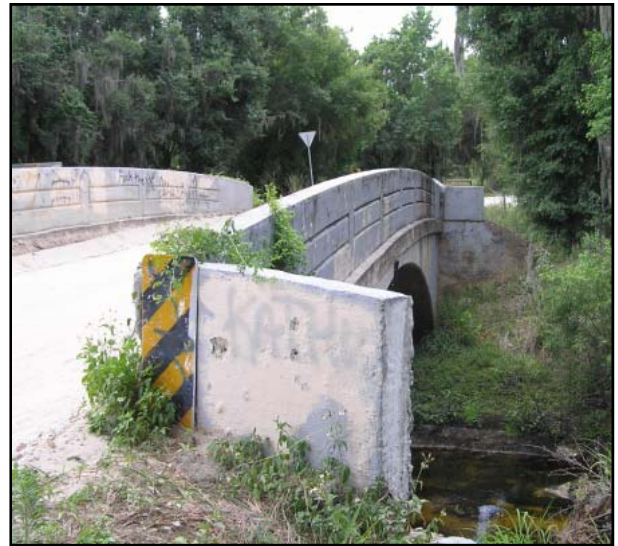
Photo 5-8. Payne Creek Bridge, Hardee County (No. 064069)
