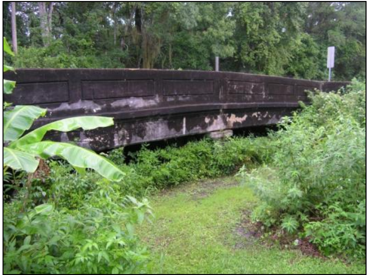
Photo 5-24. Old US-17 over Crescent Lake Outflow, Putnam County (No. 764044)
