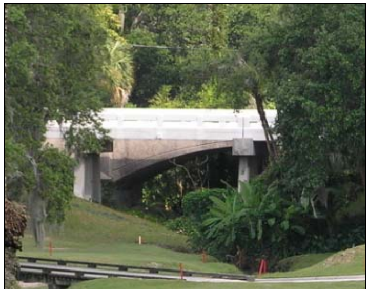
Photo 5-20. Luten “Half-Arch” Bridge, Pinellas County (No. 159901)
