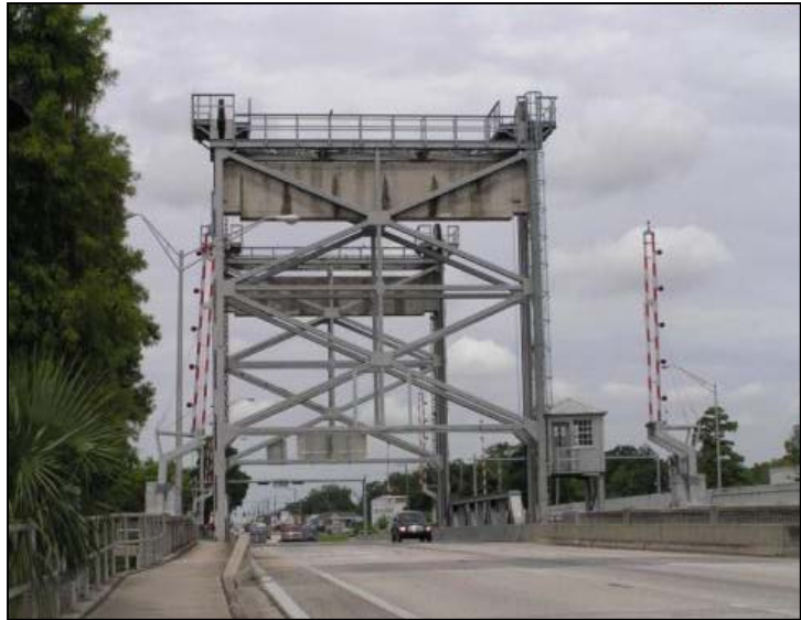
Photo 5-54. Hillsborough River Lift Bridge, Hillsborough County (No. 100920)
