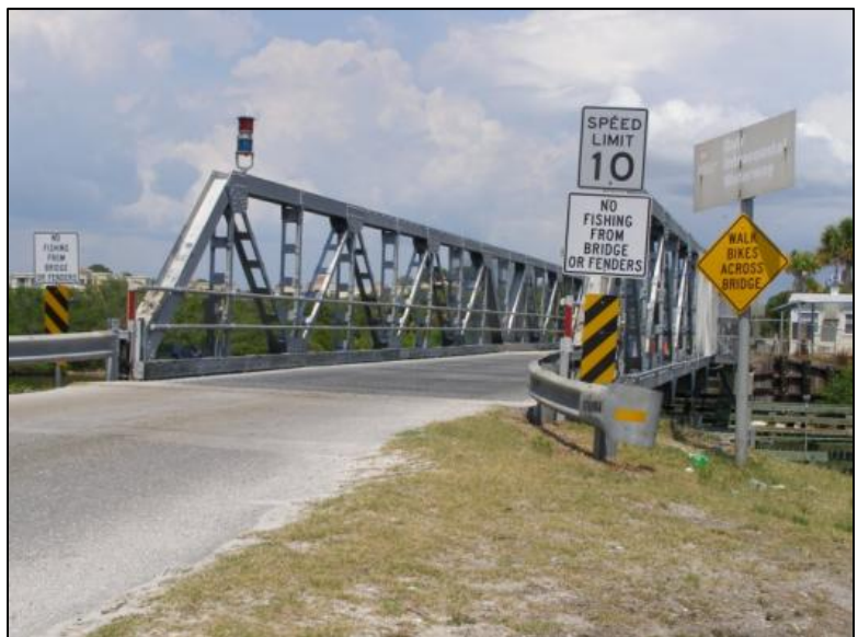
Photo 5-56. Blackburn Point Swing Bridge, Sarasota County (No. 170064)
