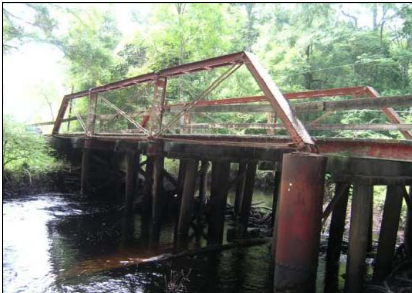
Photo 5-1. Steinhatchee Springs Bridge, Lafayette County (No. 334001)
