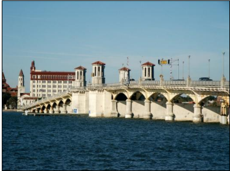
Photo 5-67. Bridge of Lions, St. Johns County (No. 780074)
