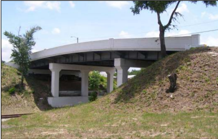
Photo 5-37. Haines City Overpass, Polk County (No. 165700)
