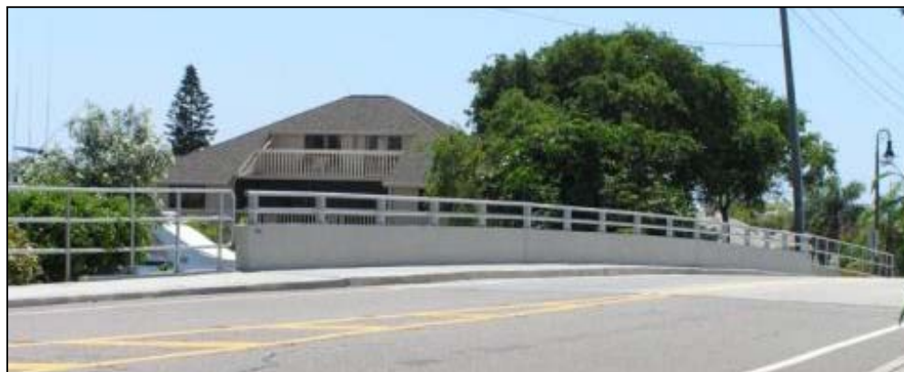
Photo 7-13. Madonna Boulevard Bridge with Replaced Railing, June 2010.
