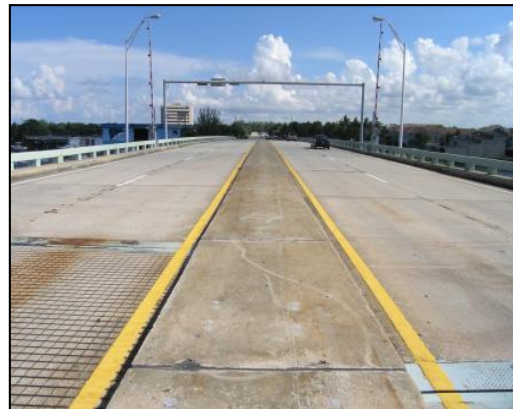
Photo 7-7. Looking East from the Main Span of the Jupiter US-1/SR-5 Bascule Bridge.
