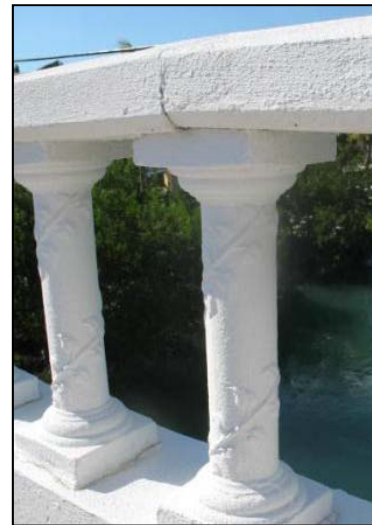
Photo 6-6. Rosen Bridge (No. 904606)
