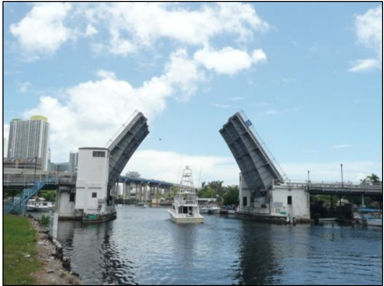
Photo 5-75. SW 1 st Street Bridge, Miami-Dade County (No. 870660)
