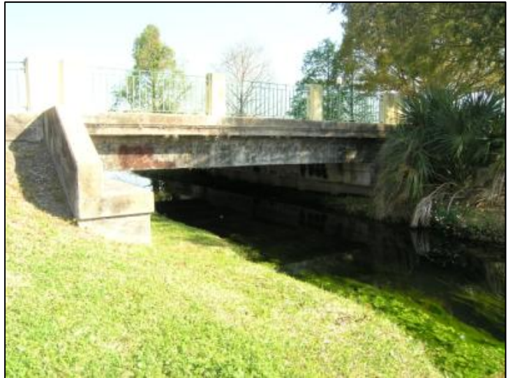
Photo 5-31. Poinsettia Avenue Bridge, Orange County (No. 755807)
