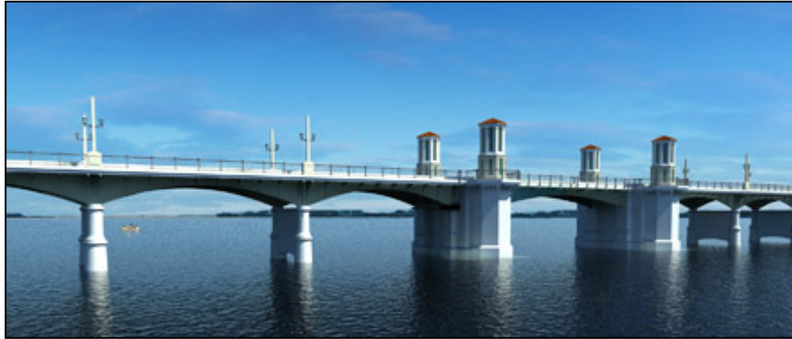
Photo 5-68. View of the Rehabilitated Bridge of Lions
