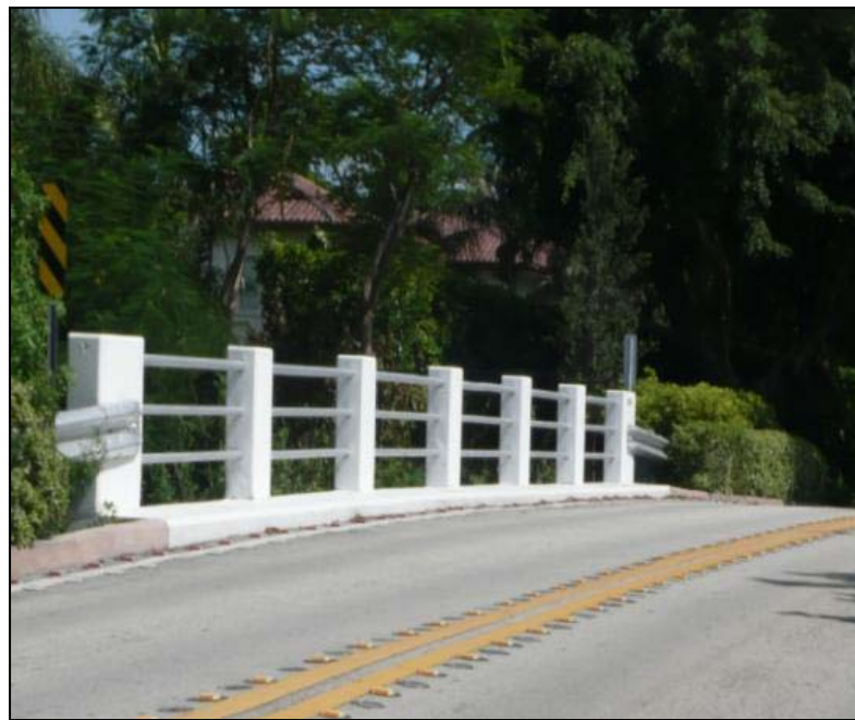
Photo 7-15. The Granada Boulevard Bridge with Replaced Railing, 2010.
