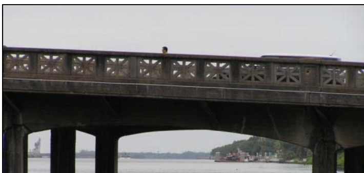
Photo 5-79. Detail of Eight-Point Star Railing Decoration.
