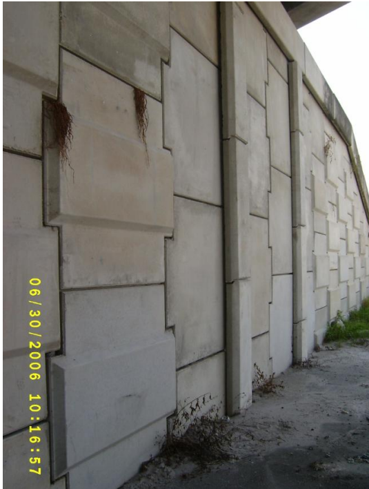
Figure 10, slip joints
