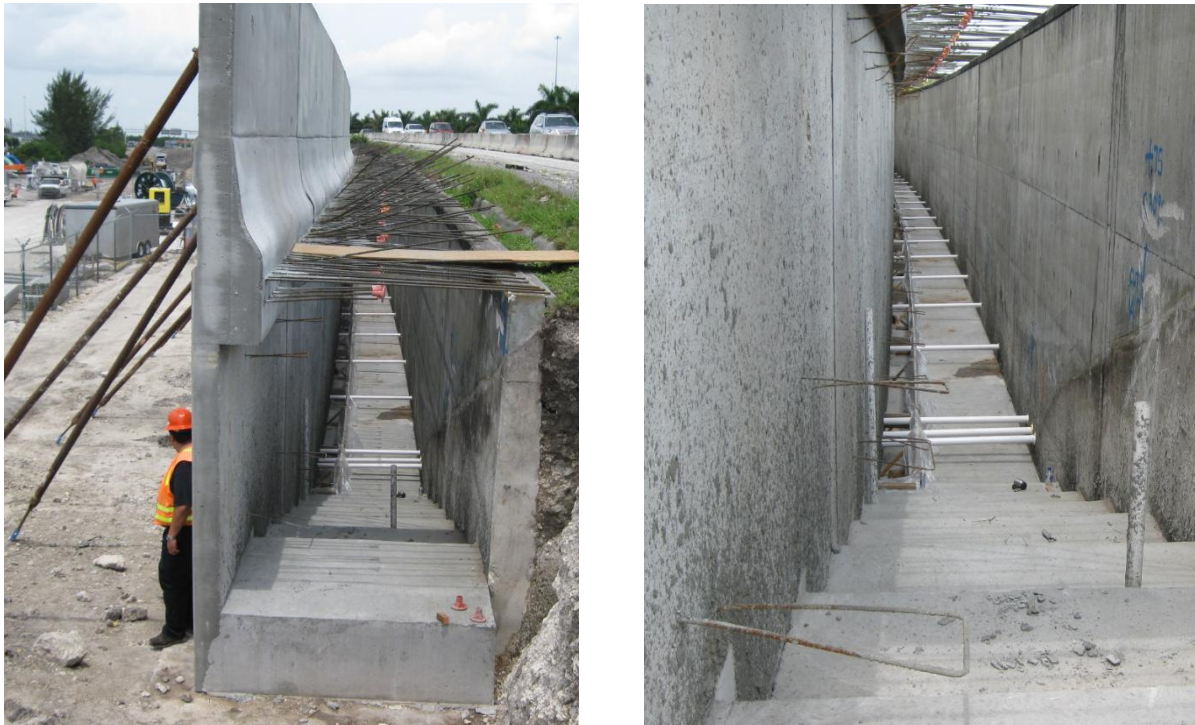
Figure 60, Cellular Concrete Wall
