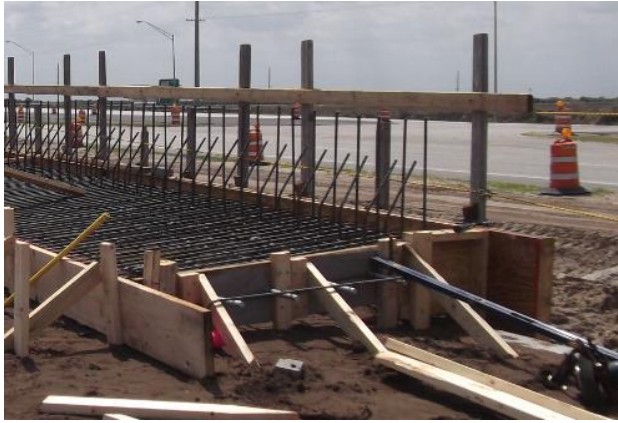
Figure 27, Barrier with Slab. Cast-in-place
