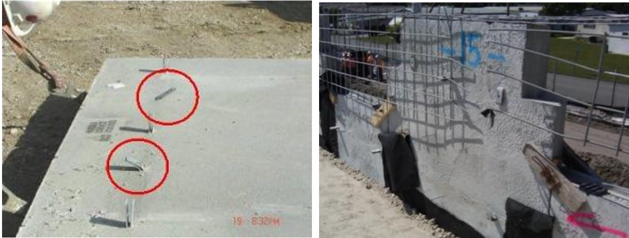
Figure 15, Damaged Tabs
