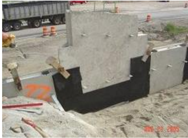
Fig 24, Filter Fabric installed at the joints
