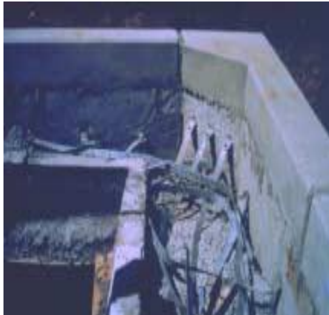
Figure 36, Not Proper Avoidance of Drainage Structure
