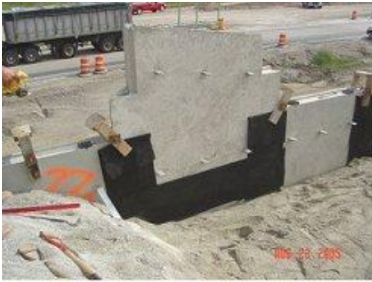
Figure 45, Attach Filter Fabric
