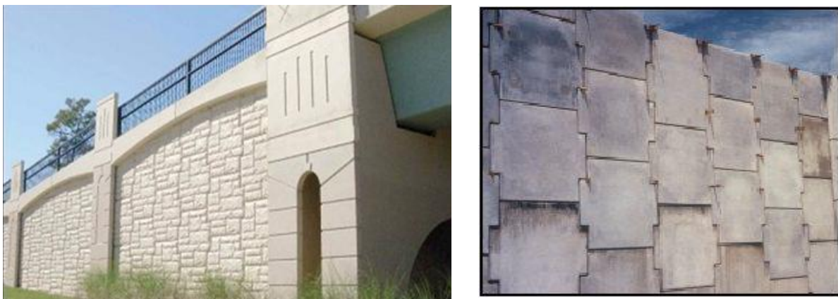
Figure 5, Panel Finishes and Shapes: top left: square panels, top right: diamond, bottom left: finish stone panels, bottom right: cruciform panels
