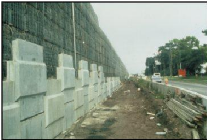
Figure 41, Temporary and Permanent Wall Facings
