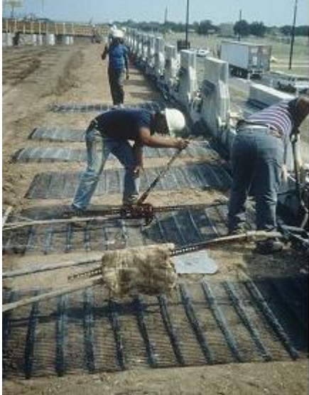
Figure 18, Geosynthetic Reinforcement (Extensible)
