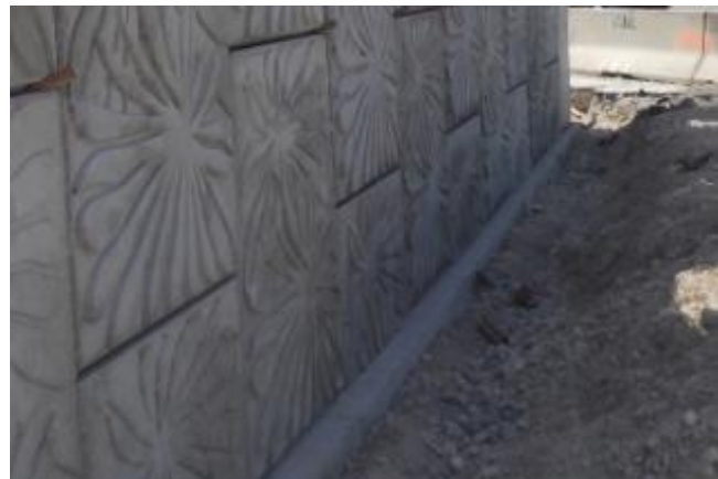
Figure 3, Leveling Pad
