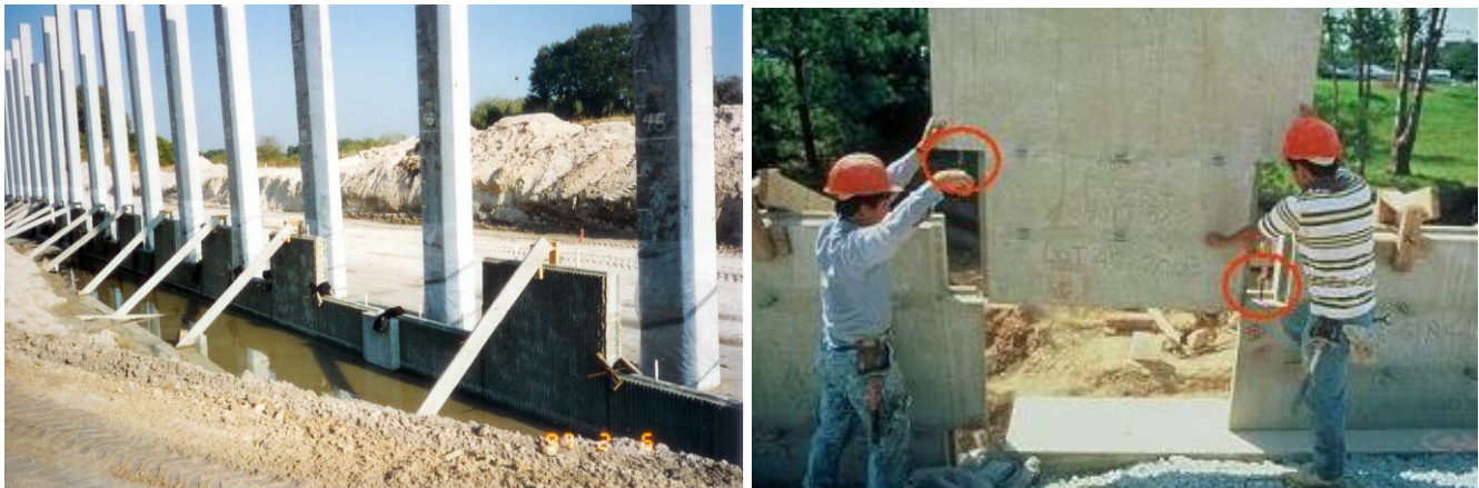
Figure 8, Placing and bracing Panels.
