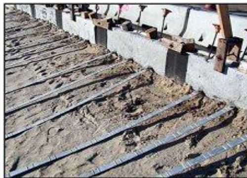
Figure 22, Reinforcement Connections
