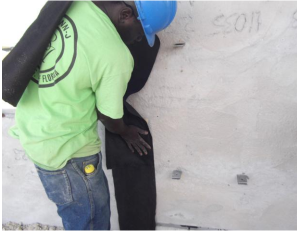
Figure 23, Filter Fabric installation
