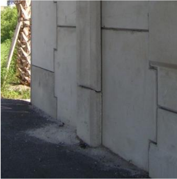
Figure 25, Loss of backfill through improperly constructed joint and filter fabric (Left: backfill washed through joint deposited next to the slip panel. Right: Void as observed from the top of wall)
