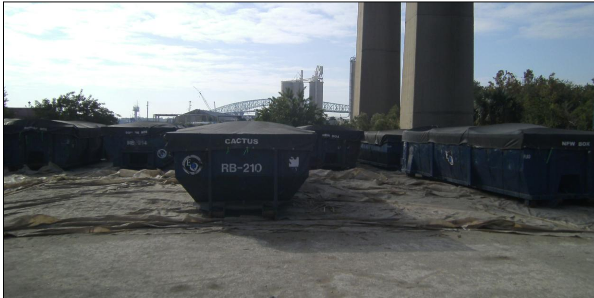
Spent Abrasive Media and Removed Paint Storage
