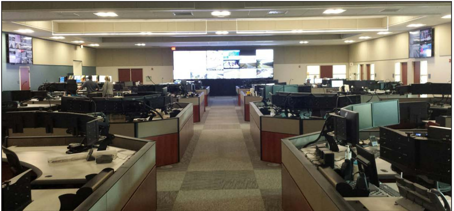
District Two's new North Florida RTMC.
