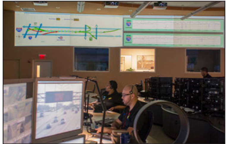
Speed data projected onto vacant walls in the TMC control room, and real-time performance measures and incident data are readily available on the video wall.
