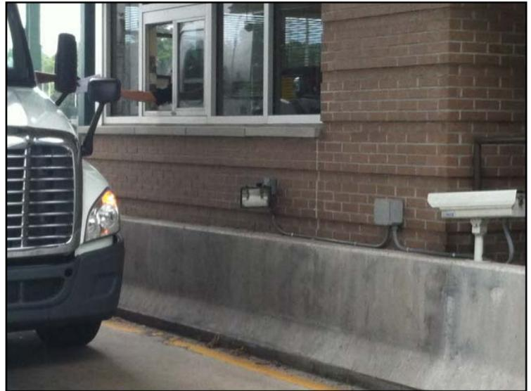
*Cameras for image capture of front license plate, side of truck, and cargo container number.*
