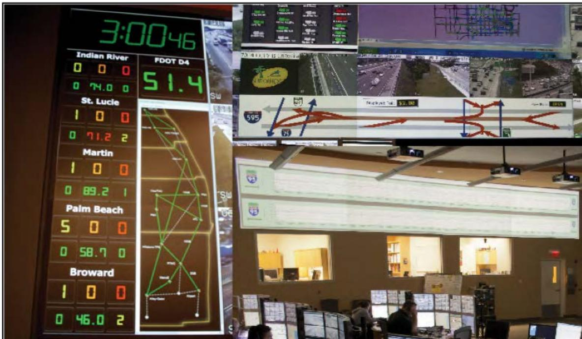
With the operator consoles on the bottom used for a personal video wall right on the desktop, the shared video wall can now be used as a status wall as show in the District Four image above. A few highlights include: the real-time, county-specific performance measures and roadside ITS network status shown on the left of the image, reversible lanes status shown on the upper-middle of the right, and the traffic speed profile shown on the lower-middle of the right.
