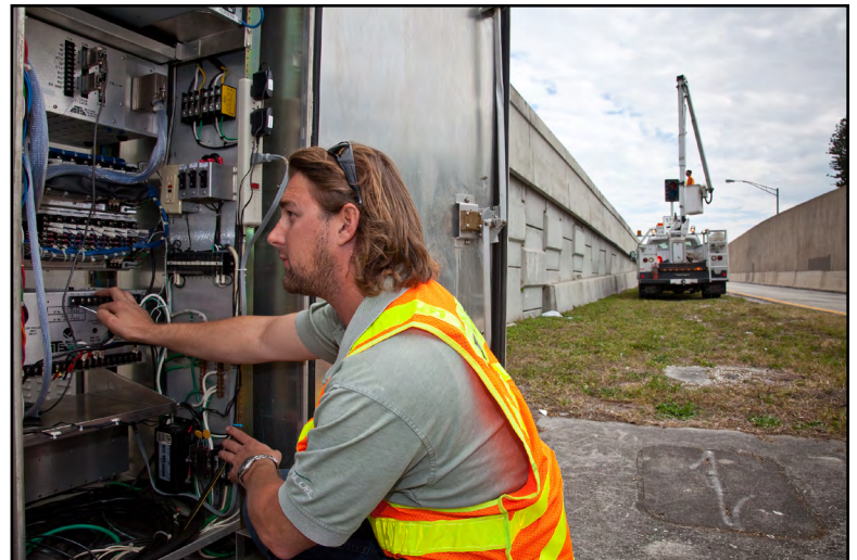
FDOT maintenance teams provide service to roadway equipment and technologies.
