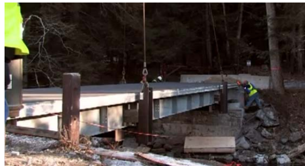
MassDOT Sapa R-Section Installation: Alan Road Bridge over Farmington River, MA
