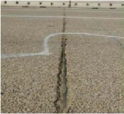
Reflective cracking and oozed material at FRP deck-to-deck joints
