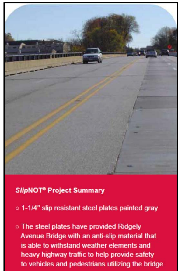
SlipNOT Road Plate on the Ridgely Avenue Bridge, Annapolis, MD
