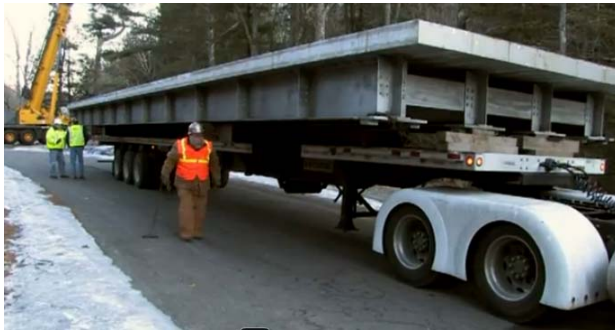
MassDOT Sapa R-Section Installation: Alan Road Bridge over Farmington River, MA
