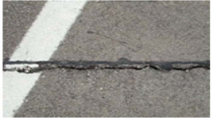
Reflective cracking and oozed material at FRP deck-to-deck joints
