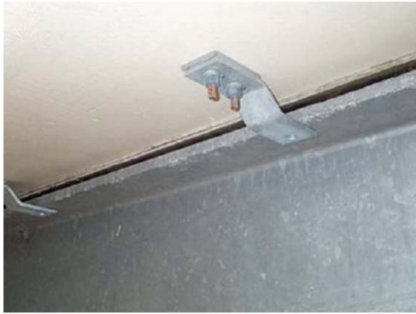
Clip Type Connection Separation
