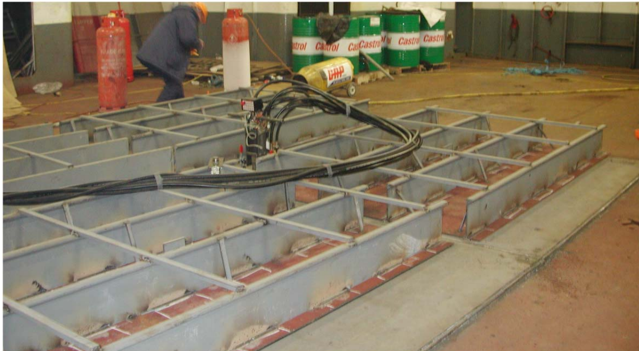
SPS Deck System Fabrication
