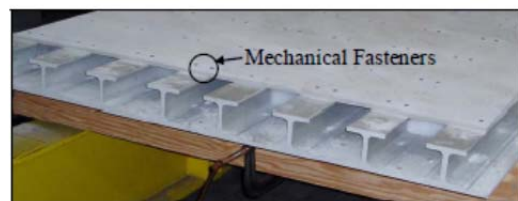
b) Picture of the deck showing all components
