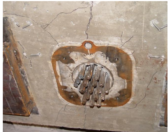
Figure 122. Photo of Radial Cracking of the specimen around the tube
