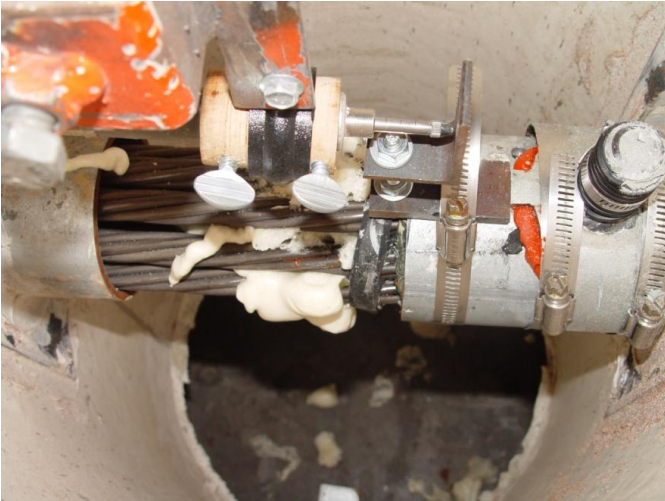
Figure 99. 12-strand - Third Specimen - Active Loading End – Post-active Loading Photo
