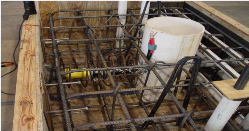
(d) Hollow section for shorter bond length - 2 nd and 3 rd 7 and 12 strand specimen Figure 10. First Set of Specimen Blocks Prior to Casting
