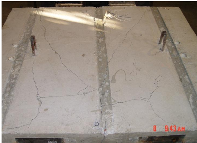
Figure 121. Photo of 19-Strand Specimen Block Cracking
