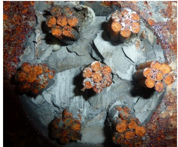
Figure 33. Crack Pattern Within Bearing Plate
