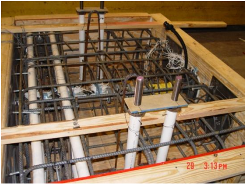
(c) DSI Bar and Tie-Down Piping
