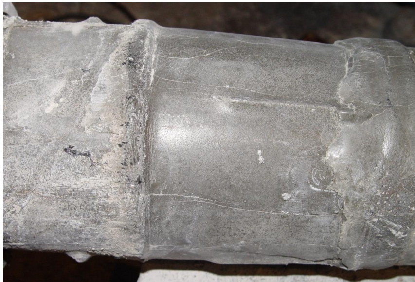
Figure 124. Grout as-found Under Removed Trumpet
