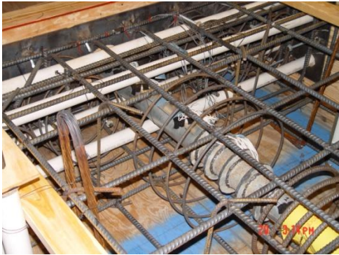
(b) Shear Flange Detailing
