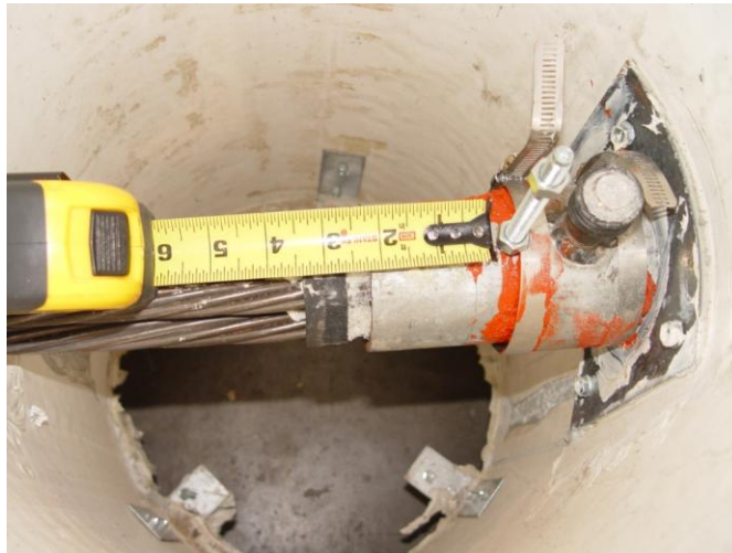
Figure 45. 7-strand - Second Specimen - Grout Slip Photo
