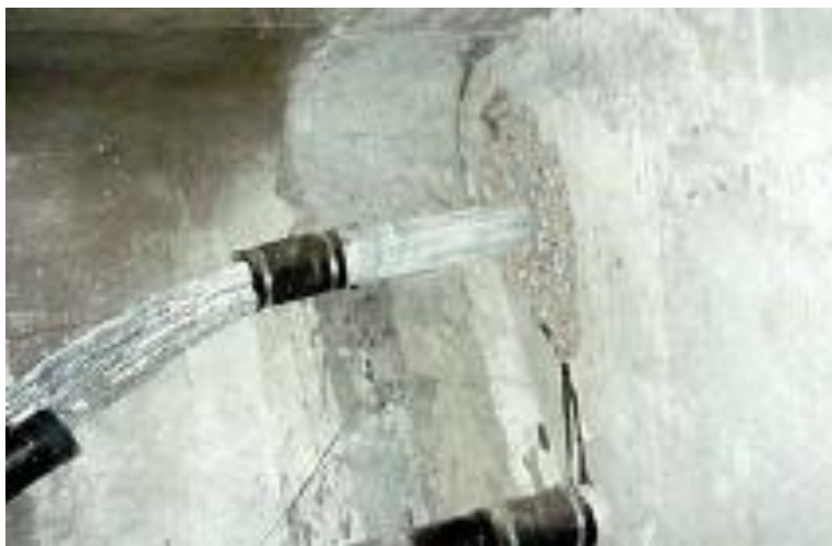
Figure 1. Mid-Bay Slipped Pipe
