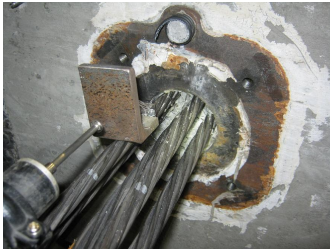
Figure 59. 7-strand – Third Specimen - Tendon Slip at Free face
