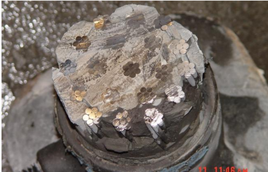
Figure 125. Cracking Located at the Removed Bearing Plate
