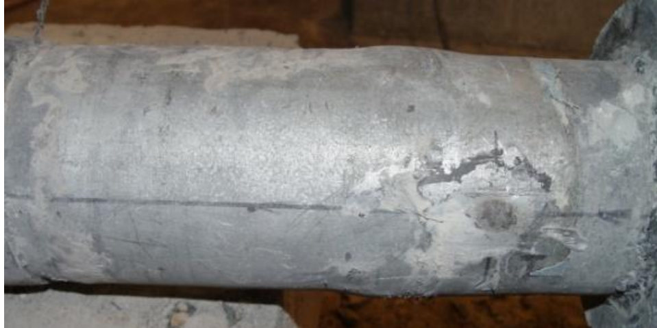
Figure 123. Deformed Location of 19-strand Pipe (R1/R6 location)
