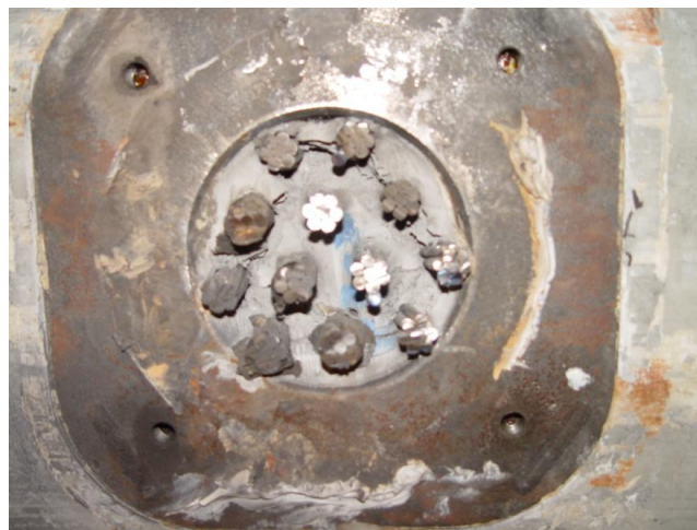
Figure 86. 12-strand - Second Specimen – Post-active Loading – De-stressing End Photo
