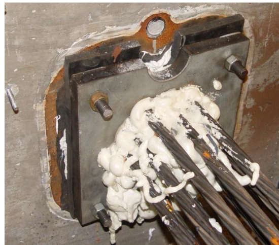
Figure 102. New Grout Block Device
