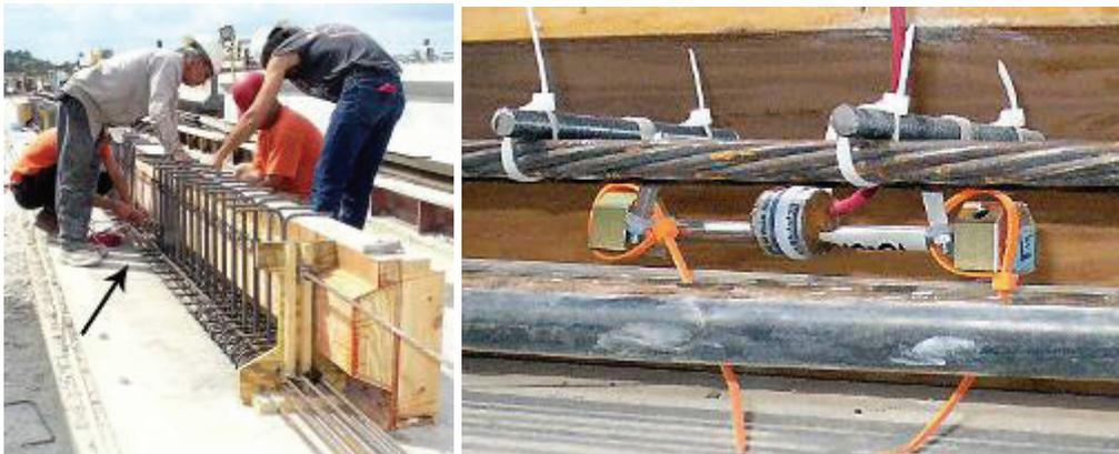
Figure 50. VWSG installation at midspan (arrow) of girder
