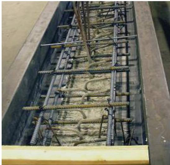
Figure 43. Bridge deck reinforcement prior to casting
