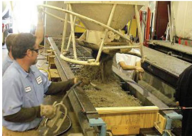
Figure 45. Deck concrete placement and vibration.
