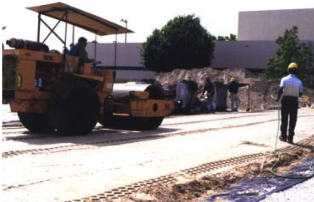
Figure 8.2 Compaction of the MSE wall
