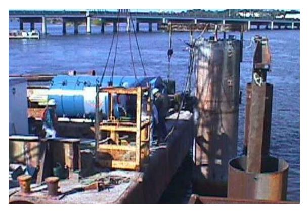
Figure 37, Lateral Statnamic Load Test
