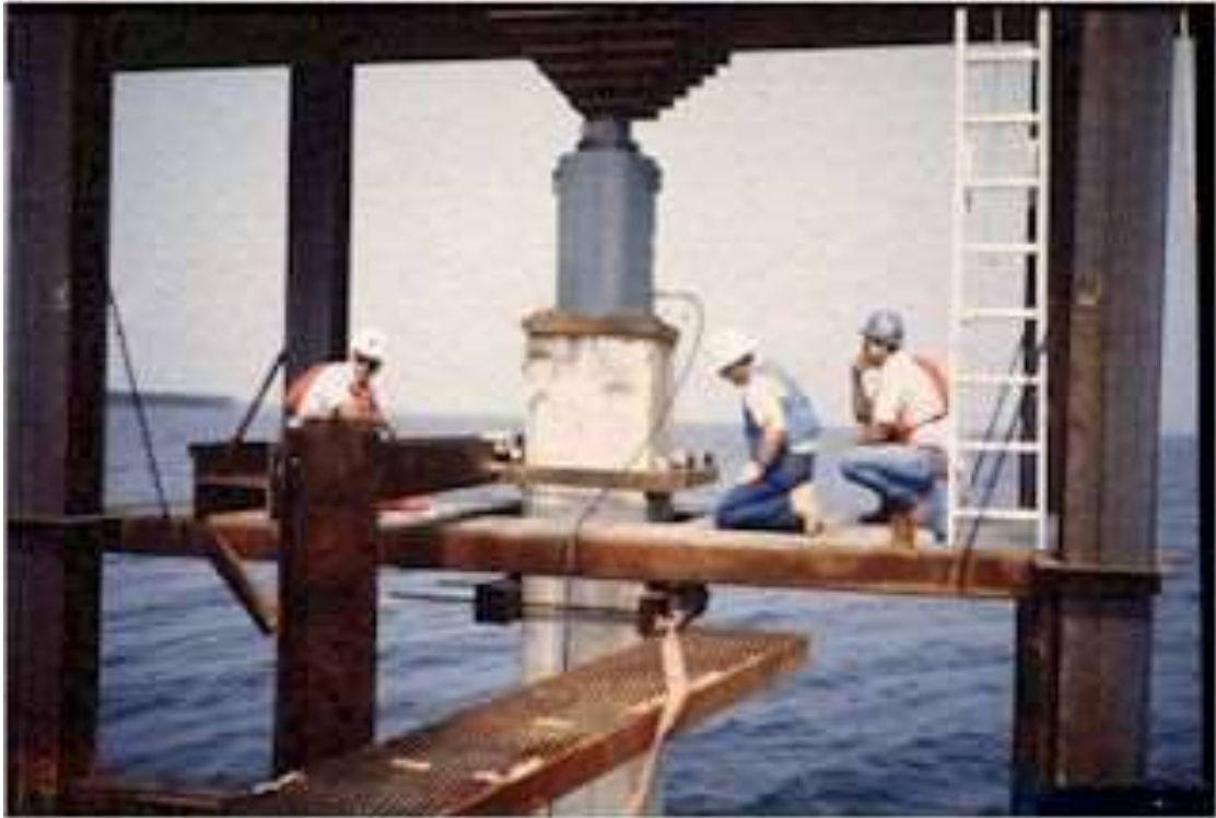
Figure 38, Static Load Test
