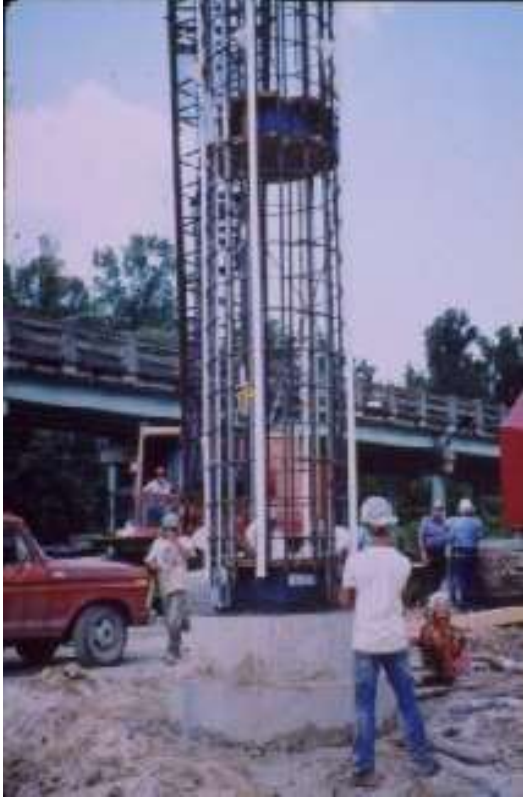
Figure 41, Osterberg Load Cells
