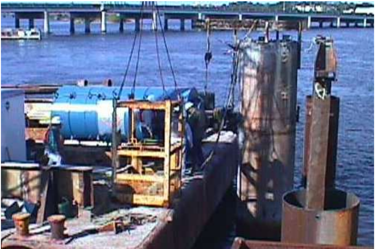
Figure 40, Lateral Statnamic Load Test
