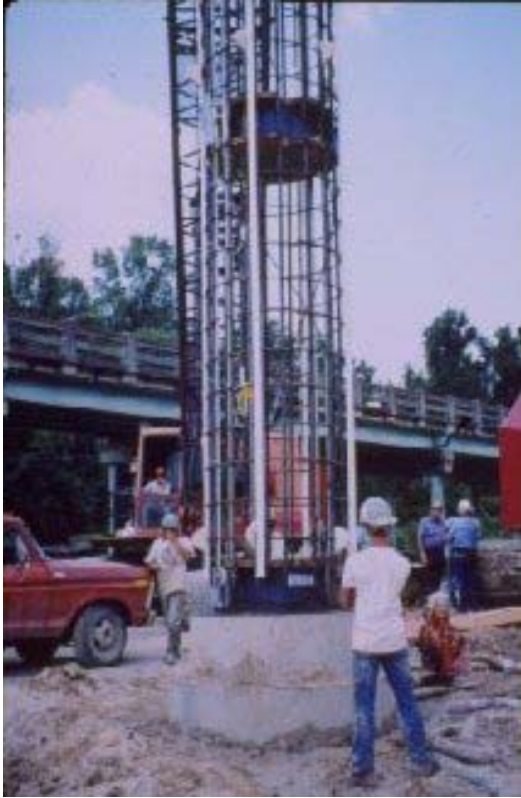
Figure 41, Osterberg Load Cells
