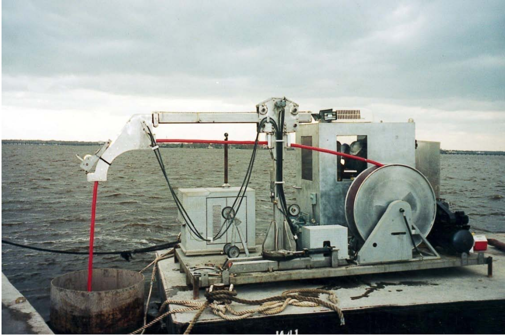
Figure 43, Shaft Inspection Device
