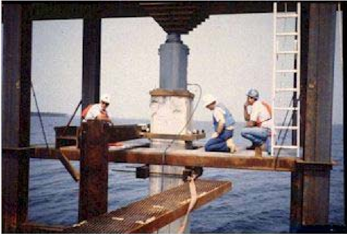
Figure 38, Static Load Test
