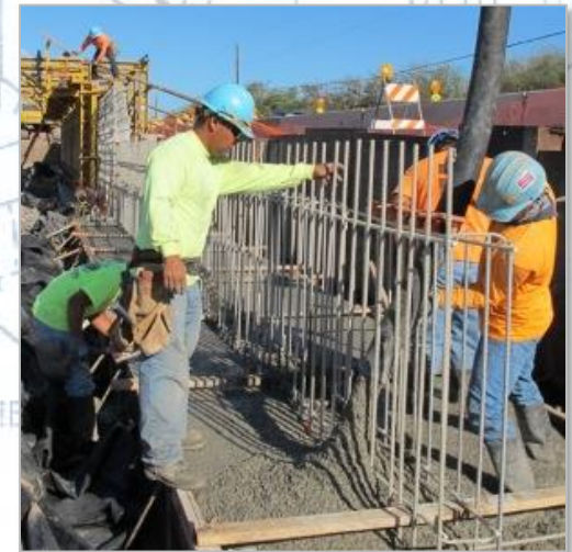
Photograph: GFRP Bars in retaining walls & railings (Hughes Bros.)
