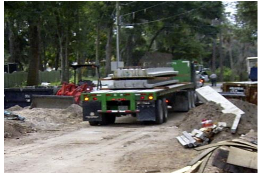
PRESTRESSED SLAB BEAMS Gospel Island, Florida (2 – 39 ft. beams @ 25 kips = 50 kips total)
