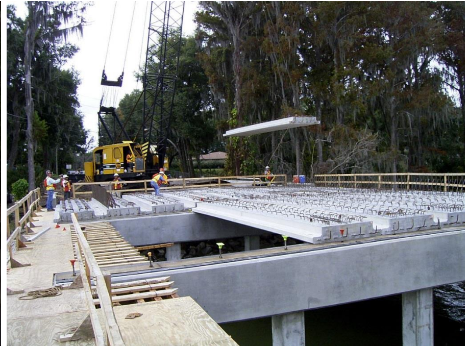
PRESTRESSED SLAB BEAMS
