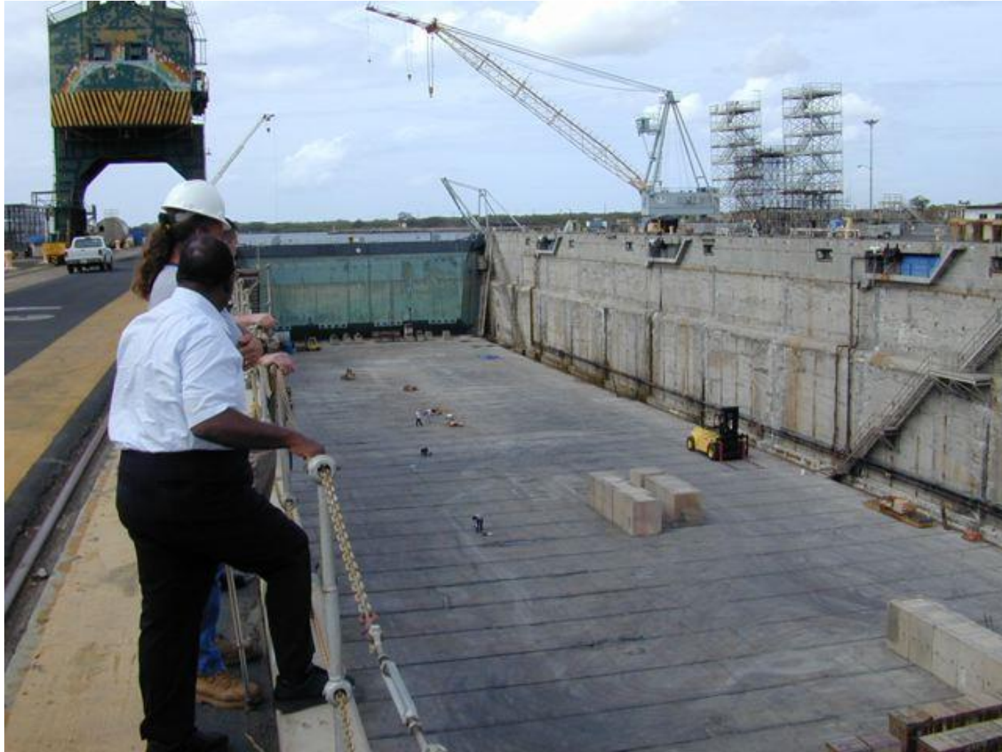
Dry Dock rehabilitation Pearl Harbor
