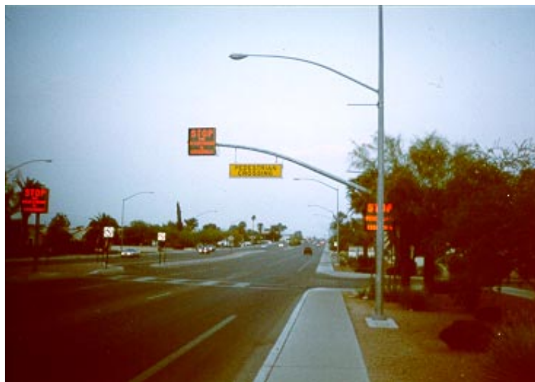
Figure 3. Pedestrian-activated overhead sign in Tucson, Arizona
