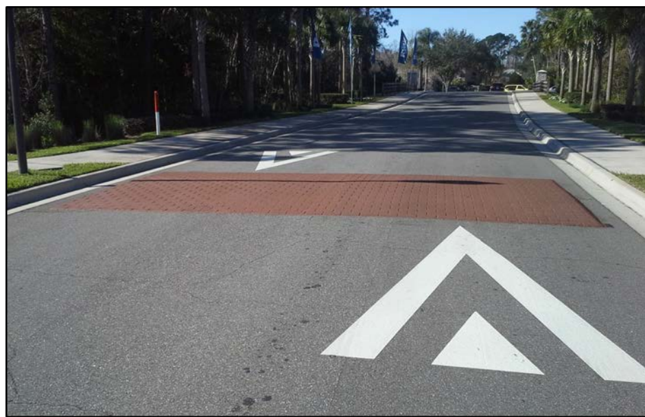
Inside Loop Road, Orange County, Florida
