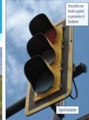
and local road agencies have adopted this treatment as a human blind drivers. The magnitude of the CMF Clearinghouse is a 15% reduction
