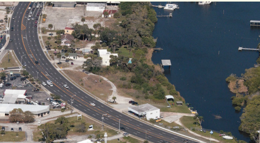
District 5: Ranger Construction Industries for their project on State Road 5 Melbourne from South of State Road 500/192 to North of State Road 518 in Brevard County.
