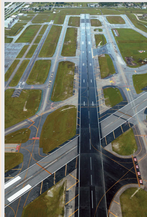
Special Projects Award goes to Community Asphalt for their Palm Beach International Airport Runway 10L-28R in Palm Beach County.
