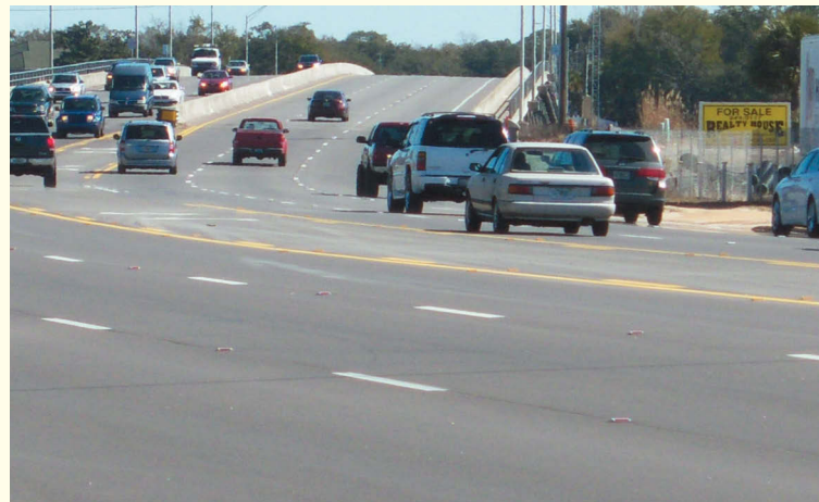
District 3: Midsouth Paving Inc. for their project on Hwy 85: from State Road 30 (US98) to a point North of Richburg Avenue in Okaloosa County.
