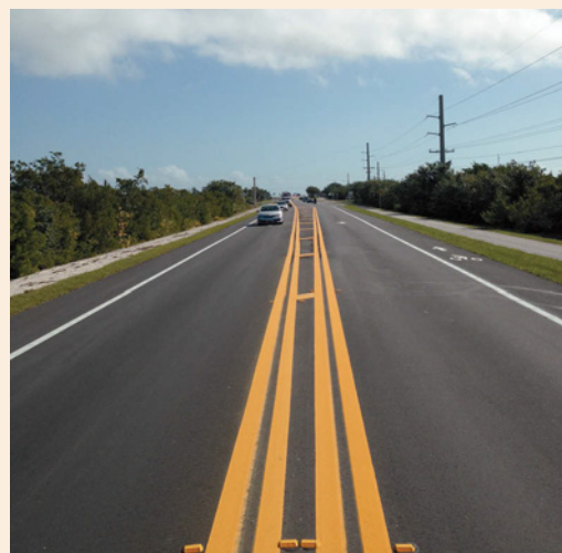
District 6: General Asphalt Co., Inc. for their project on State Road 5/Overseas Highway from West Indies (MM 27.4) to West of Ships Way (MM 29.5) in Monroe County.
