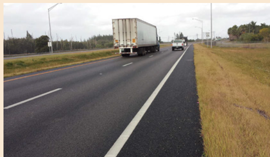
District 6: Community Asphalt Corp for their project on State Road-25 (Okeechobee Road); From a point west of Northwest 118th Avenue to the Miami-Dade County Line in Miami-Dade County.
