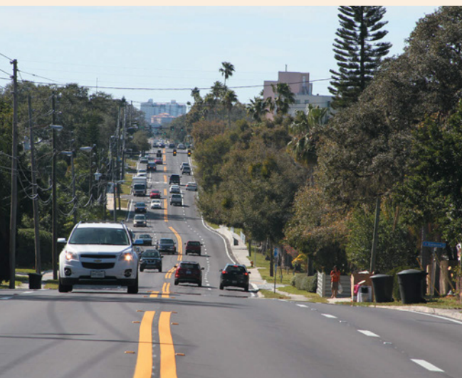
District 7: The Lane Construction Corp. for their project on State Road 590 (Drew St.) from Myrtle Avenue to Mariva Avenue in Clearwater in Pinellas County.
