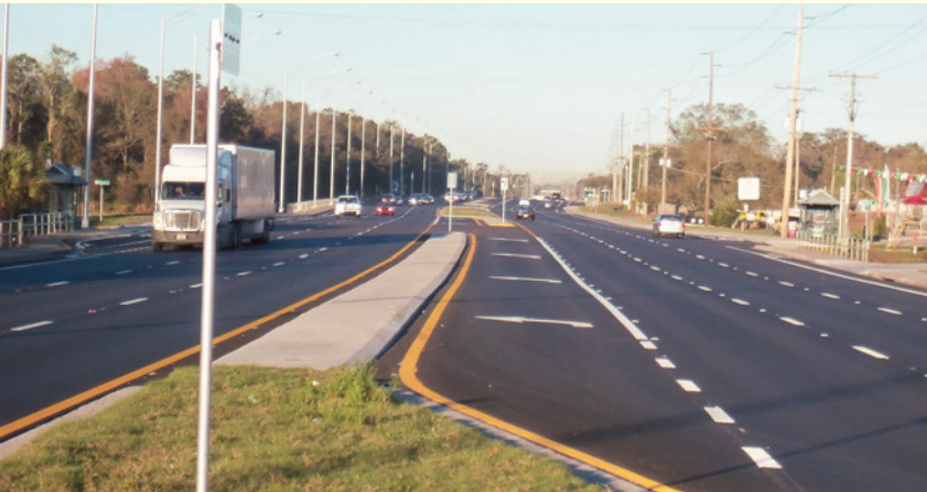
District 7: Ajax Paving Industries of Florida, LLC for their project on Martin Luther King Blvd. (State Road 574) from I-4 to Laura Street in Hillsborough County.
