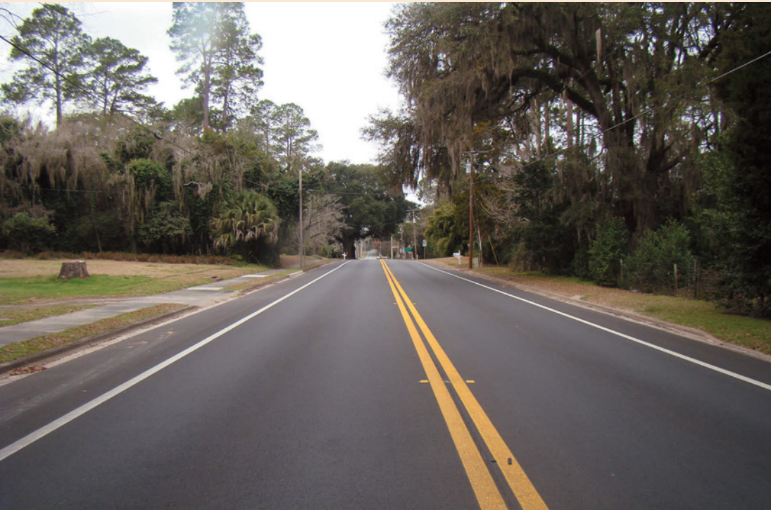
STATEWIDE & District 3: Anderson Columbia Company for their project on State Road 69 from North of State Road 10 (US 90) to State Road 71 (Bryan Street) in Jackson County.
