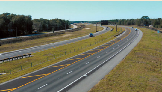
District 8: D.A.B. Constructors, Inc. for their project on Suncoast Parkway from M.P. 28.678 to 37.415 in Pasco County.
