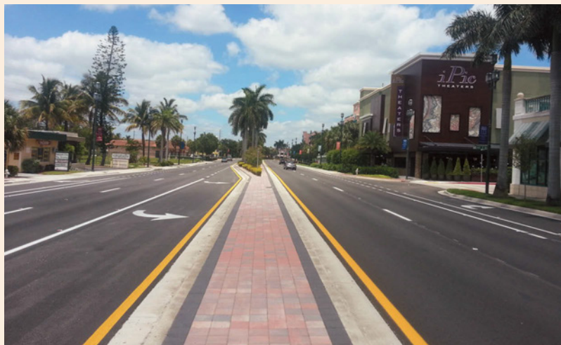
District 4: Ranger Construction Industries for their project on State Road 5 (US-1) from Camino Real Road to North of Glades Road in Palm Beach County.
