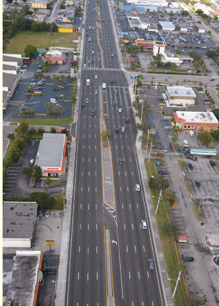
STATEWIDE & District 4: Ranger Construction Industries for their project on State Road 704/Okeechobee Boulevard from Military Trail to State Road 9/I-95 in Palm Beach County.
