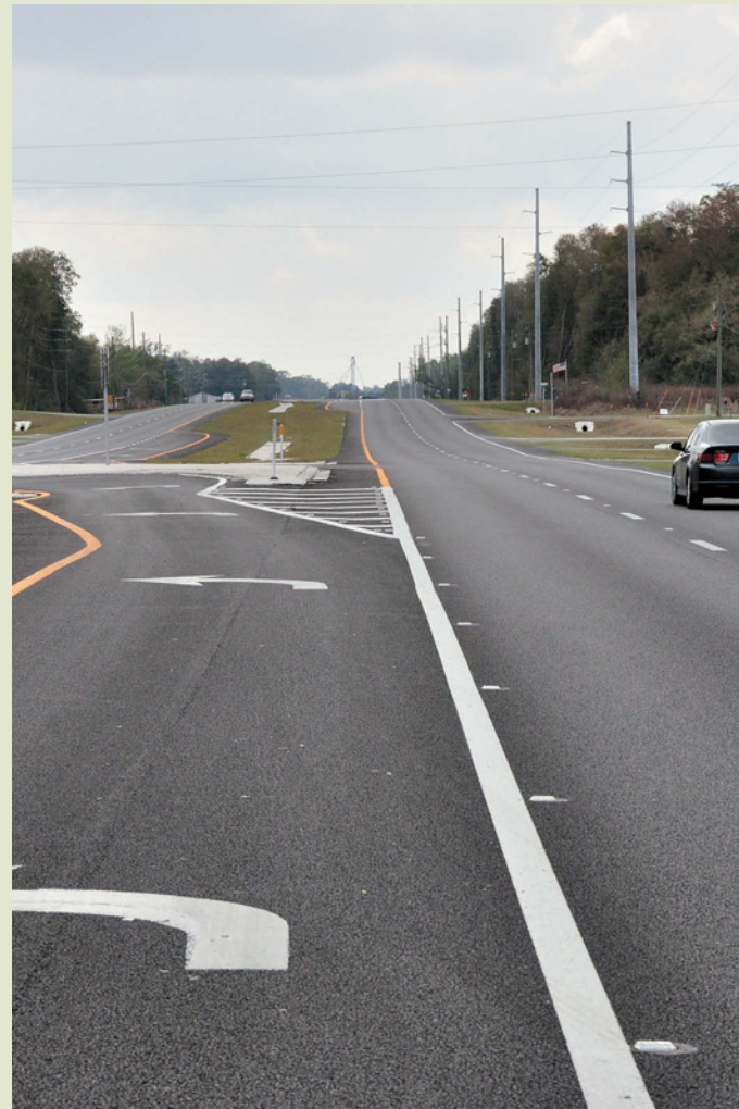
District 5: DAB Constructors, Inc. , for their project on SR 35 from the Sumter County Line to CR 42 in Marion County.
