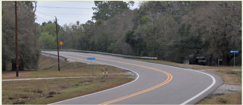
District 2: Hubbard Construction Company for their project beginning at the Duval/Nassau County Line on SR 200 and goes 14.692 miles in Nassau County.
