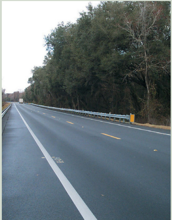
District 2: Anderson Columbia Co., Inc. , for their project on SR 100 from the Clay County Line to CR 309 in Putnam County.
