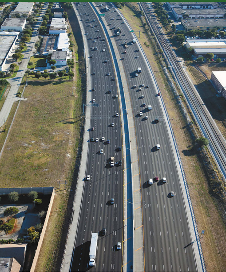
STATEWIDE and District 4: Community Asphalt Corporation for their project on SR 9 (I-95) North Bound from South of Linton Blvd. to South of Boynton Beach Blvd. in Palm Beach County.
