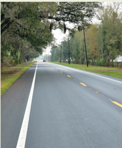
District 5: DAB Constructors, Inc. , for their project on SR 35 from Hernando County line to Main Street and from Main Street to SE 13th Ave. in Sumter County.
