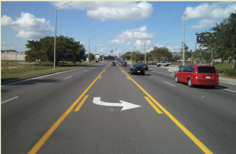
District 1: APAC-Southeast, Inc. , for their project on SR 555 (US 17) from South of Cypress Gardens Blvd. to South of Havendale Blvd. in Polk County.
