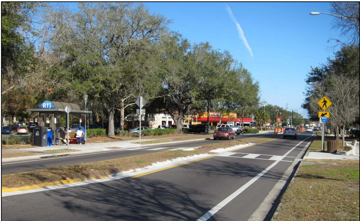
North Main Street, Gainesville, FL
