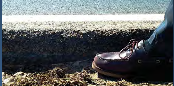
Sharp, steep pavement edge drop-offs can contribute to crashes.
