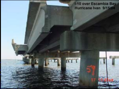
Misaligned Spans: 50 EB & 16 WB
