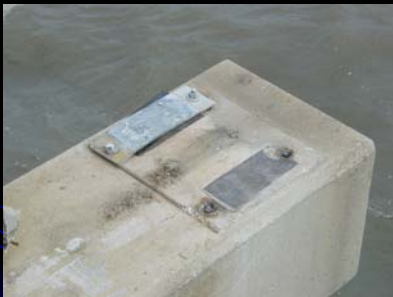
Hold-Down Bolts & Embedded Studs Sheared
