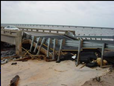
East Abutment of WB Bridge
