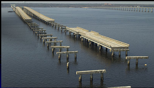
60' Trestle Spans Missing: 46 EB & 12 WB
