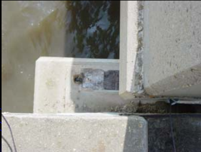
Hold-Down Bolts Sheared
