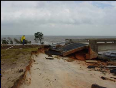
East Abutment of EB Bridge
