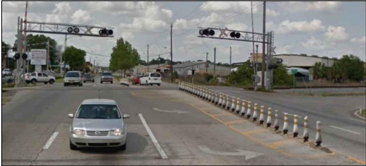
Alexander Street, SR 39A, Plant City, FL 1
