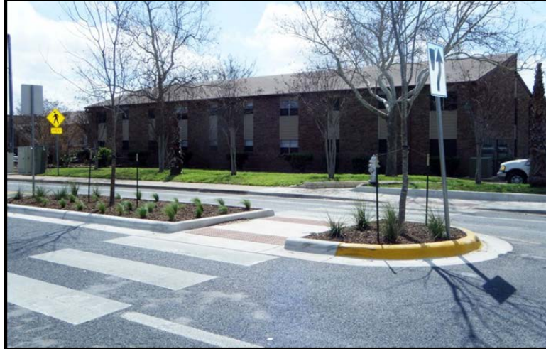
Figure 8 – 56 Pedestrian Median Refuge with Curb Extension
