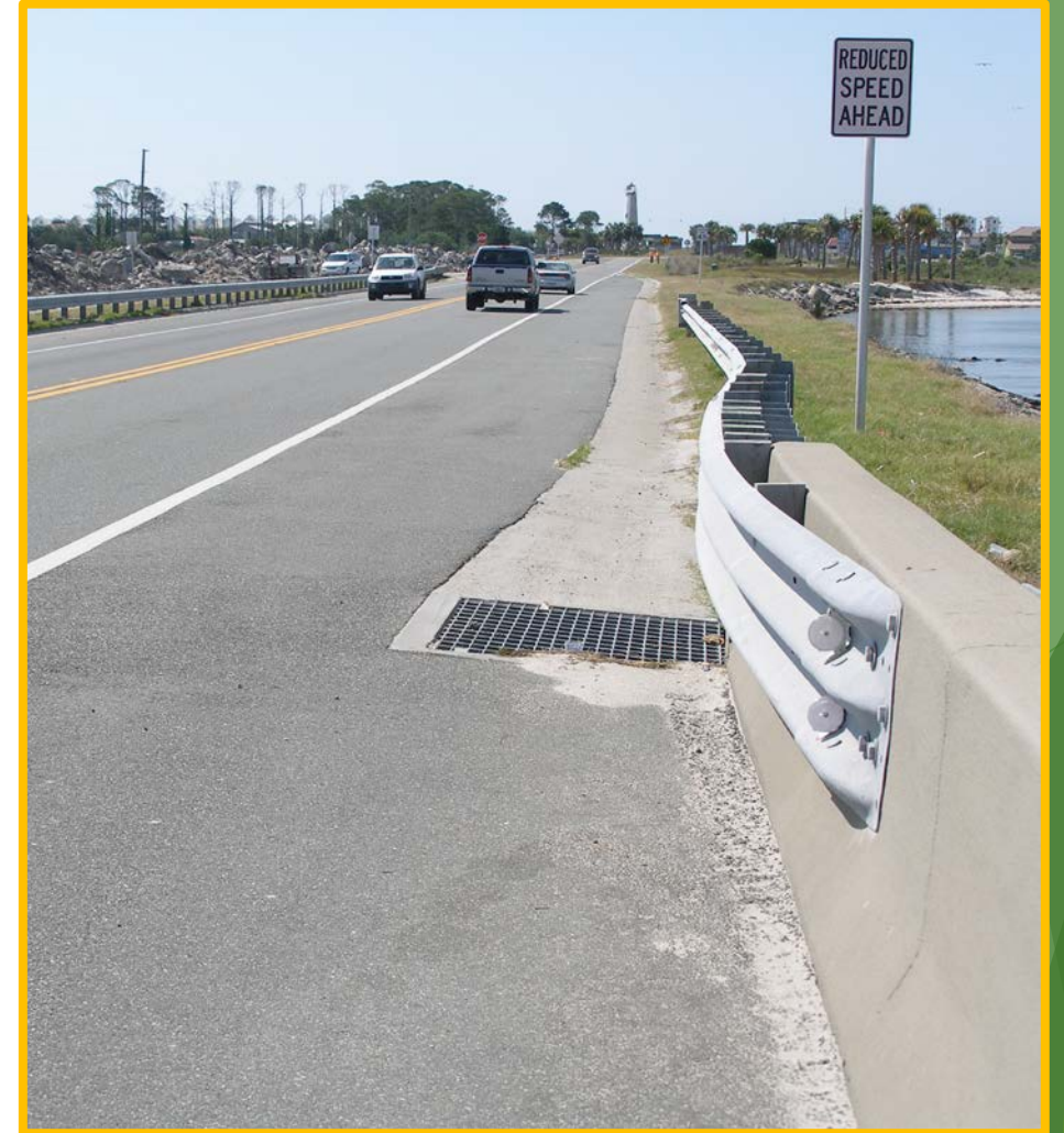
SR 309, St. George Island Bridge, FL
