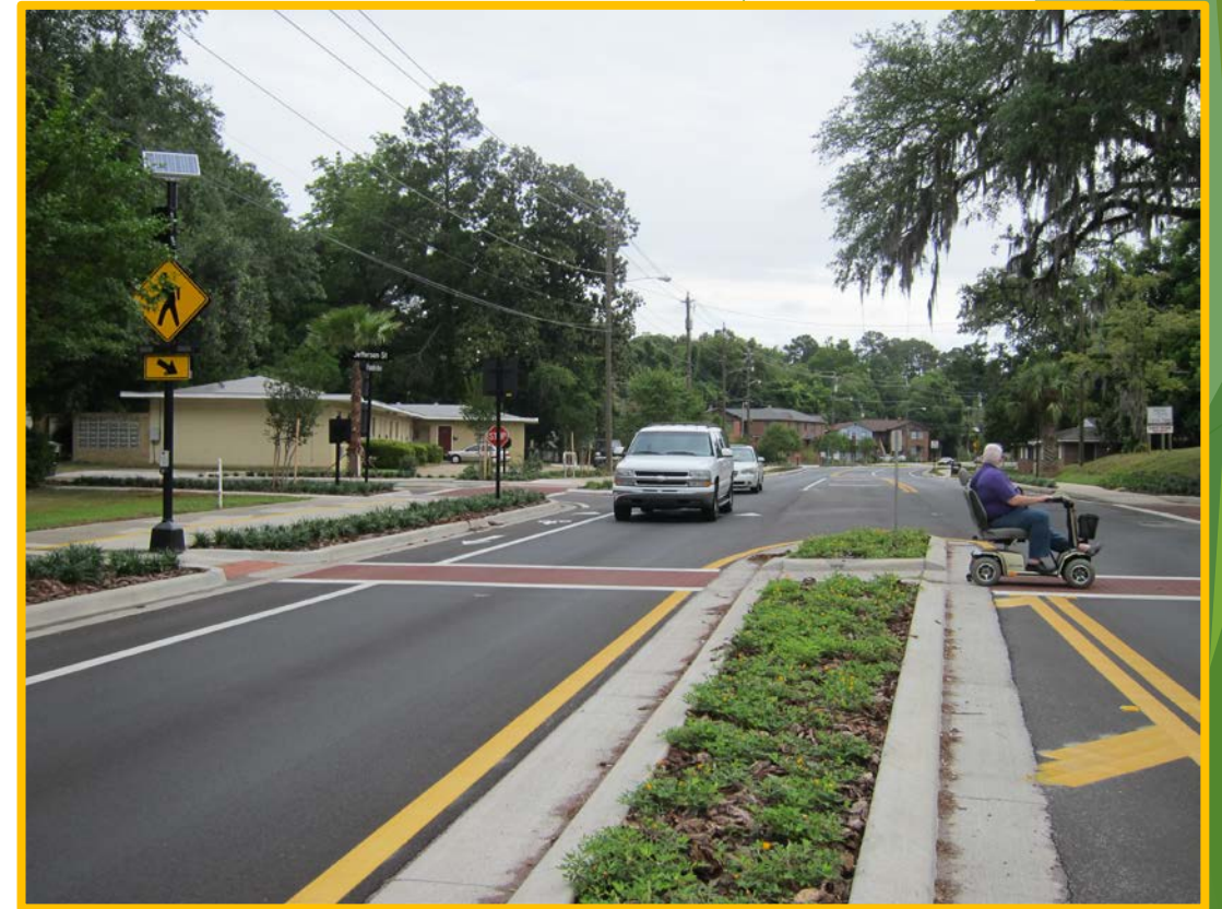
Franklin Blvd, Tallahassee, FL
