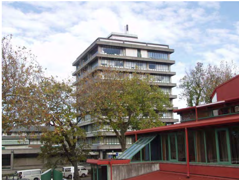
Figure 1 University of Auckland Engineering Building where the Hydraulics Laboratory and the flume used for the live bed scour experiments are located.
