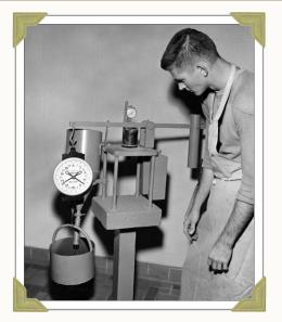
**1955:** An unidentified man performs the Florida Bearing Value test in the Bearing Value and Compaction room at the SRD Testing Laboratory in Gainesville. *Source: Florida Memory*
