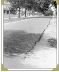
**1917:** A county-built sand-asphalt road near Mount Dora showing typical wear patterns and ragged shoulders. *Source: Florida Memory*
