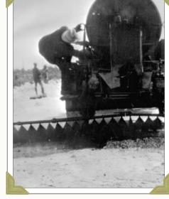
**1917:** Asphaltic oil is sprayed on a prepared roadbed to create a sand-asphalt road. *Source: Florida Memory*
