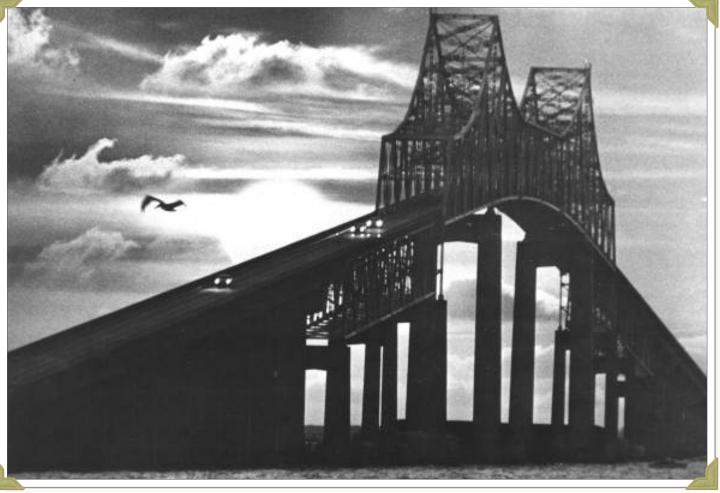
1963: The original Sunshine Skyway, spanning Lower Tampa Bay from St. Petersburg to Manatee County, showcased the use of prestressed concrete and spurred designers and engineers to refine and enhance prestressed concrete for structural applications. Source: Florida Memory
