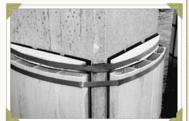
Approx. 1987: Conductive rubber was developed by FDOT and first used in 1987 on the piles of a bridge carrying US-90 in Jacksonville. Source: NCHRP Synthesis 398
