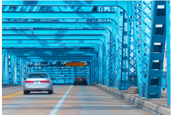
The Main Street Bridge in Jacksonville, Florida, over the St. Johns River, is a steel girder bridge.
