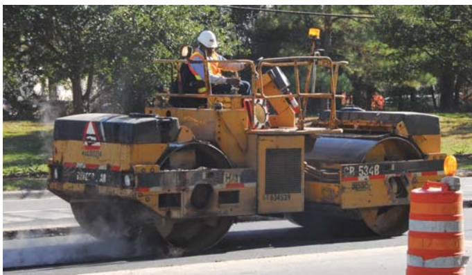
A vibratory roller compacts fresh asphalt.
