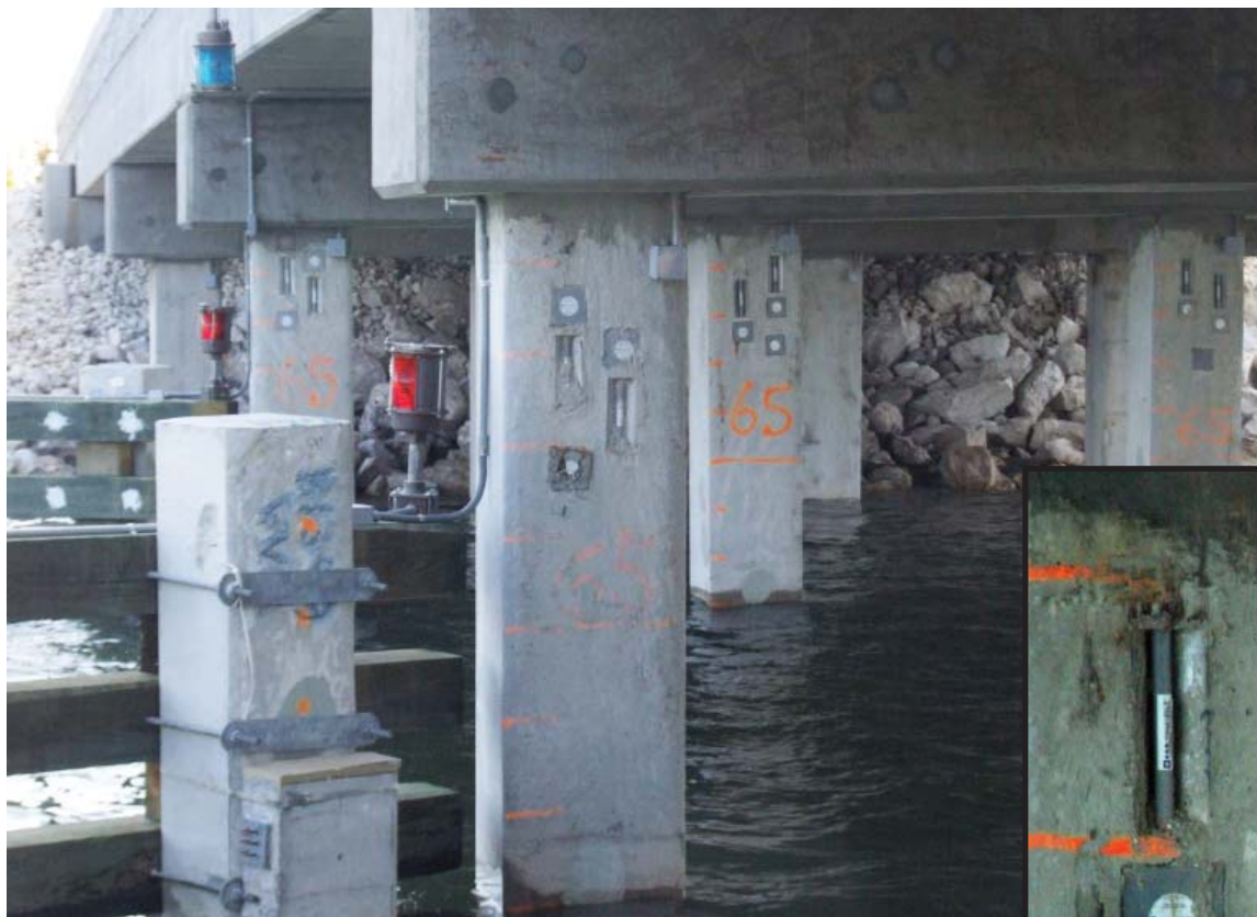
Above: Embedded data collectors, sensor battery packs, and electrical connection boxes are visible on piles and durability segments attached to fender piles of the Key Royale Bridge.
