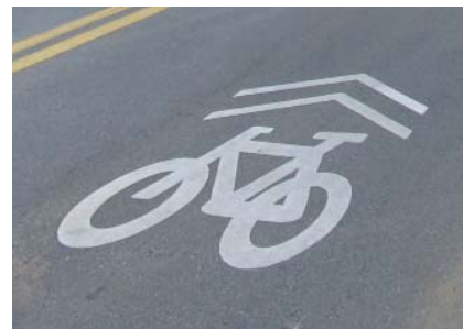
Sharrows are markings placed on roadways to indicate that bicycles share the lane with automobiles.
