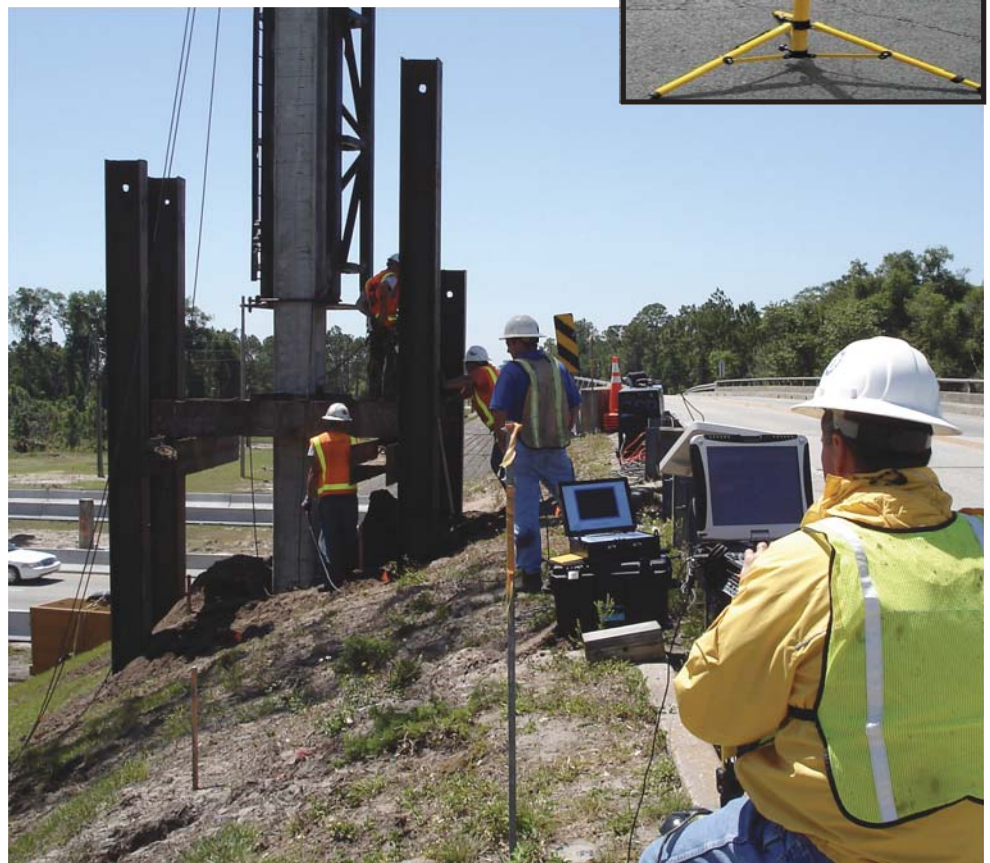
Bottom photo: Field engineers monitor pile driving characteristics at a construction site.
