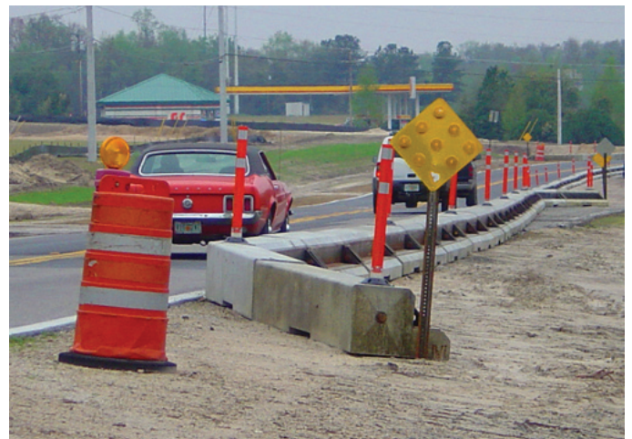
Sloping ends will soon replace blunt barrier ends.
