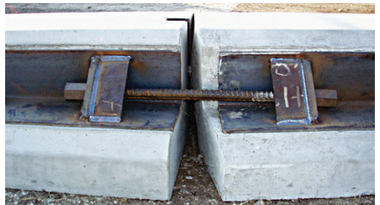
The linkage between barrier segments.
