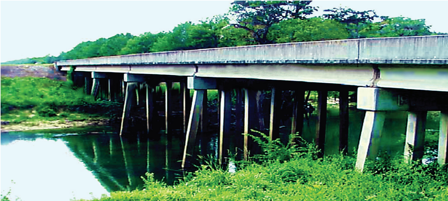
The foundation piers of the I-10 Chipola River bridge are sited in limerock. Core rock samples from the bridge site were used for the first test of the Rotating Erosion Test Apparatus (RETA).
