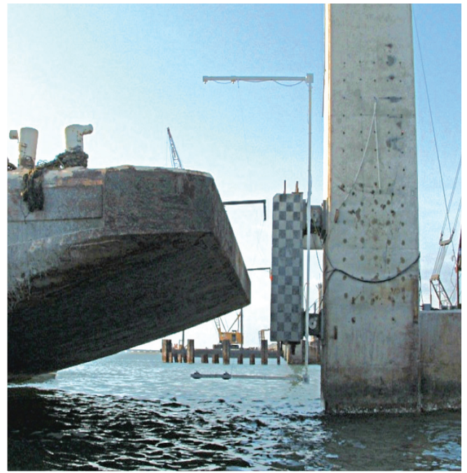
Above and left: The barge approaches the bridge piling.
