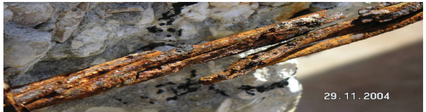
Corrosion on interior steel strands.
