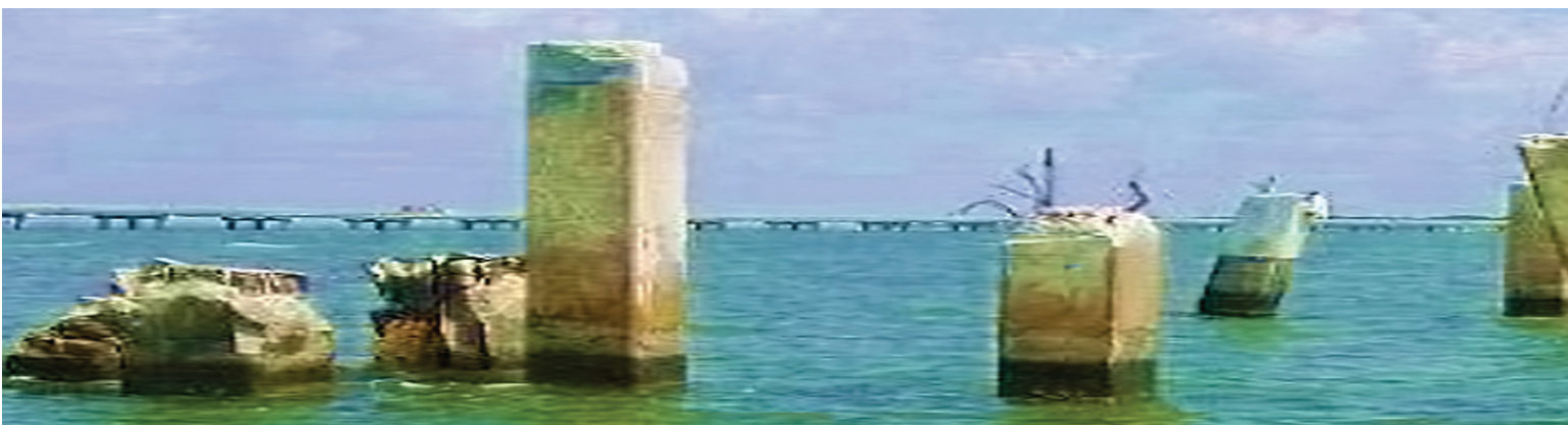
Corroded pilings at the St. George Island Bridge.
