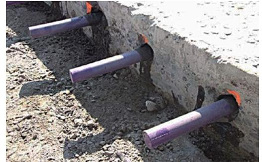
*Dowel bars, studied in this project, are set in one slab of pavement waiting for the next one to be poured.*
