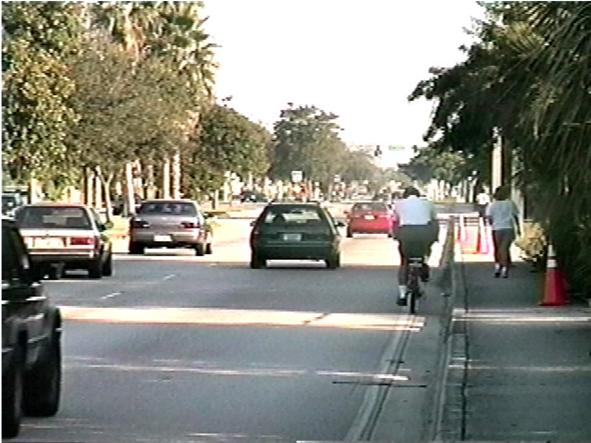
Figure 1. Before condition with 14-foot wide curb lane.
