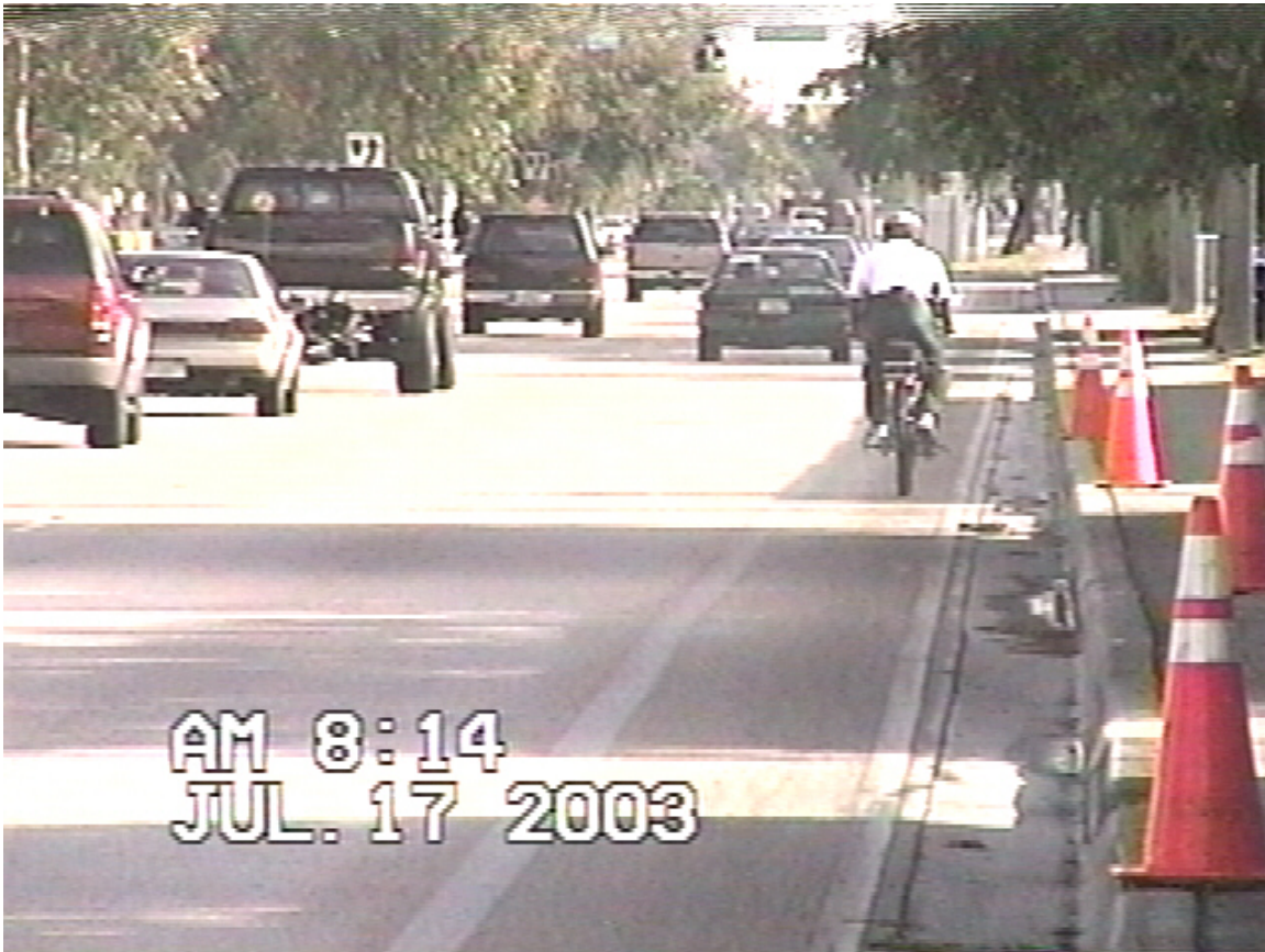
Figure 2. After condition with 11-foot travel lane and 3-foot undesignated lane.
