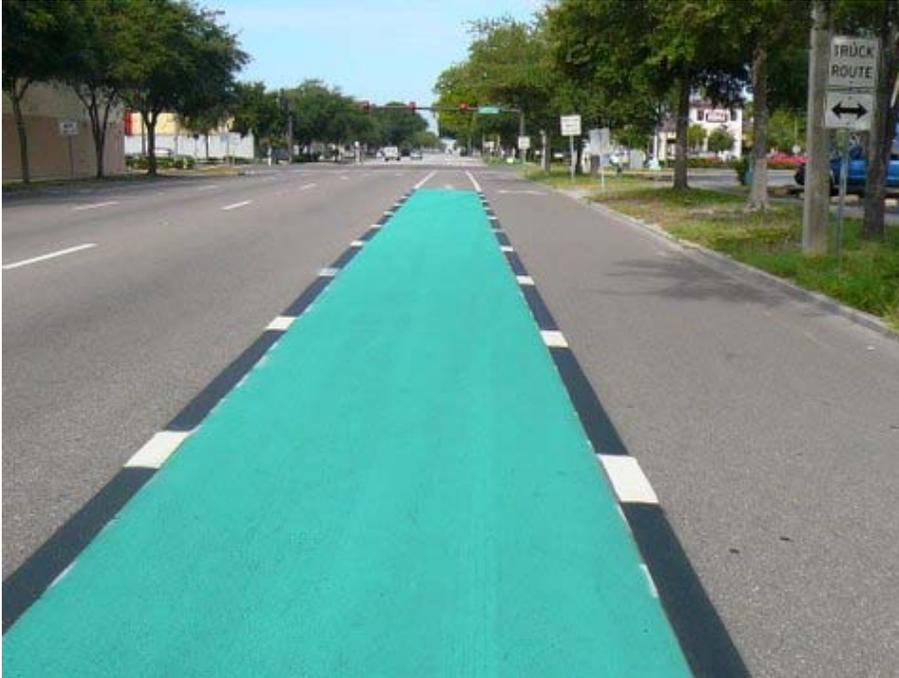
**Figure 4. Black mini-stripes added to border of green bike lane weaving area.**
