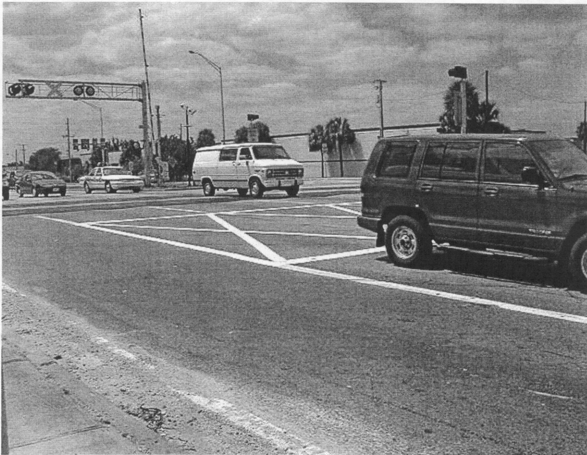
Figure 2-2. Commercial Blvd. Crossing with European X Markings Installed
