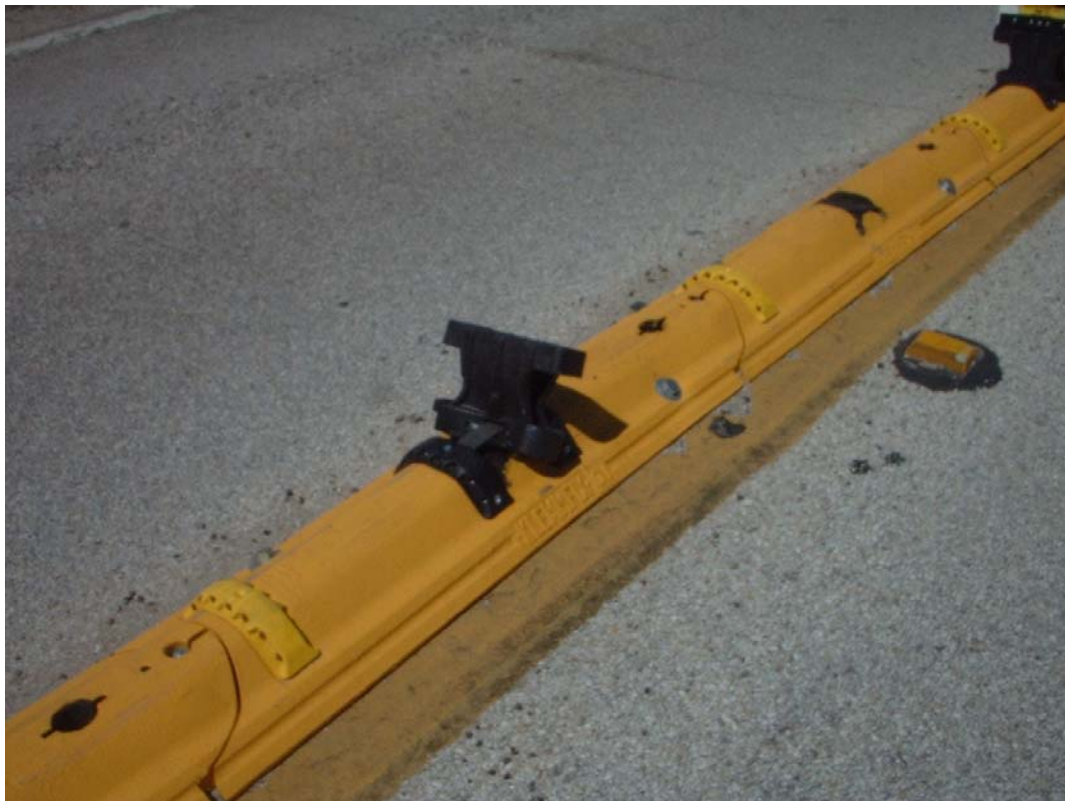
Figure 4-1: QWICK KURB® Damage
