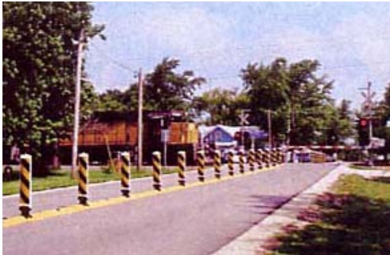
Figure 2-1: QWICK KURB® Crossing
