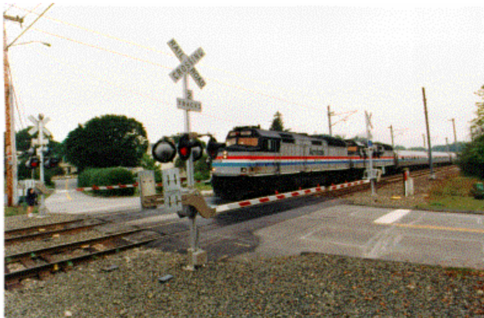
Figure 2-7: Four-Quadrant Gate with Automatic Train Stop
