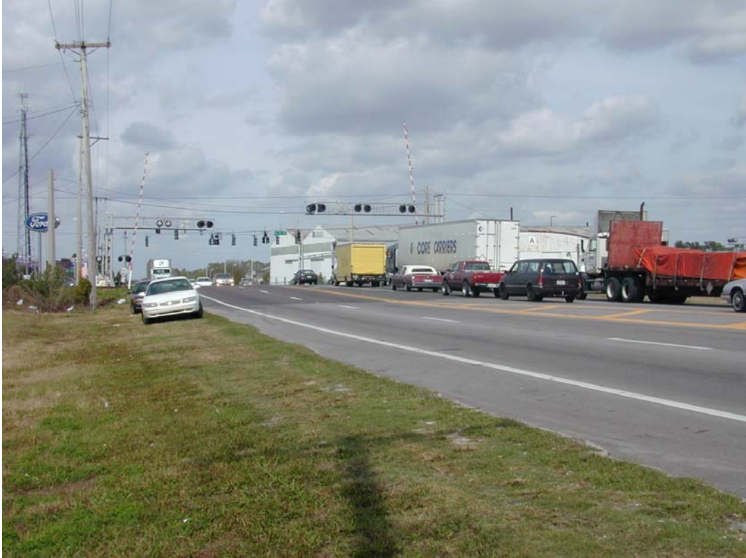
Figure 3-3: Park Road Site from the South (Before Separator Installation)
