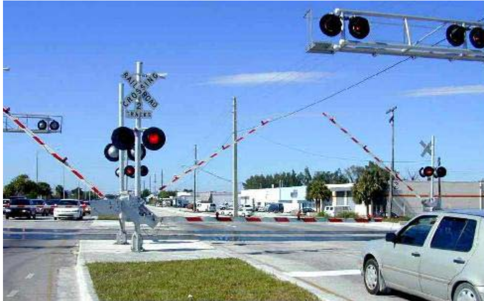
Figure 2-2: Four-Quadrant Gate Railroad Crossing
