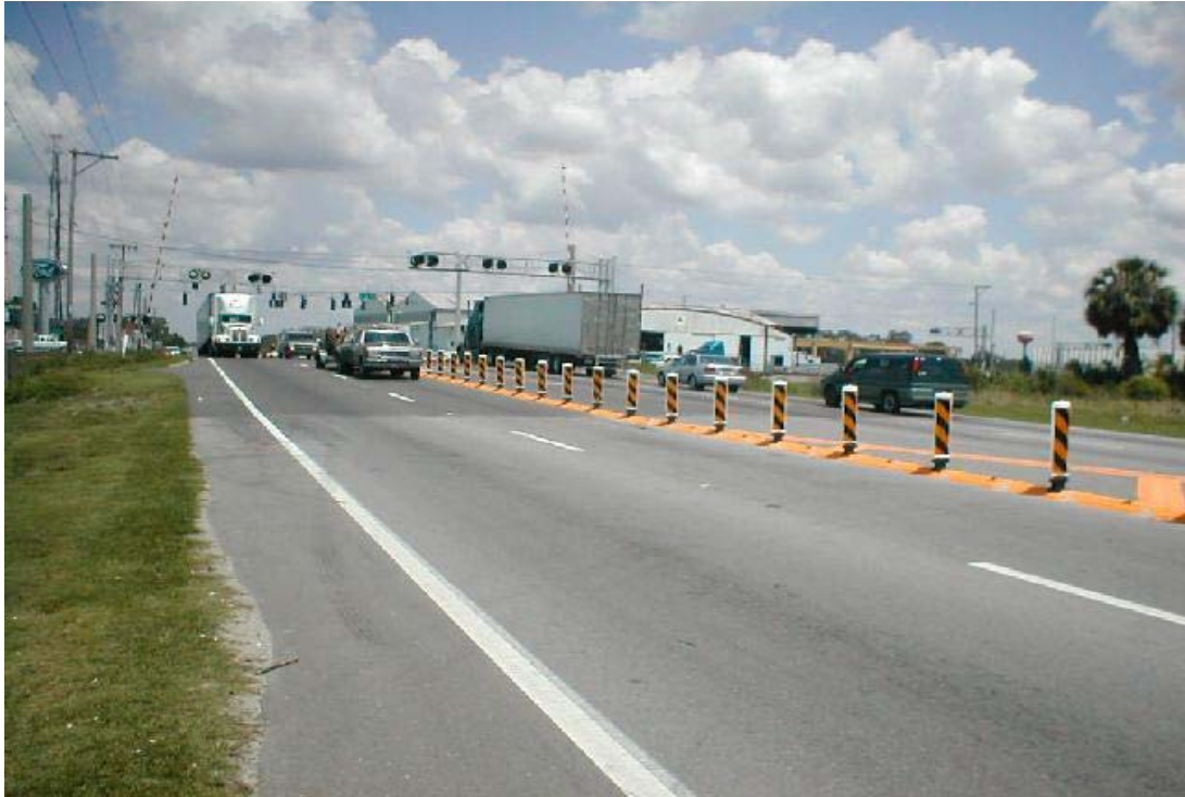
Figure 3-4: Park Road Site from the South (After Separator Installation)
