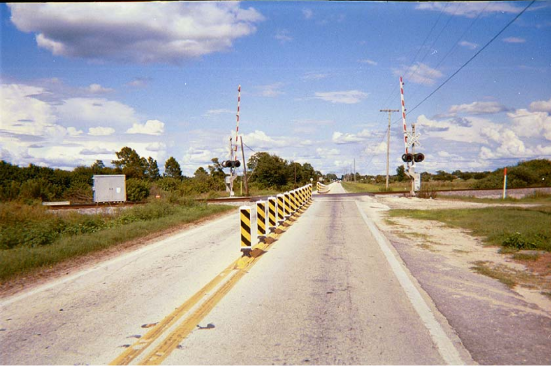
Figure 3-10: US-98 Site from the West (After Separator Installation)
