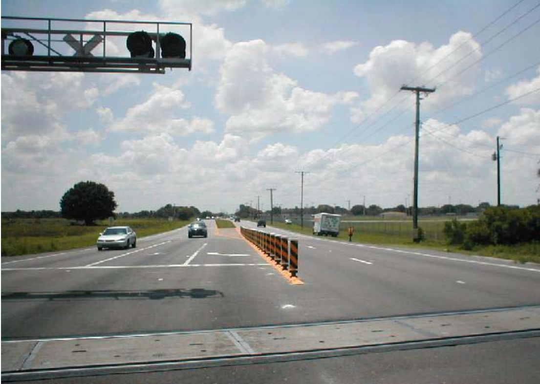
Figure 3-5: Park Road Site from the North (After Separator Installation)
