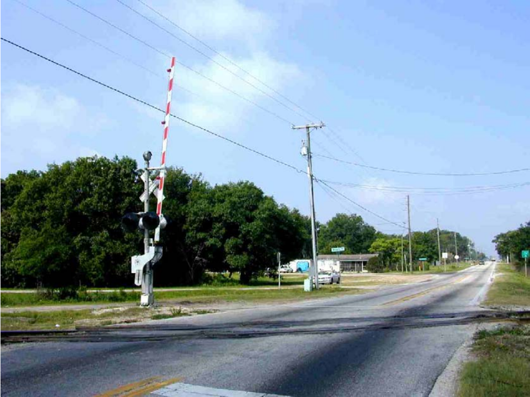
Figure 3-9: US-98 Site from the East (Before Separator Installation)
