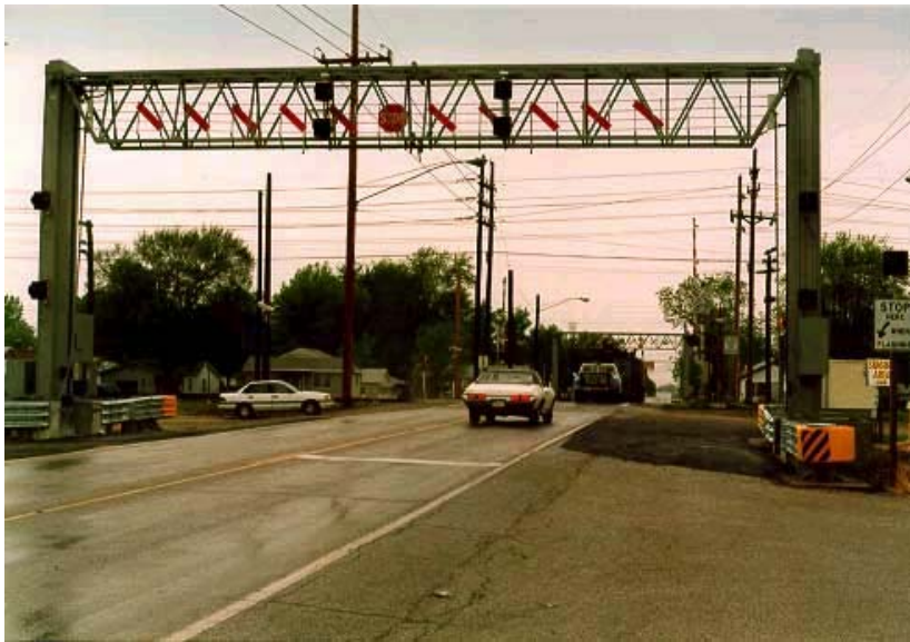
Figure 2-3: Vehicle Arresting Barrier at Railroad Crossing
